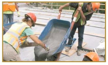
Batch size and mixing performance are factors in the outcome of these blends and were analyzed to determine recommended procedures for the most robust mix design. Recent test mixes developed at Montana State University demonstrated compressive strengths of approximately 20 ksi with flows of 8-11 inches. The mixes were also tested for tensile strength, elastic modulus, and shrinkage.
