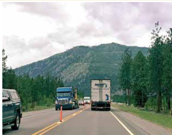
Example of crossover traffic on I-90.
