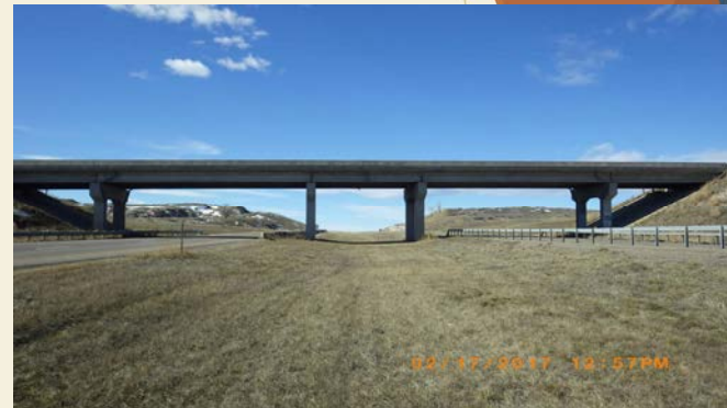
Image of Colstrip Interchange Bridge
