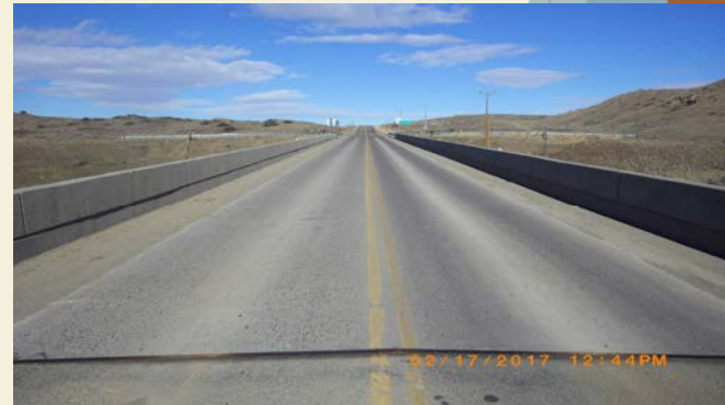
Image of Deck of Colstrip Interchange Bridge
