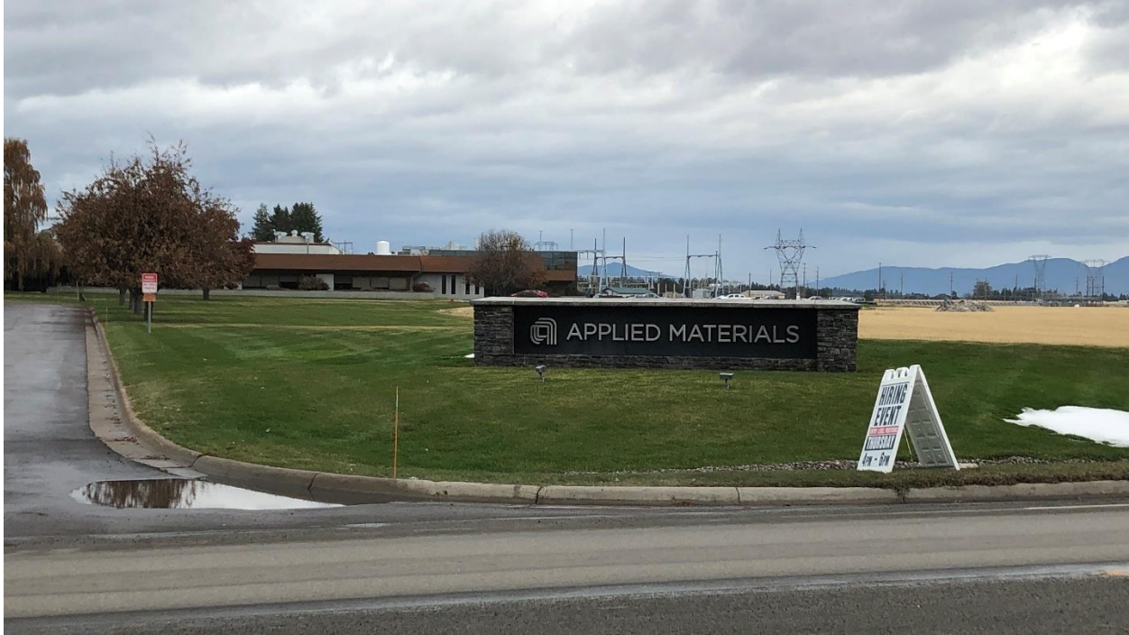
The Applied Materials facility, located North of W. Reserve Dr., is a large quantity hazardous waste generator.
