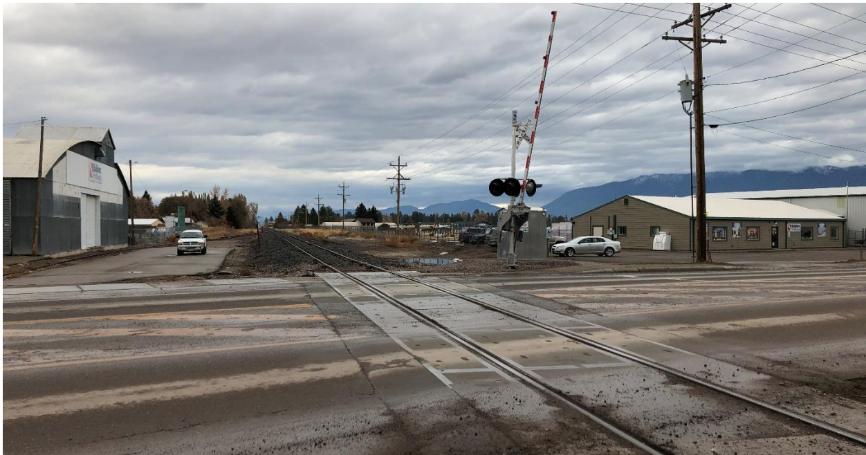
The Montana Rail Link crossing was recently updated with new pedestrian-friendly improvements.
