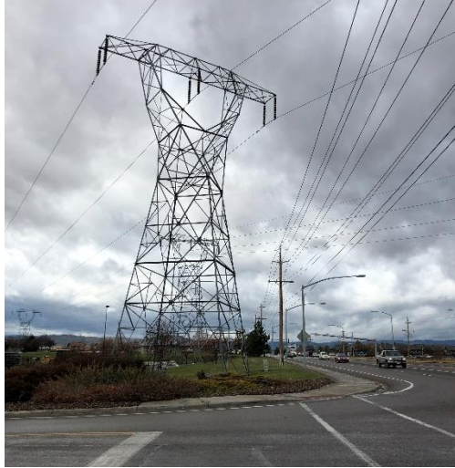
Utilities are present within the corridor, like these major power transmission towers.
