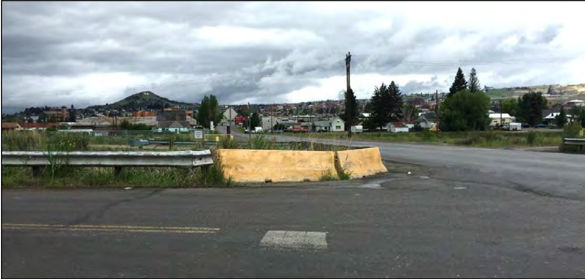
Photograph 1. Barricades on the northwest corner and the skewed approach angles of the Kaw and George intersection may be contributing to a crash trend.
