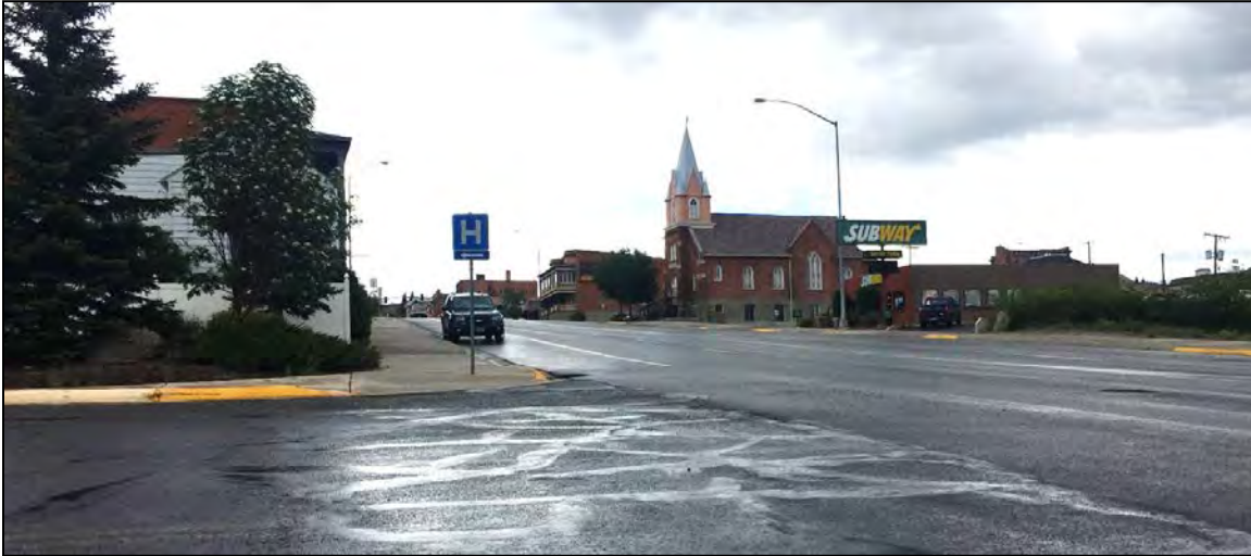
Photograph 4. Grade changes on Montana Street may be contributing to a crash trend at the intersection of Montana Street and Porphyry Street.
