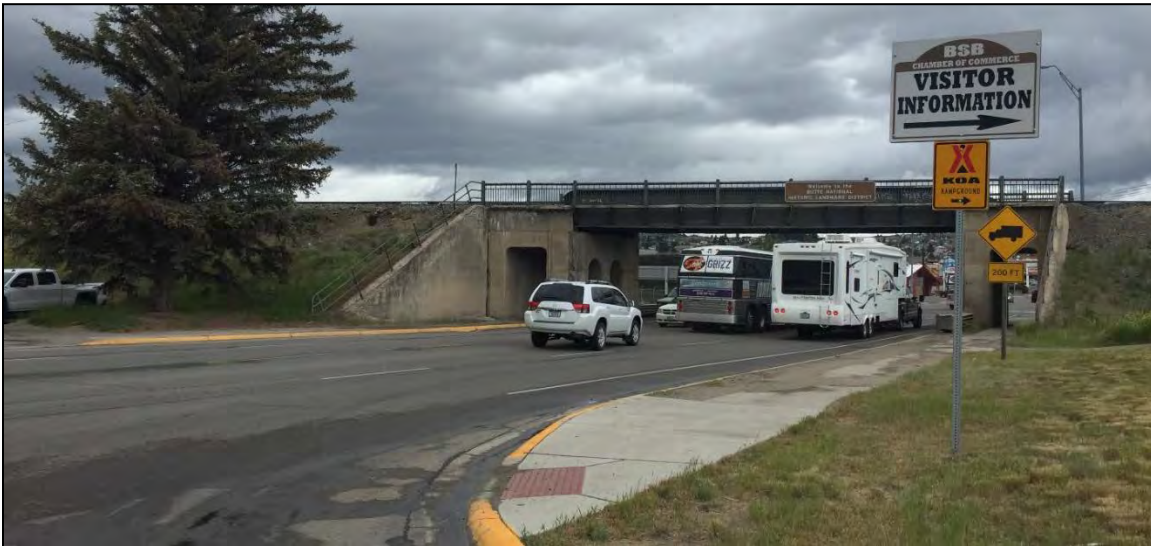
Photograph 3. The intersection of Montana and George would benefit from a southbound left-turn lane, but the road width is restricted by the nearby railroad structure.
