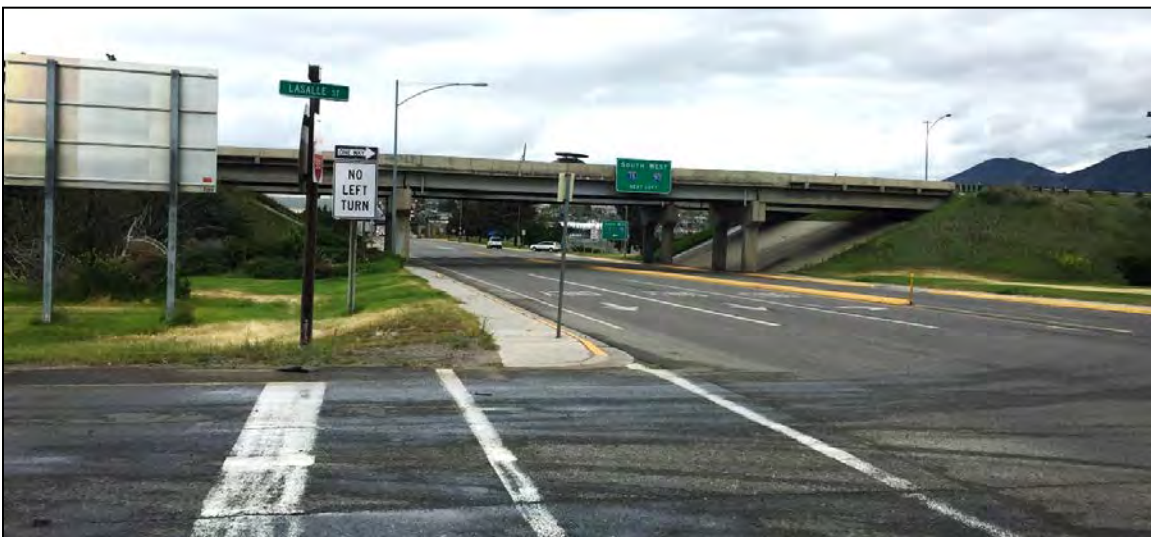
Photograph 2. The intersection of Montana and La Salle should be reviewed for traffic signal warrants.
