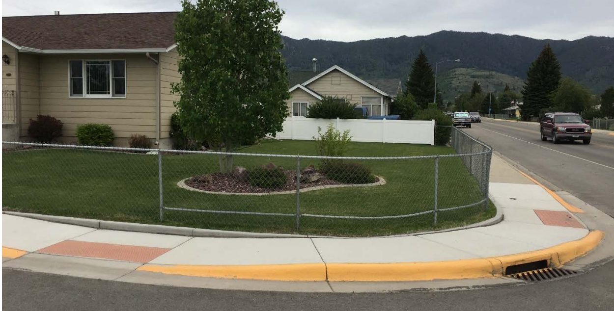
Photograph 6. Street corner showing an updated ADA-compliant sidewalk.
