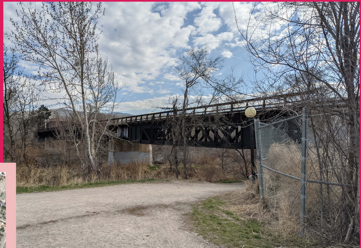
Existing Montana Rail Link Trestle
