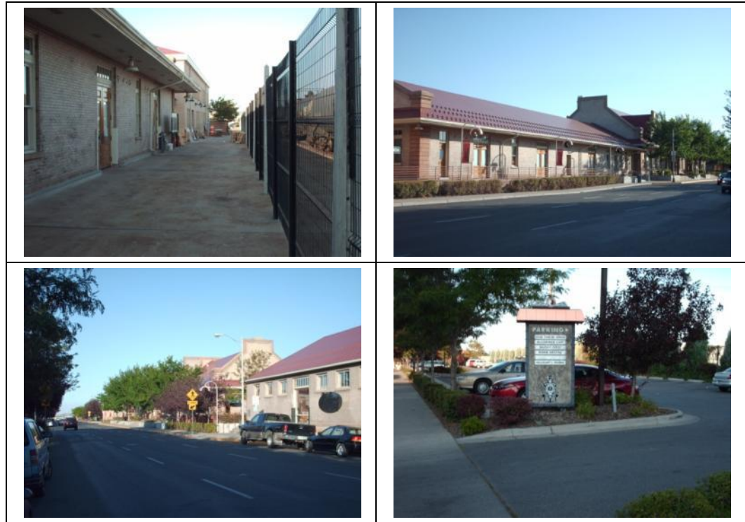
Figure 4.4 Station Photos Billings, Montana
