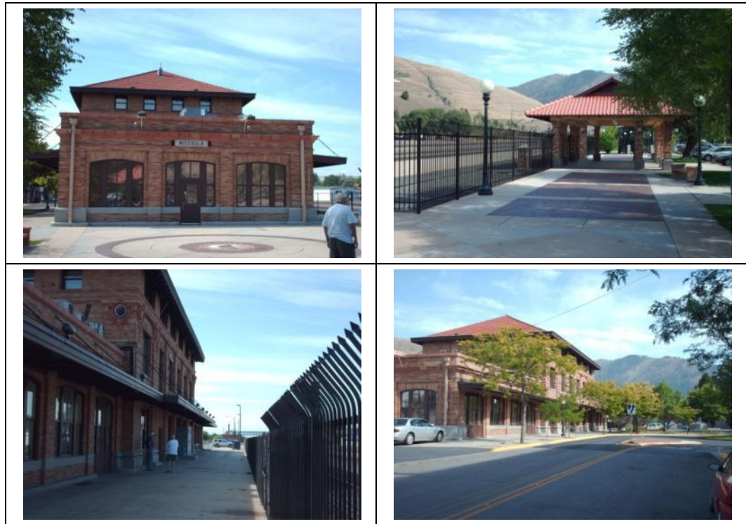
Figure 4.8 Station Photos Missoula, Montana
