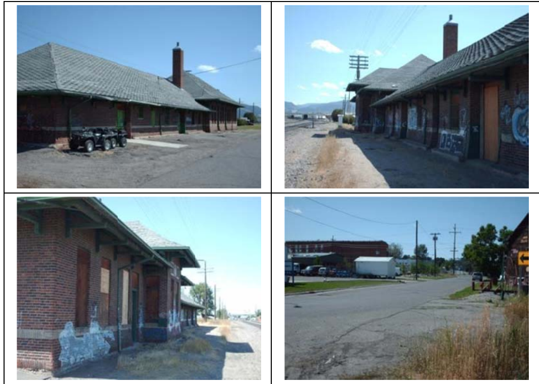
Figure 4.6 Station Photos Bozeman, Montana
