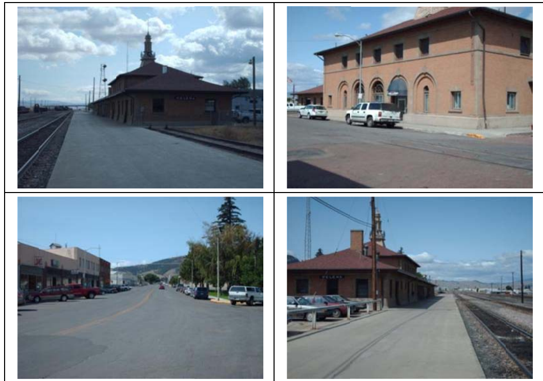
Figure 4.7 Station Photos Helena, Montana
