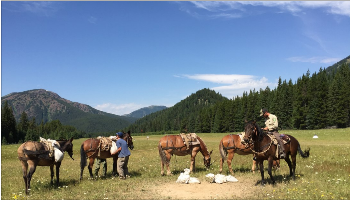
The U.S. Forest Service pack string hauled in feed sacks filled with river gravel to fill-in mule wallows near the airstrip and tie down area. Since Schafer is in the Bob Marshall Wilderness, no wheel vehicles are permitted, so the pack mules are put to good use for maintaining the airstrip.
