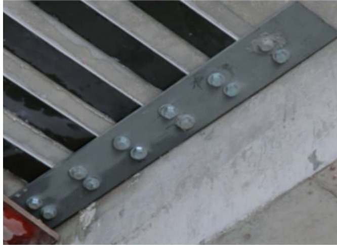
Figure 4: Example mechanical anchorage system [23].
