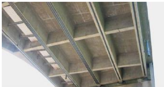
Figure 28: Repaired Louisa Fort Gay bridge girders [39].
