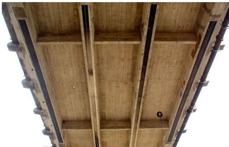
Figure 30: FRP-strengthened Uphapee Creek bridge girders [40].
