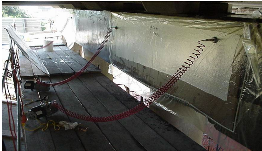
Figure 39: Vacuum bagging system adopted in repairing the Salt Pond Road Bridge [44].
