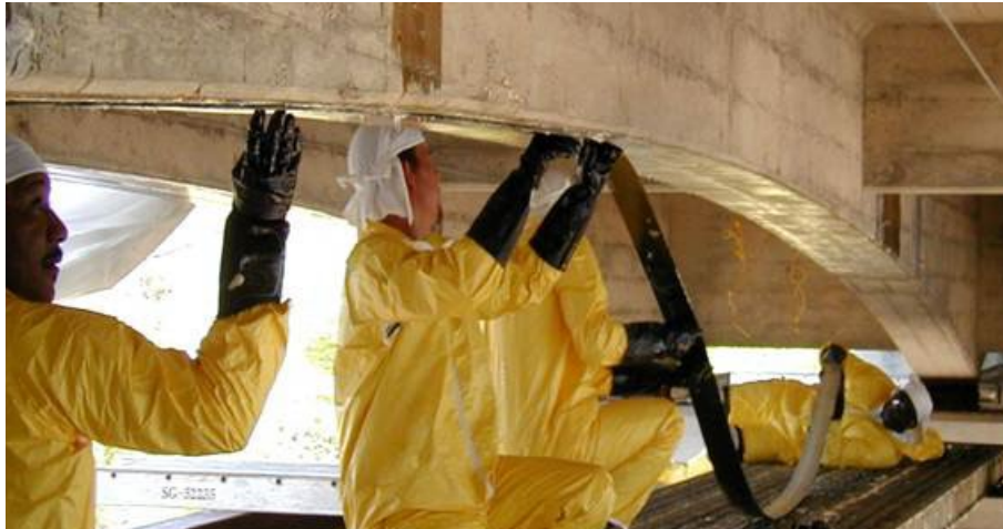
Figure 29: Application of FRP strip to the Uphapee Creek bridge girder [40].
