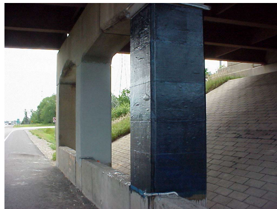
Figure 35: Repaired I-96 overpass bridge columns [42].
