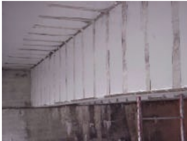
Figure 32: FRP-strengthened girder of State Route 378 bridge, New York [41].
