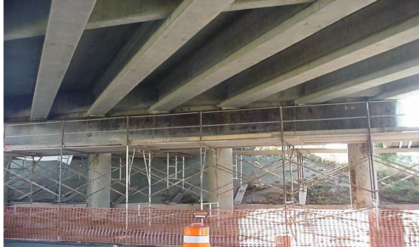
Figure 38: Scaffolding and safety measures for repairing the Salt Pond Road Bridge [44].
