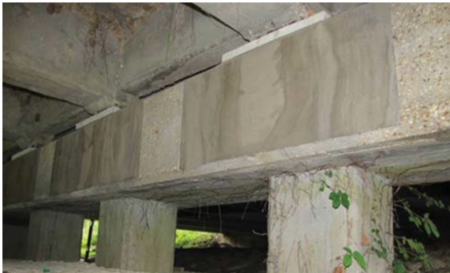
Figure 41: Repaired pile cap of the Morganza Spillway bridge, Louisiana [45].
