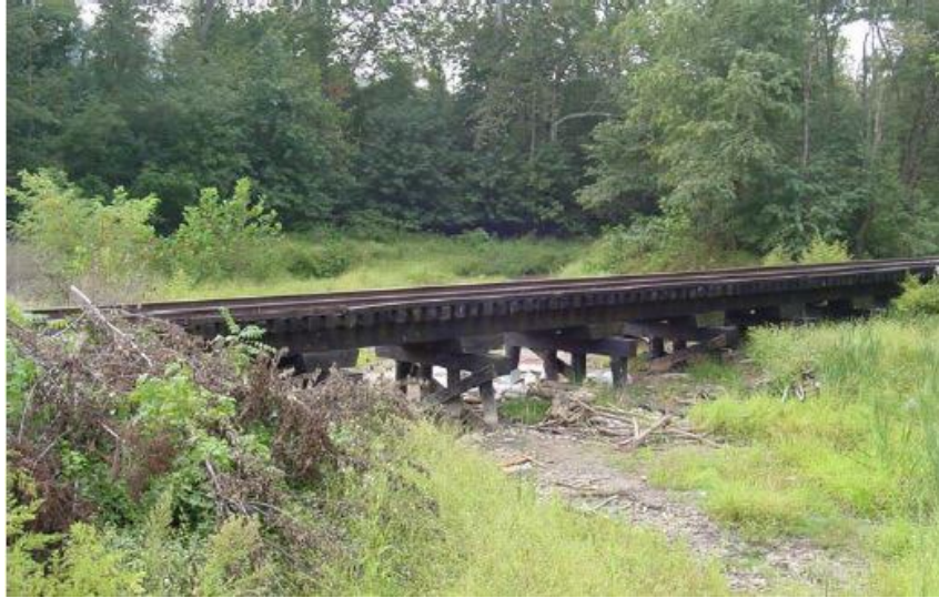
Figure 12: Photograph of timber railroad bridge in Moorefield, West Virginia [35].
