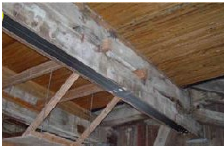
Figure 11: Post monitoring of Sins bridge, Switzerland [34].
