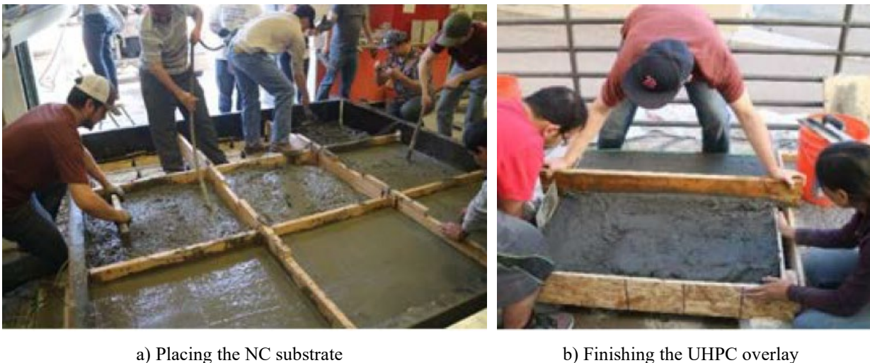
Figure 6: Preparation of UHPC-NC slabs [24]
