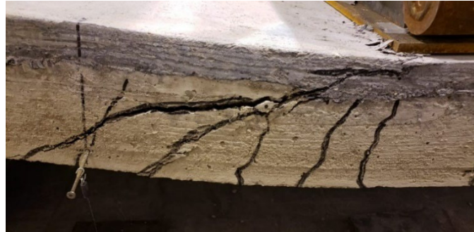
b) Shear crack extending through the overlay
