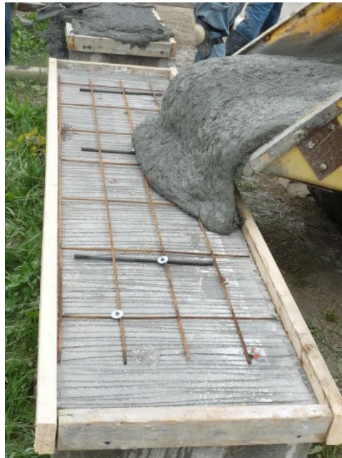
Figure 4: Casting UHPC on slab specimens [23]
