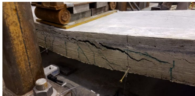
c) Shear crack on other end of slab
