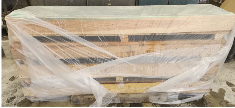
Figure 44: Formwork stacked for curing.
