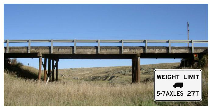
The Montana Department of Transportation (MDT) recently issued a new load posting for the MT 200 Drainage Bridge 14 miles west of Brockway, in McCone County. The posting is part of a multi-year effort to update load ratings and postings on bridges around Montana as mandated by the Federal Highway Administration (FHWA).
