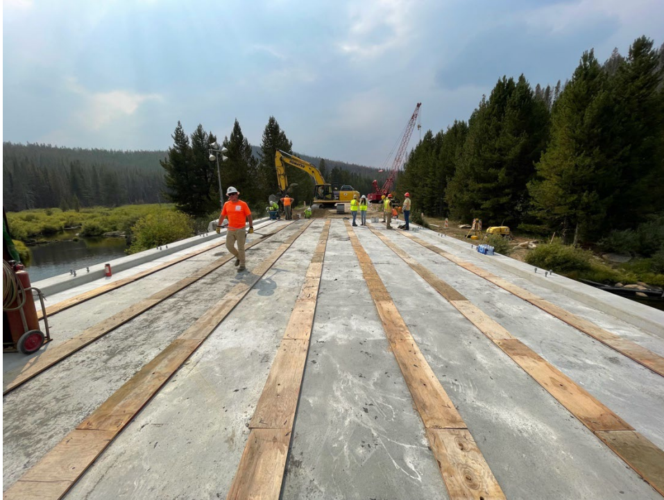
Figure 60: Keyways with top forming
