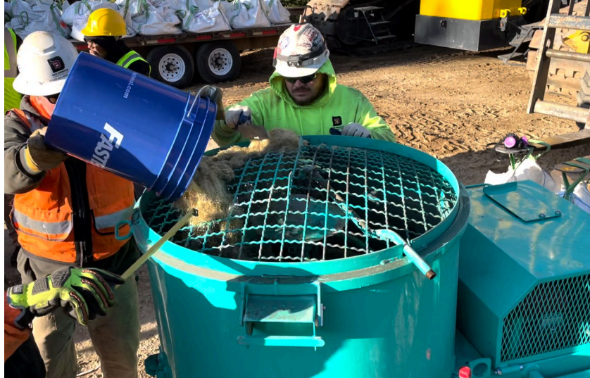
Figure 27: Steel fibers being added to the mixer
