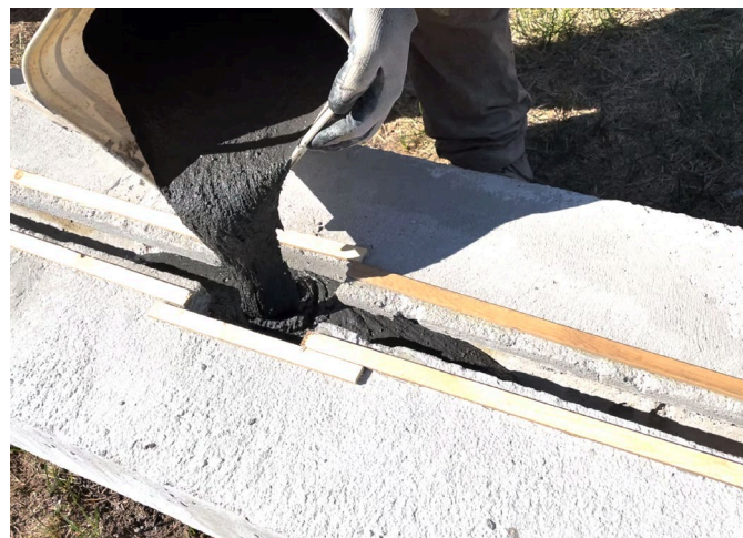
Figure 34: MT-UHPC being placed into keyway mockup
