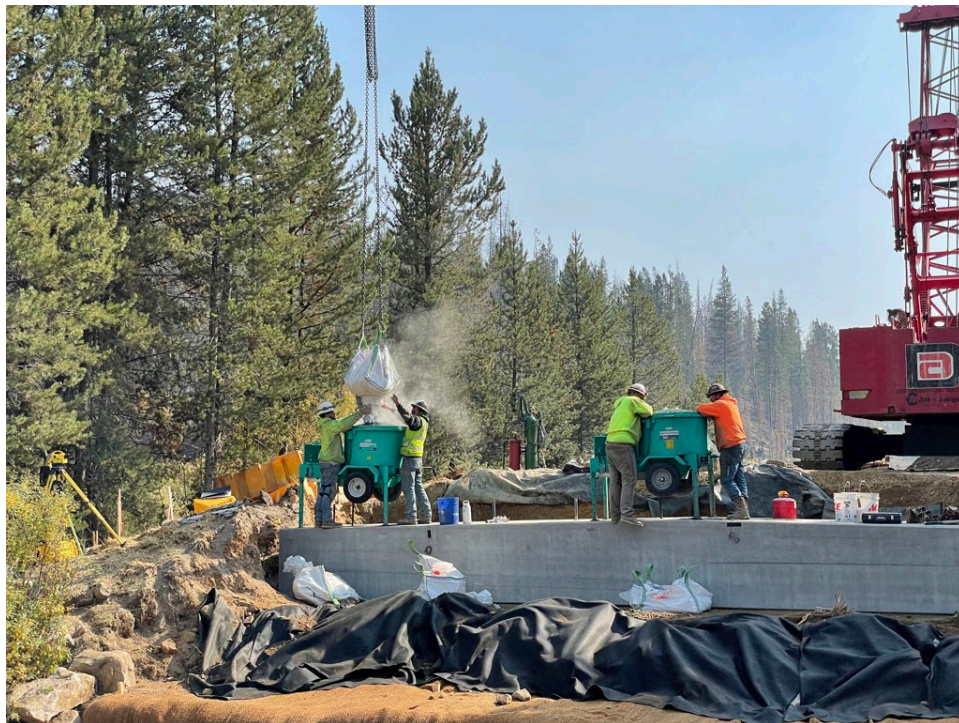
Figure 48: MT-UHPC dry mix being added to mixer on pile cap
