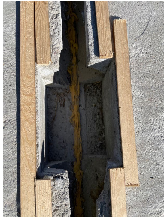
b) inside keyway showing foam sealant
