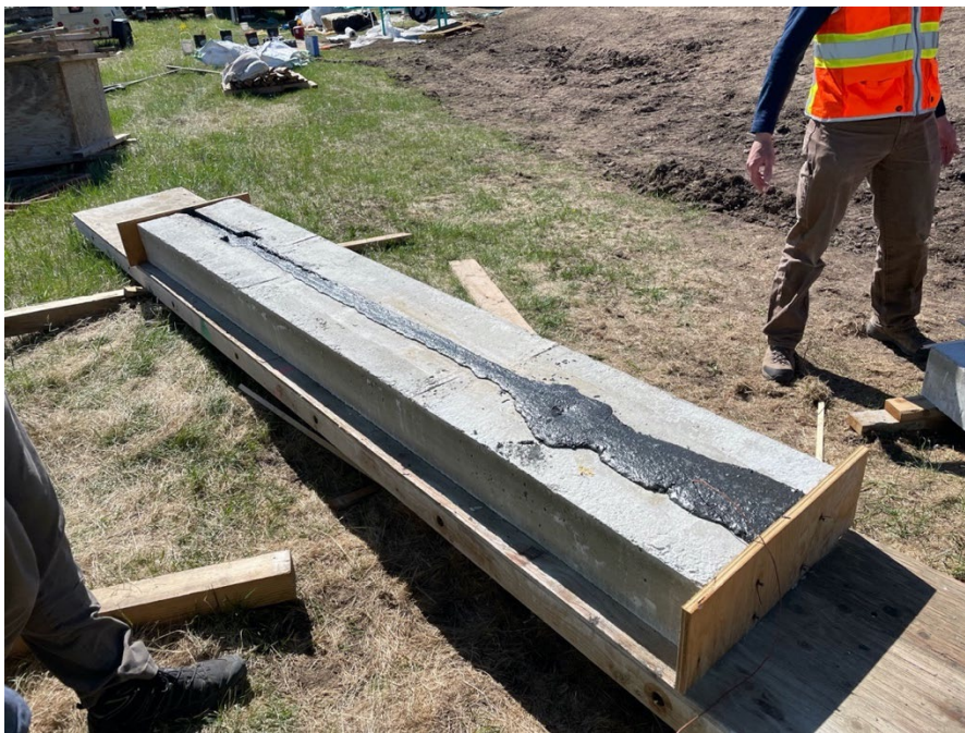
Figure 36: Sloped keyway mockup after MT-UHPC placement
