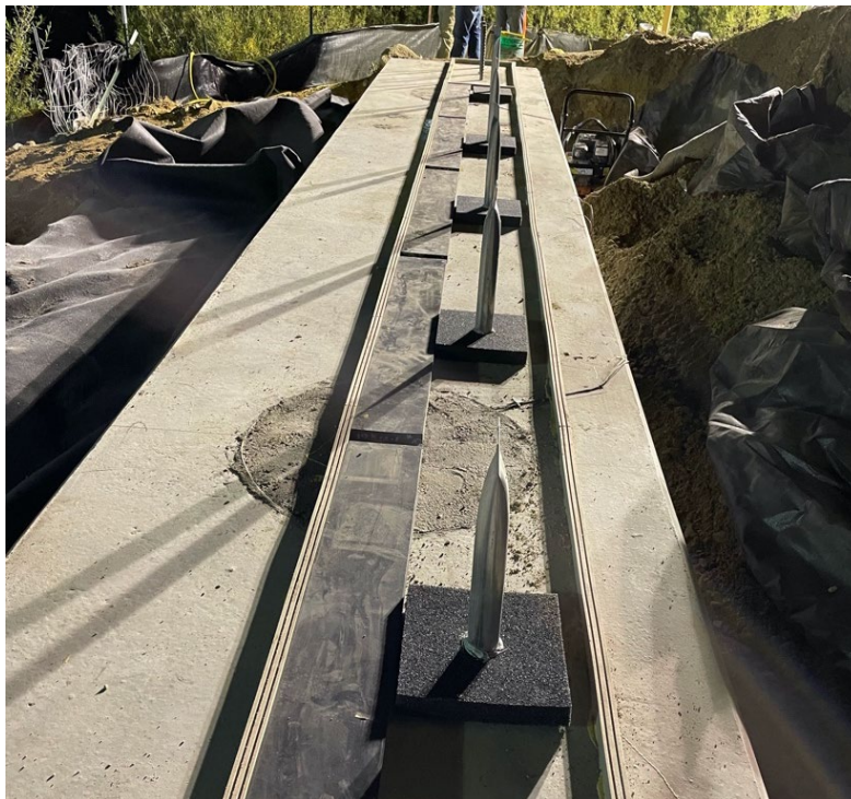
Figure 50: Pile cap after UHPC placement, just prior to the beam placement
