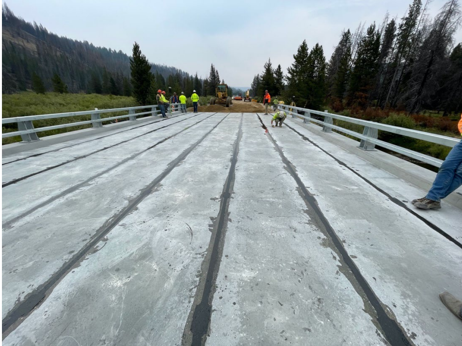
Figure 67: Bridge deck after epoxy application on all keyways
