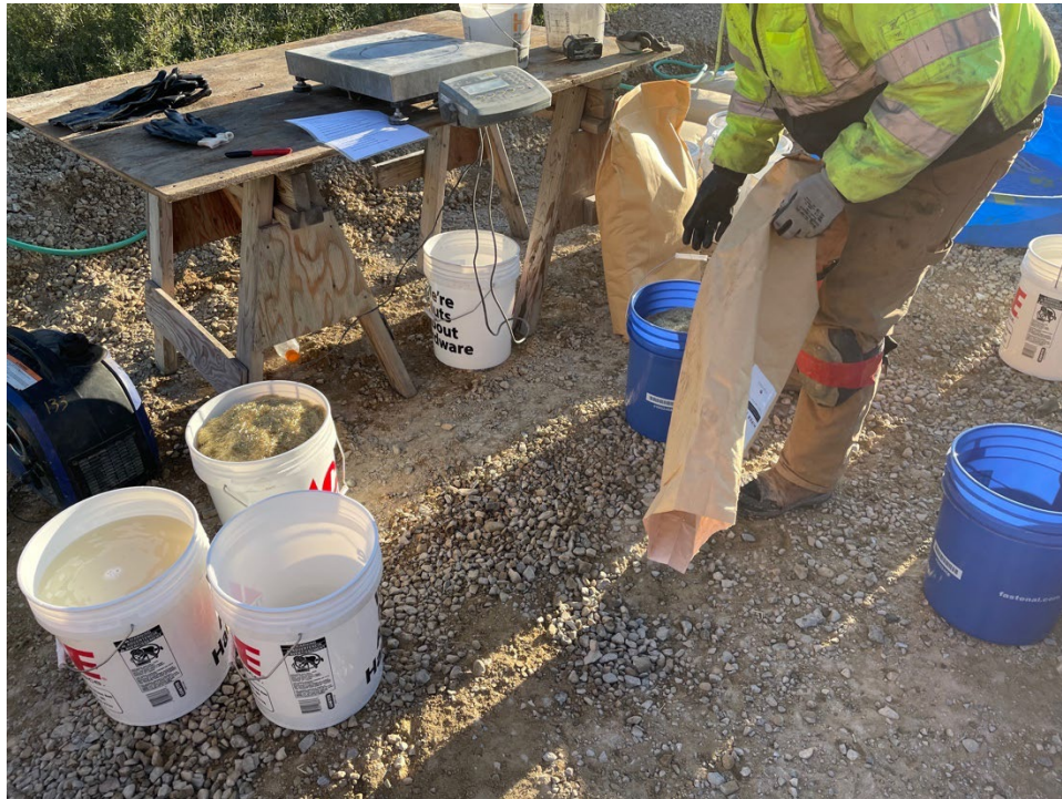
Figure 26: Water, HRWR, and steel fibers being weighed on site
