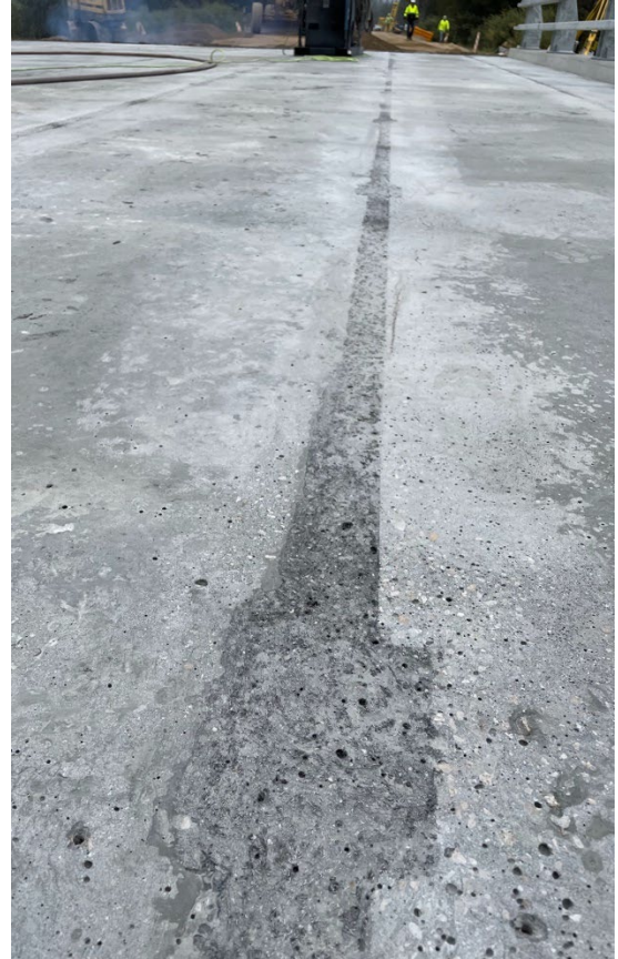
b) keyway with air pockets
