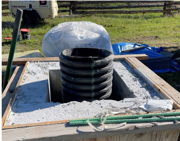
Figure 28: Mockup pile to pile cap connection
