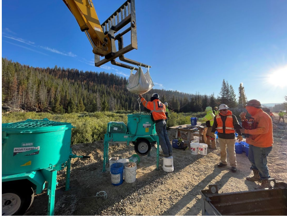
Figure 25: Sack of dry mix being added to the mixer
