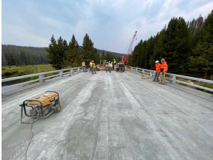
Figure 64: Bridge deck immediately after keyway grinding
