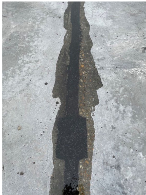
Figure 66: Finished keyway after epoxy application
