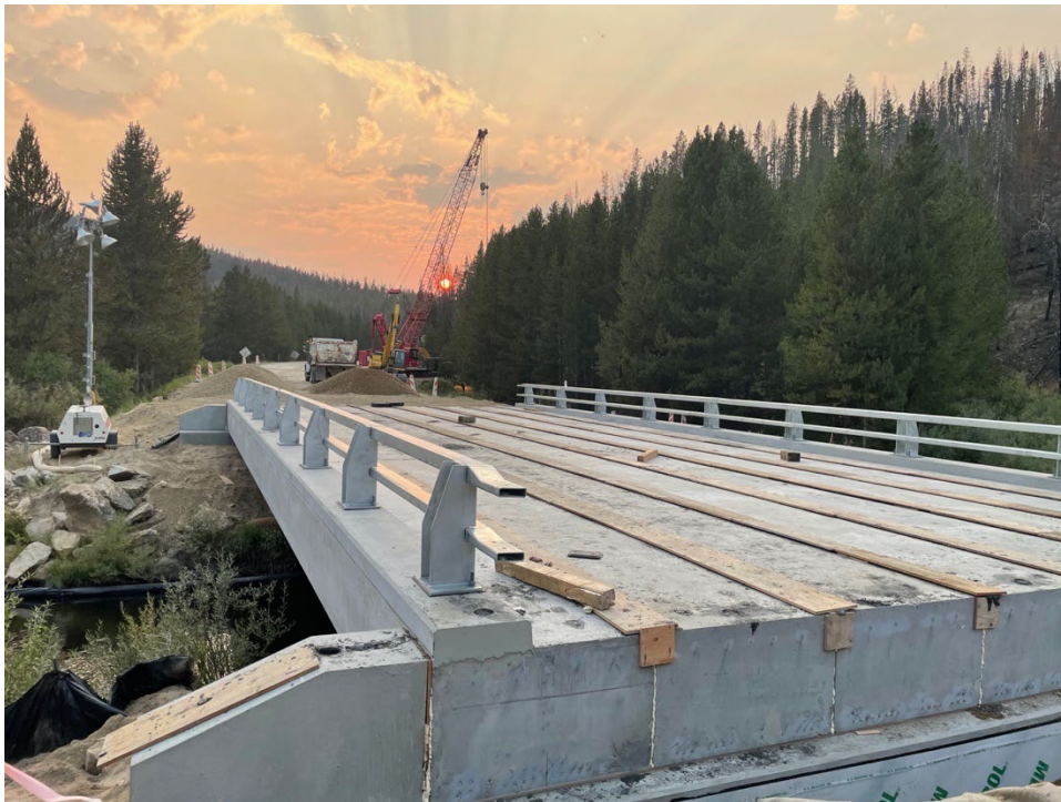
Figure 61: Complete bridge with keyways after UHPC placement and top forming
