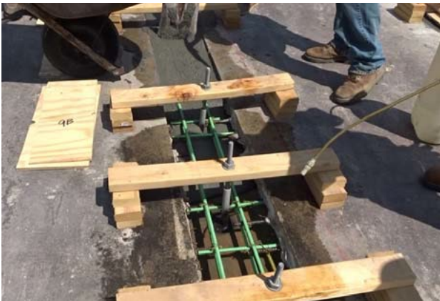
(a) Pre-wetting surfaces and placement of UHPC
