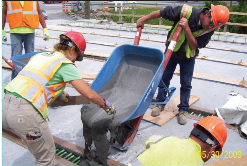
Figure 2: Longitudinal connections placed using a wheelbarrow [3]
