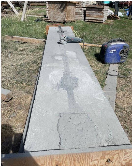
Figure 38: UHPC surfaces ground after a 6-hr cure time
