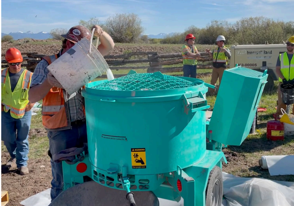
Figure 31: Water and HRWR being added to mixer
