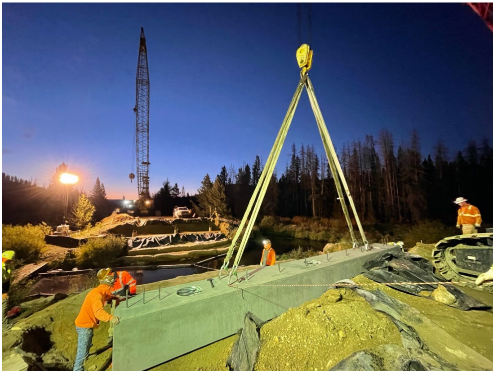
Figure 44: Pile cap being placed on steel pipe piles
