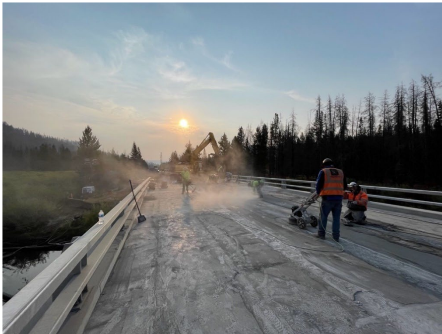
Figure 63: Bridge during grinding process
