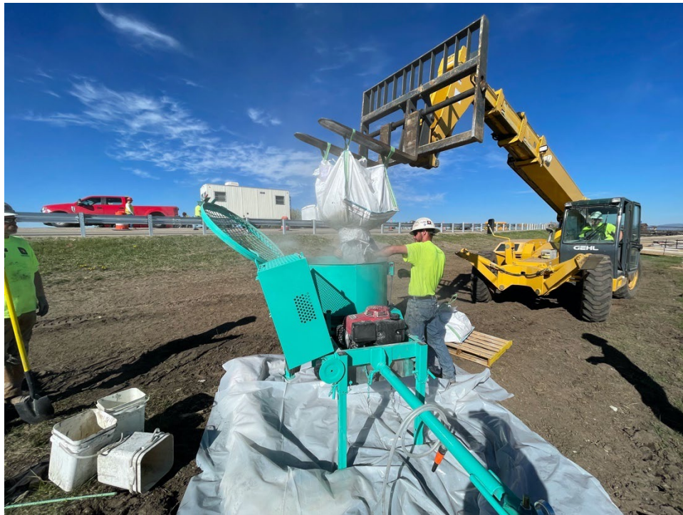
Figure 30: Dry mix being added to mixer
