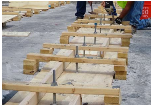
(b) Top forming after placement
