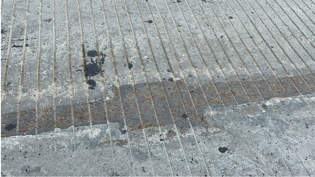
Figure 72: Closeup view of keyway joint in east bridge
