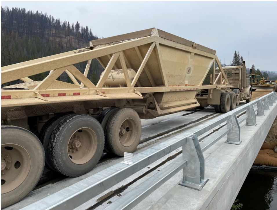
Figure 68: First vehicle to cross bridge after keyways reached required strength
