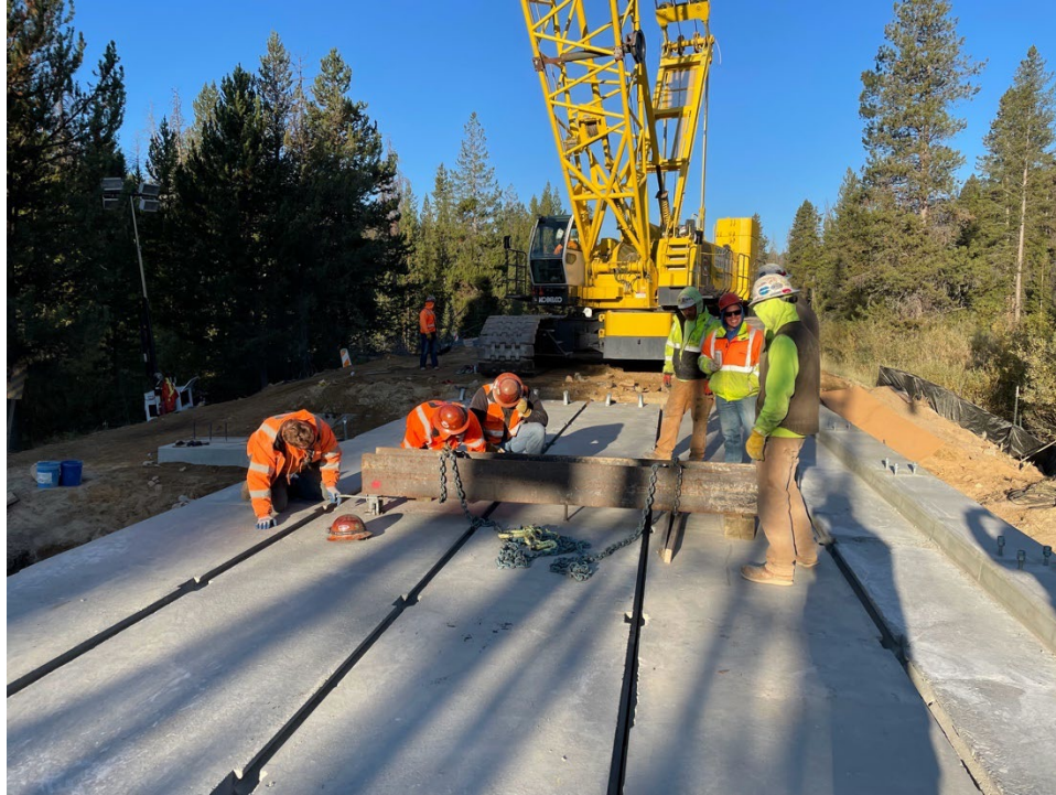
Figure 55: Longitudinal beam elements being leveled
