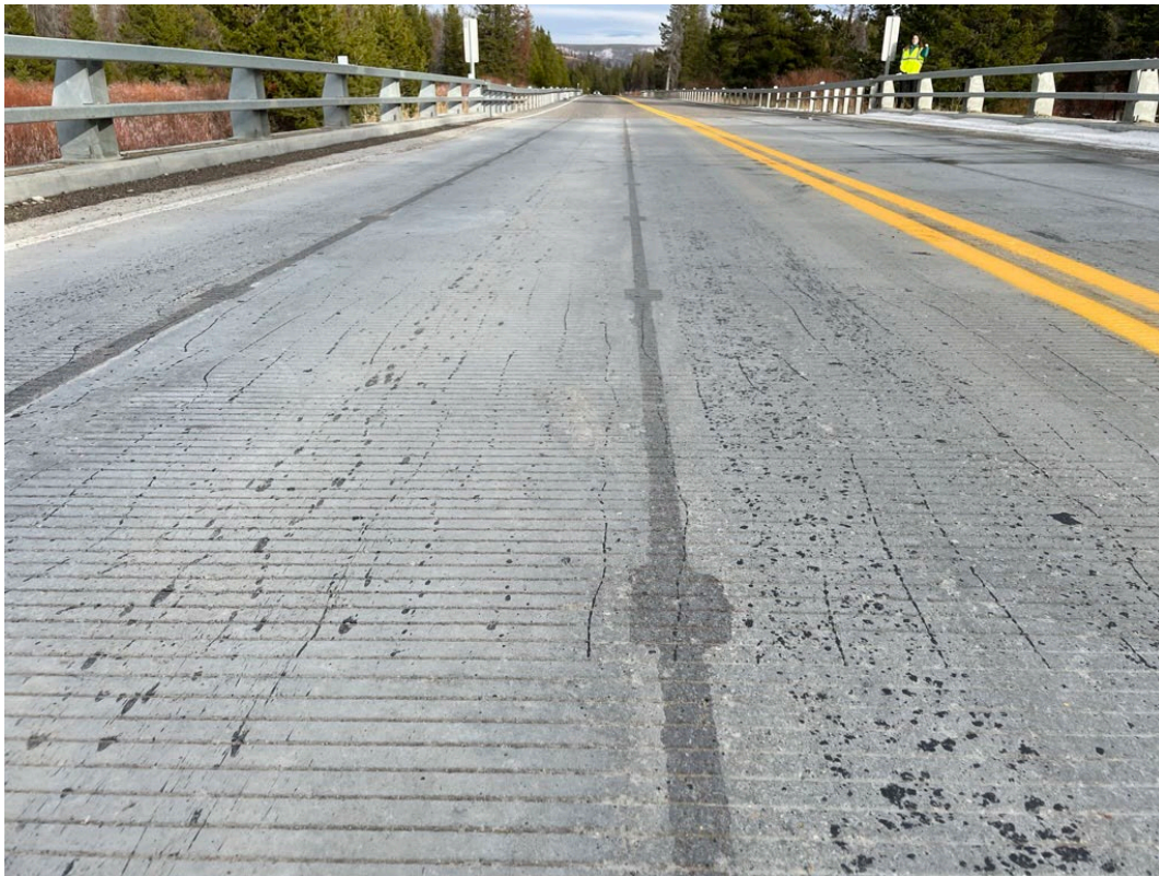
Figure 71: Overview of east bridge
