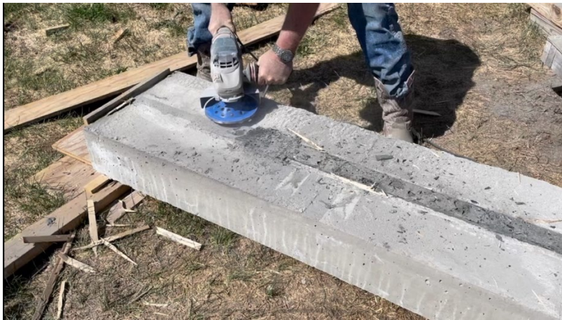
Figure 37: UHPC being ground around keyway
