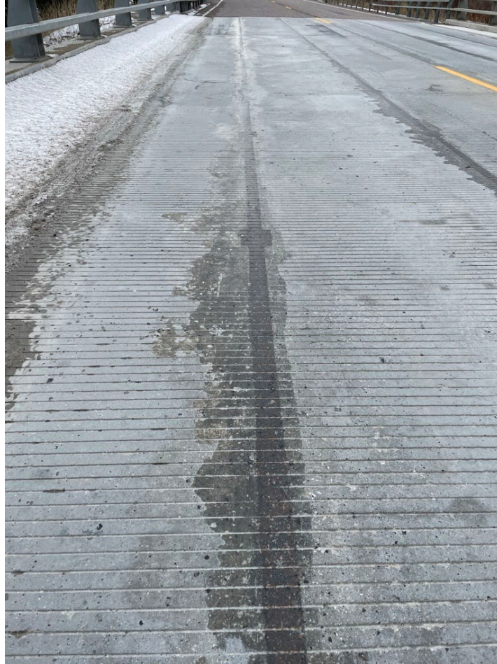
Figure 76: Keyway overview from west bridge
