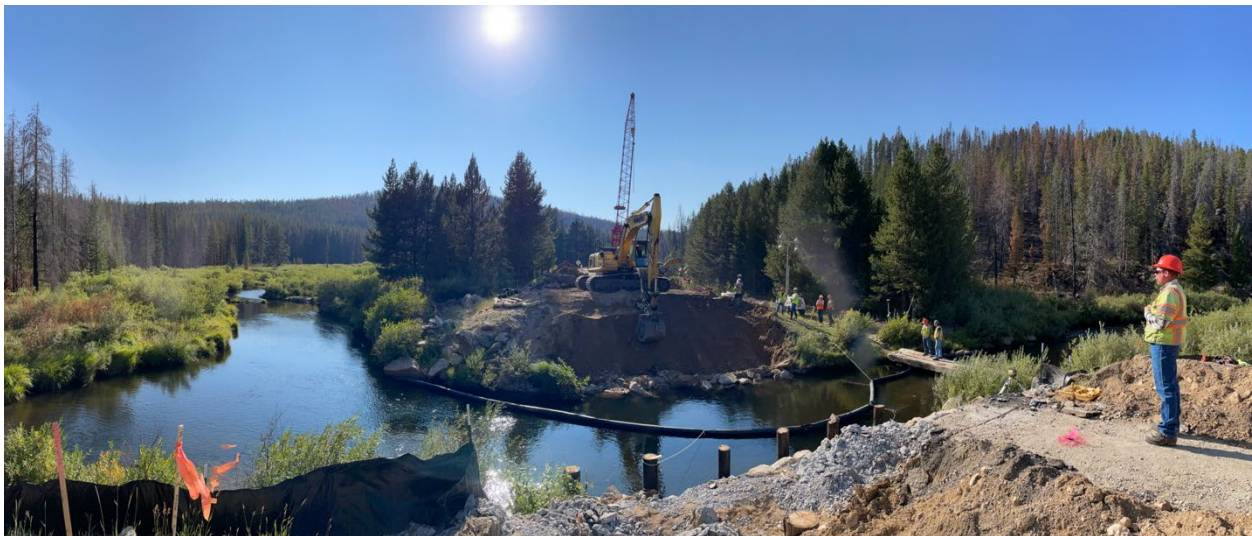
Figure 40: Bridge site after removal of existing bridge
