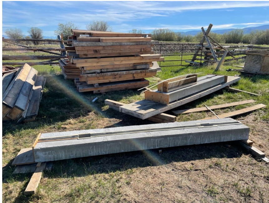
Figure 29: Mockup keyway connections
