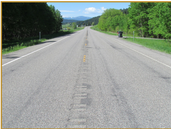
Centerline rumble strip prior to Jointbond application.
