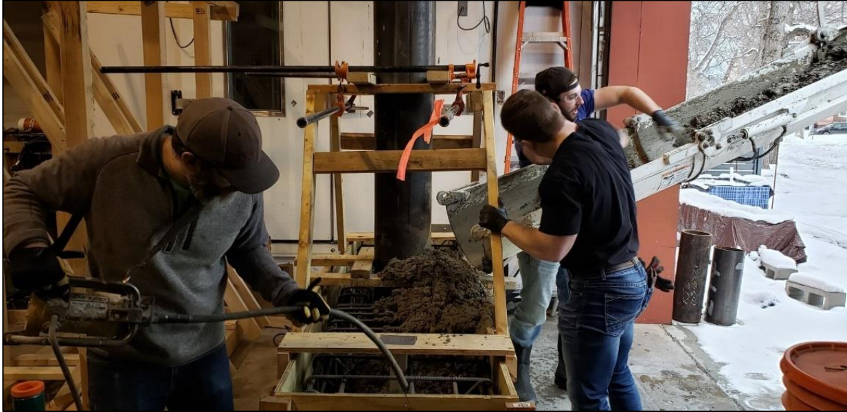
Figure 20: Filling the cap from concrete truck chute
