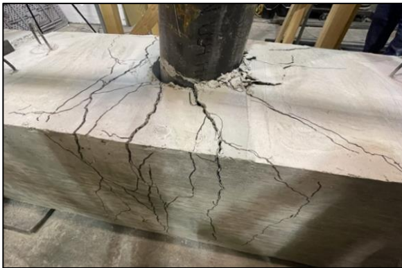
Figure 35: VT2/3-4 failure from initial loading direction
