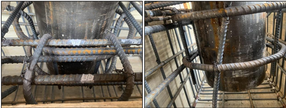
Figure 17: U-Bar placement in VT2/3-4U
