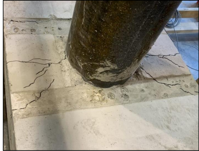
Figure 42: VT2/3-6 45-degree cracks (138 k-ft)
