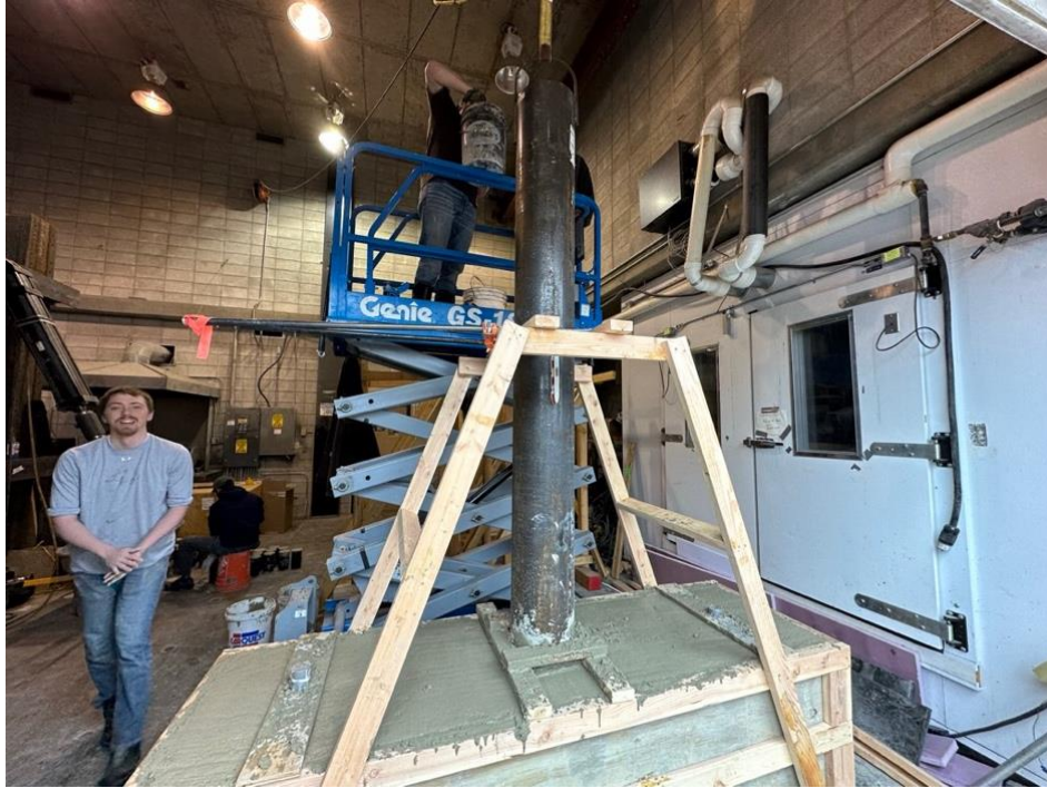
Figure 21: Filling CFST with Concrete
