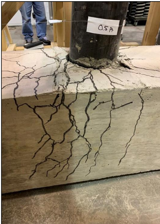
Figure 28: VT1/2-4 failure from initial loading direction
