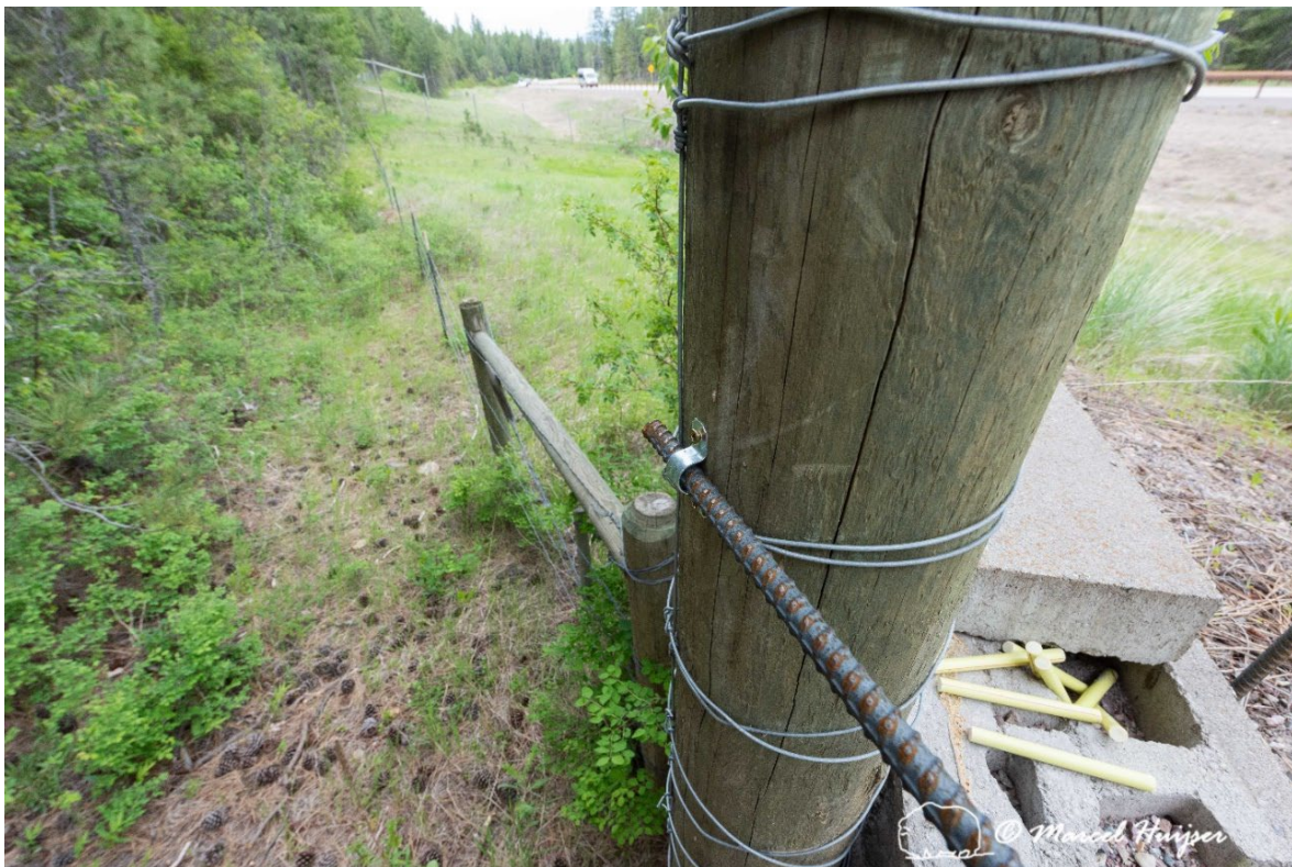
Figure 8: The L-shaped corner elements were connected to the fence posts with brackets and screws.
