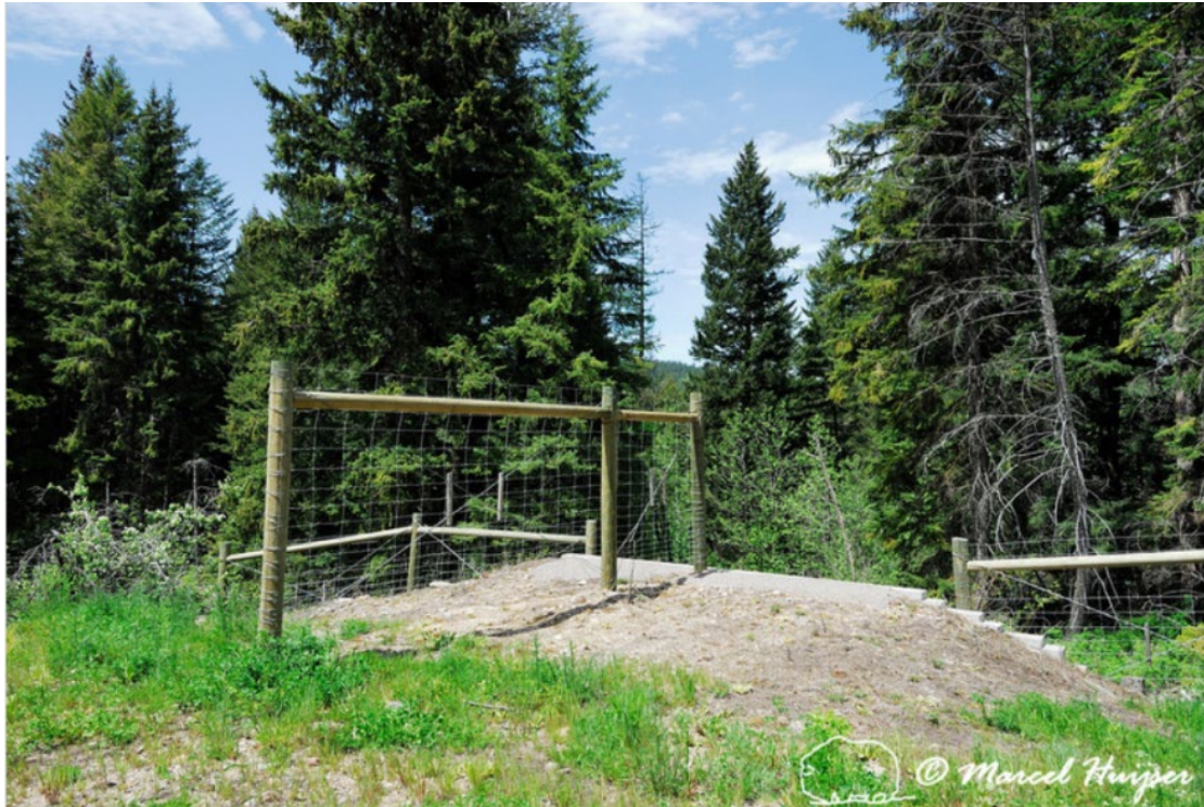
Figure 2: An unmodified jump-out in the Evaro area. The mound allows the animals to walk up to an opening in the fence, with a drop of around 1.83 m (6 ft) to the habitat side of the jump-out.
