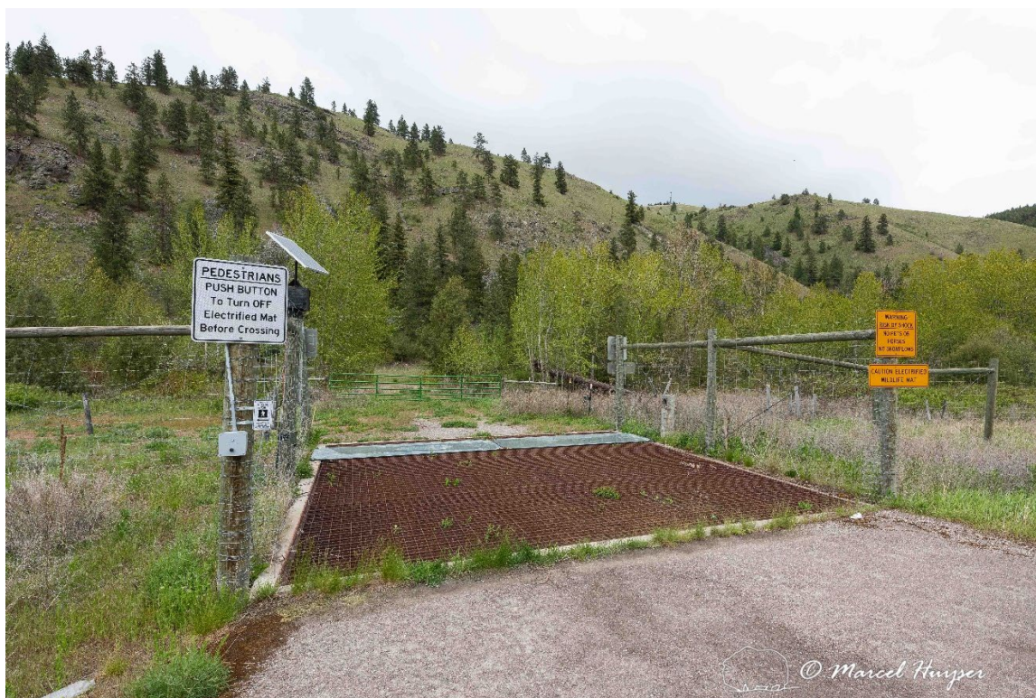
Figure 8: The signs associated with an electrified mat on top of a wildlife guard. There is a set of signs on both the habitat side and the roadside.
