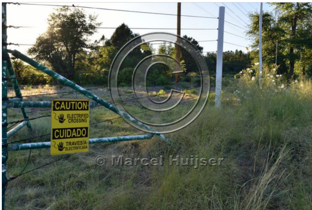
Figure 9: Electric fence associated with an animal detection and driver warning system at a fence end, S.R. 260 east of Payson, Arizona (see Gagnon et al., 2010).
