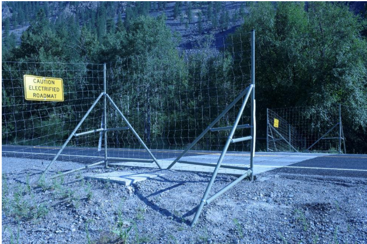
Figure 8: “Caution Electrified Roadmat” sign along MT Hwy 200 near Thompson Falls, Montana.
