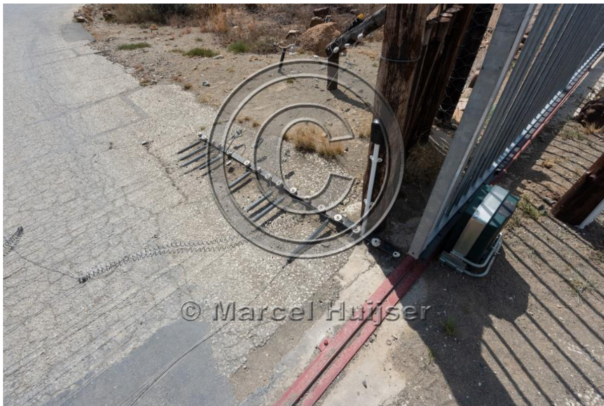
Figure 13: Electrified wires on road surface at gate, South Africa.
