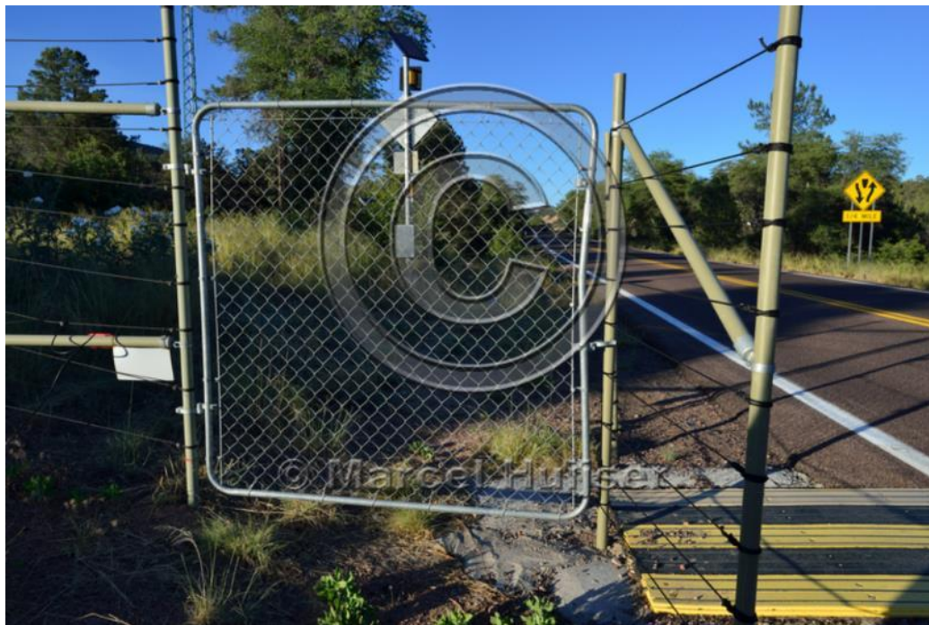
Figure 11: Pedestrian gate at electric fence associated with an animal detection and driver warning system at a fence end, S.R. 260 east of Payson, Arizona.
