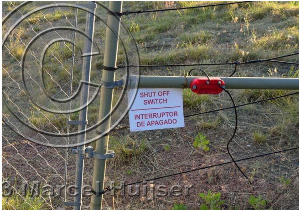
Figure 12: Shut off switch at pedestrian gate at electric fence associated with an animal detection and driver warning system at a fence end, S.R. 260 east of Payson, Arizona.
