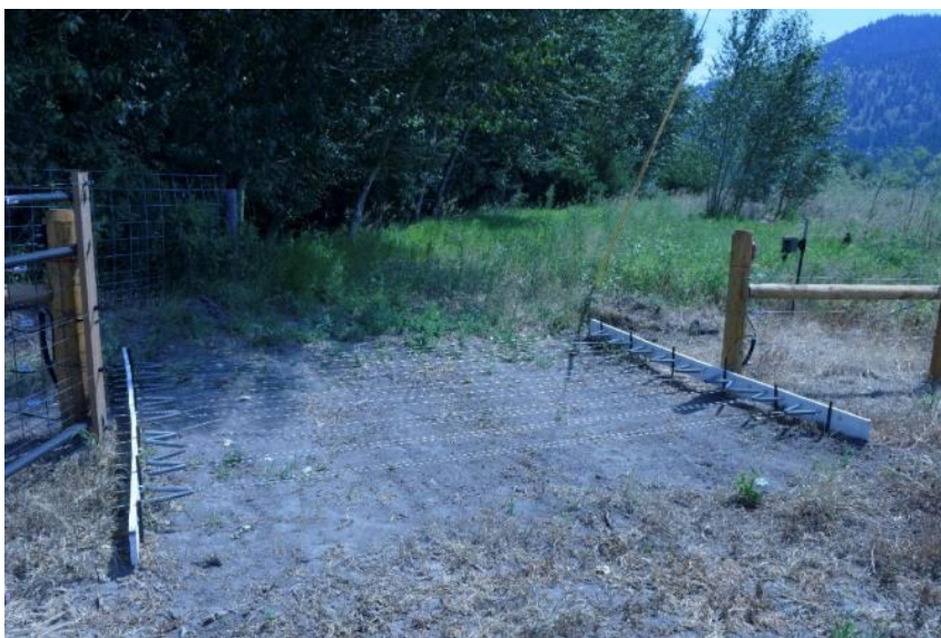
Figure 5: Electrified wires above the ground. Note that a vehicle can drive over these wires.
