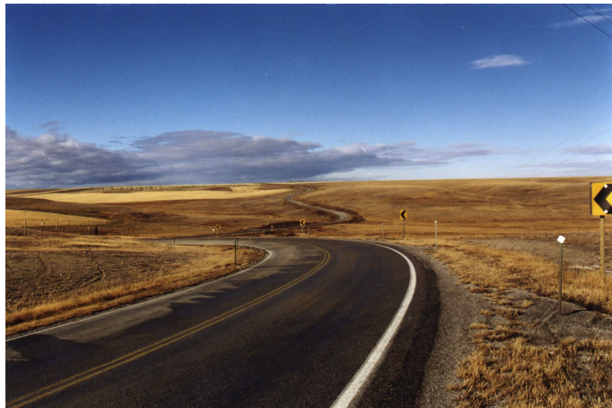
Photo 1-1: View of the northern portion of the corridor, north of Pendroy Junction.
