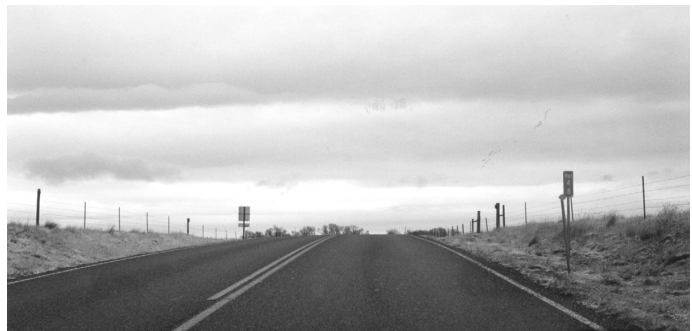
Photo 1-3: Representative substandard vertical curve and poor sight distance north of Choteau.
