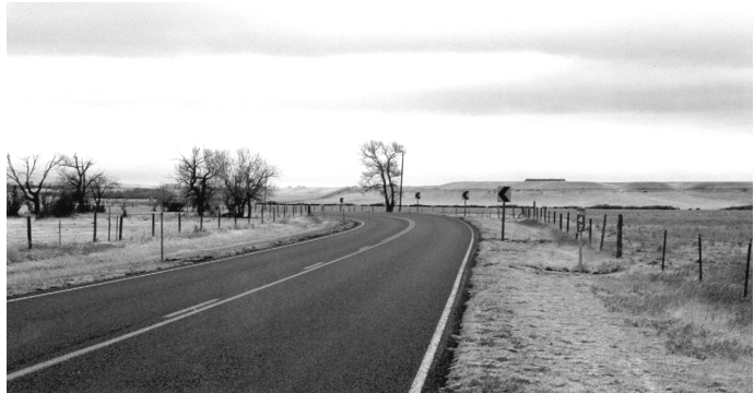
Photo 1-2: Representative substandard horizontal curve north of Choteau.
