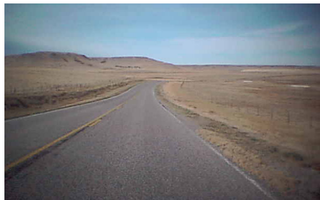
Photo 2-1: View of current roadway width with no shoulders.
