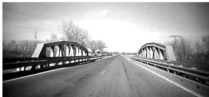
Photo 1-5: View of the Teton River bridge south of Choteau.
