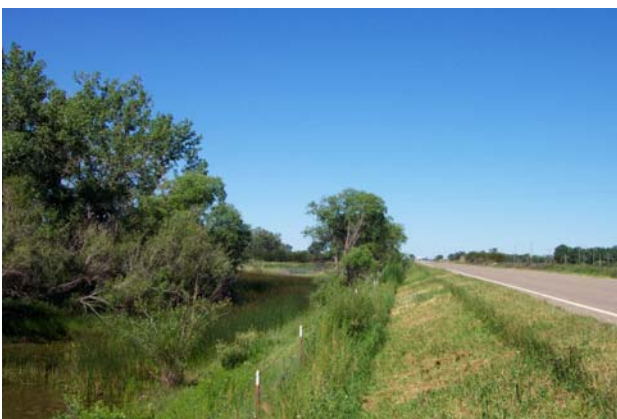
Figure 1.6 Steep side slope in clear zone
