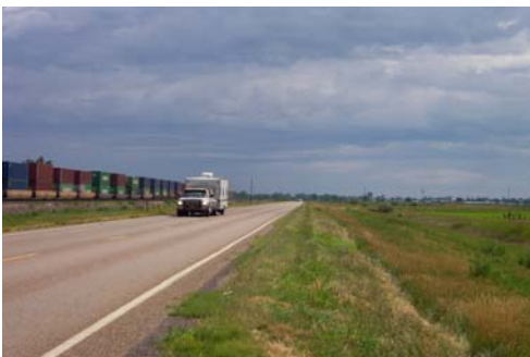
Figure 1.4 Typical narrow shoulder condition
