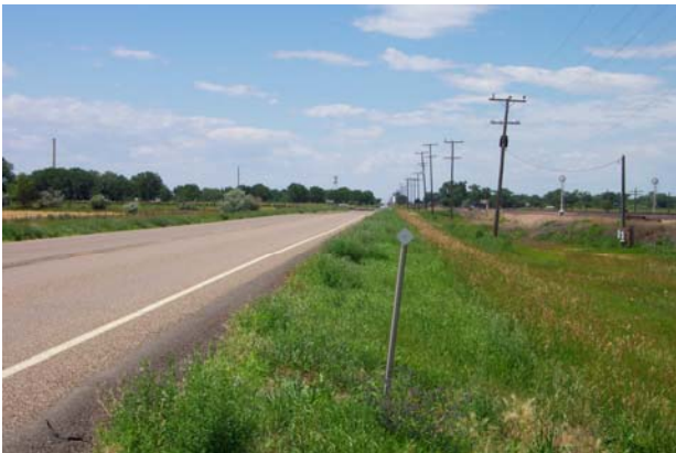
Figure 1.5 Power poles in clear zone
