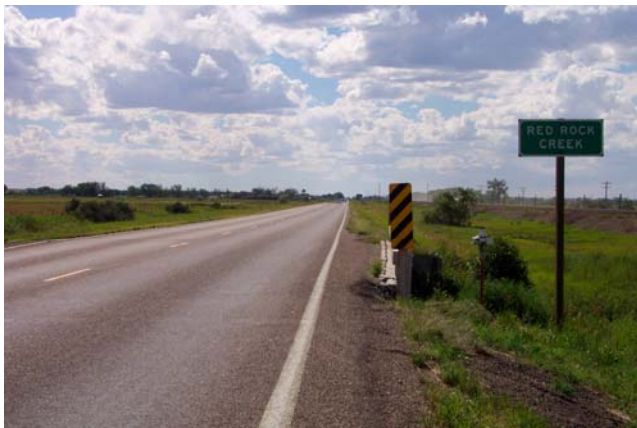
Figure 1.11 Typical bridge with narrow shoulders
