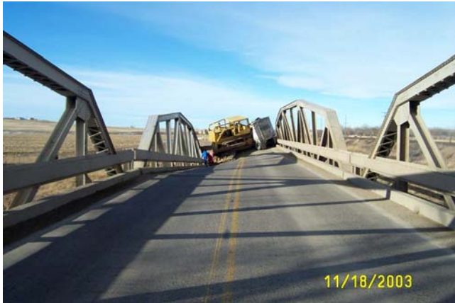
Figure 1.10 Milk River Bridge Collapse
