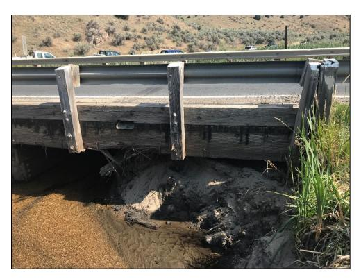
Photo 3. Fine gravel, sand, and silt deposits beneath Highway 287 Bridge over Granite Creek.
