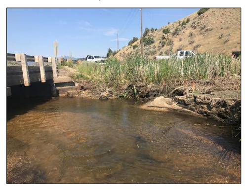
Photo 1. Sediment deposition observed on upstream side of Highway 287 Bridge over Granite Creek
