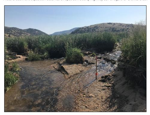
Photo 2. Photo looking upstream from Highway 287 Bridge over Granite Creek showing stream bed aggradation. .
