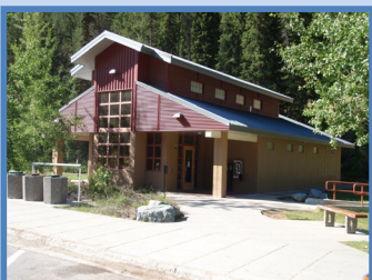
Dena Mora Rest Area
