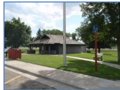
Bridger Rest Area
