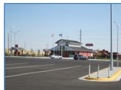
Harlowton Rest Area
