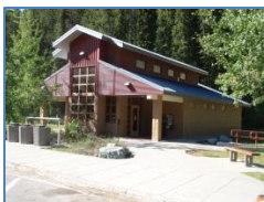
Dena Mora Rest Area
