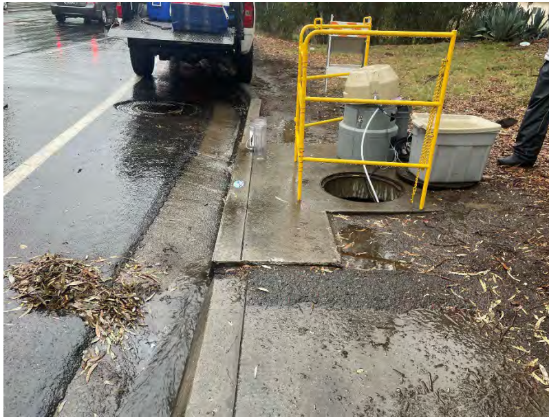
Figure 4-8b. Example of Temporary Automated Sampler Setup
