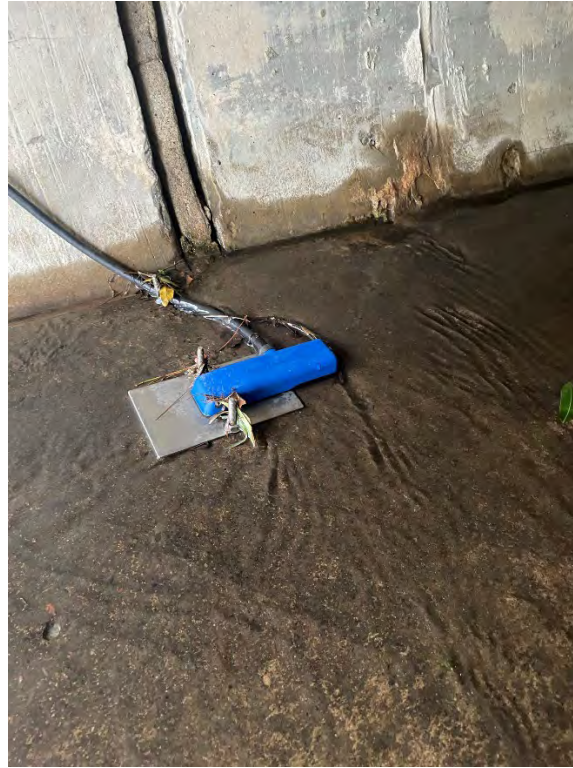
Figure 4-6. Example of Flow Sensor Installation
