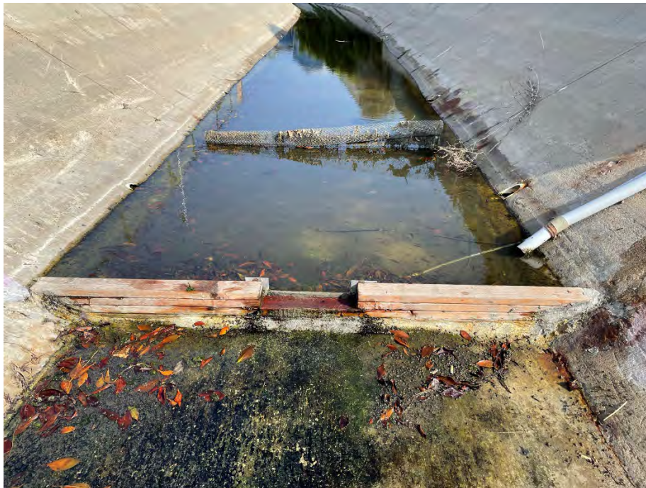
Figure 4-3. Rectangular Weir
