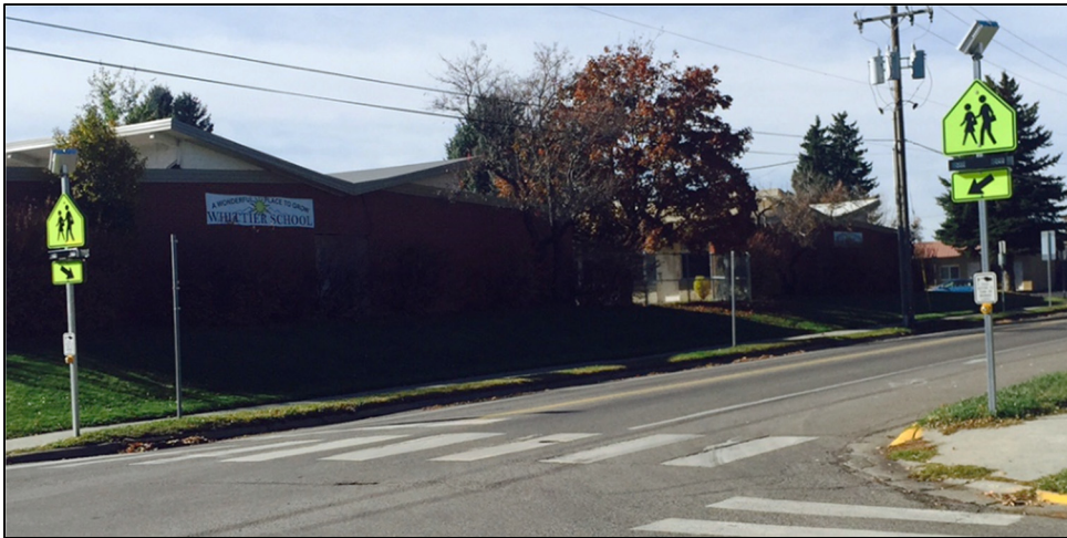
RRFBs in front of Whittier School on Peach Street
