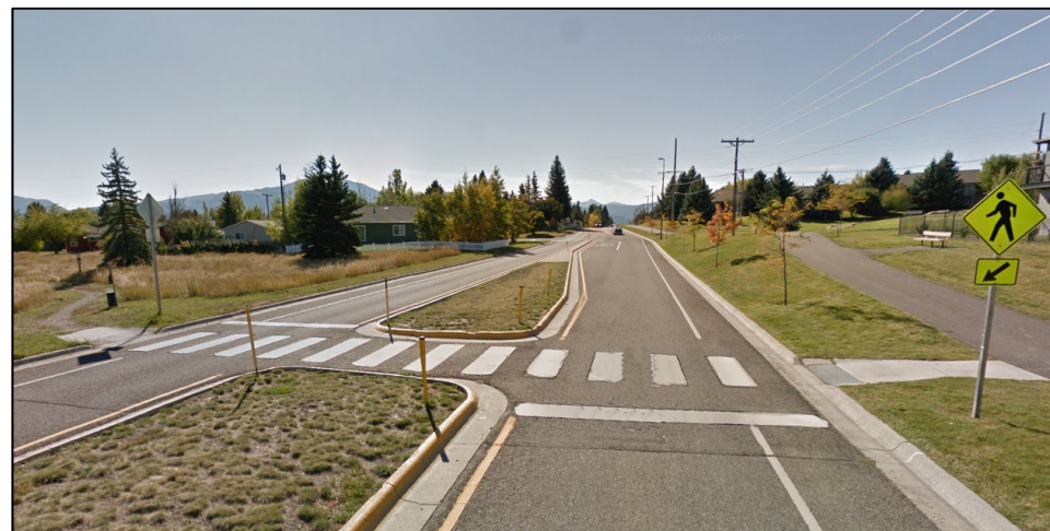
Existing pedestrian refuge on Highland Boulevard
