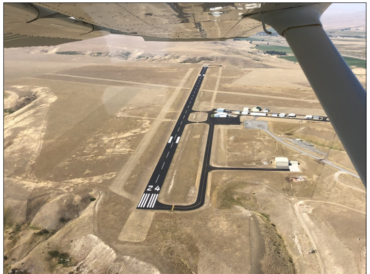
Big Timber Airport after pavement rehab project. Photo Credit: Aeronautics Staff
