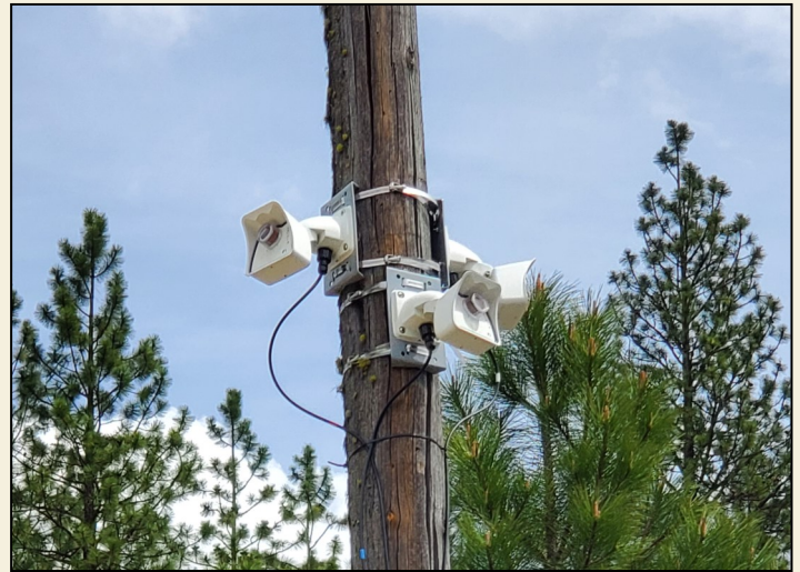
Finished airport weather camera installation. Photo courtesy of Montana Aeronautics.
