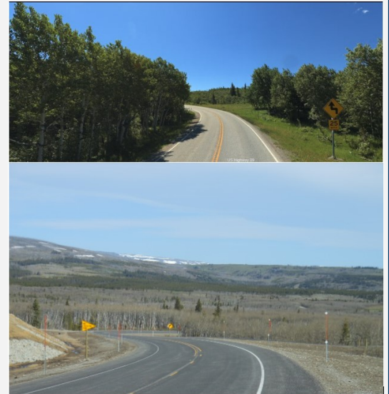
Before (top) and after (bottom) photos of the project corridor demonstrate the widening of US-89 and other safety features of the completed project that received national recognition.
