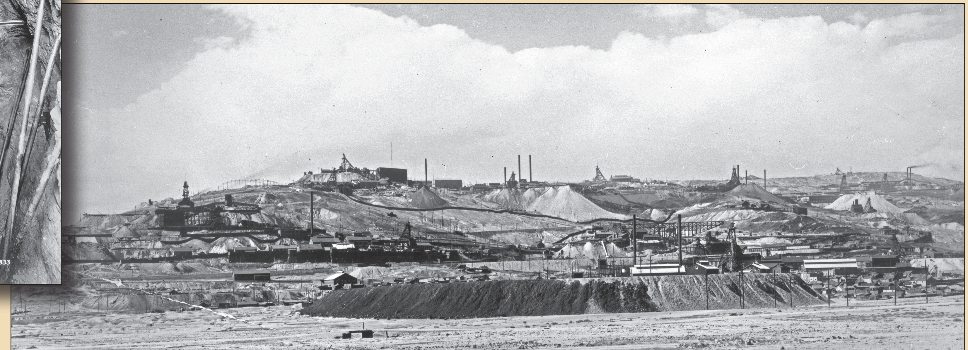
Copper Mines, ACM (Anaconda Copper Mining Co.) Butte, Montana. Meaderville side of Butte Hill. Butte Mines Looking West.
