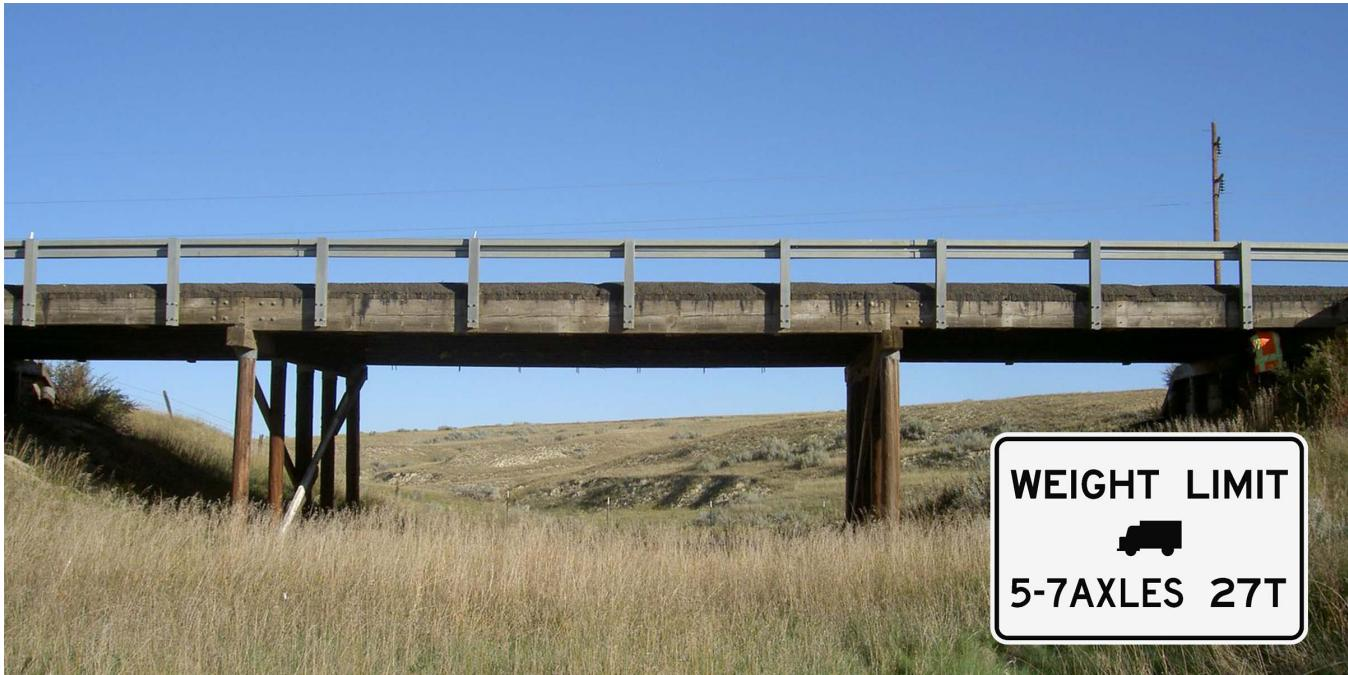
The Montana Department of Transportation (MDT) has issued an updated load posting for the [MT 200 Drainage Bridge](#), 14 miles west of Brockway, in McCone County. The posting is part of a multi-year effort to update load ratings and postings on Montana bridges as mandated by the [Federal Highway Administration](#) (FHWA).
