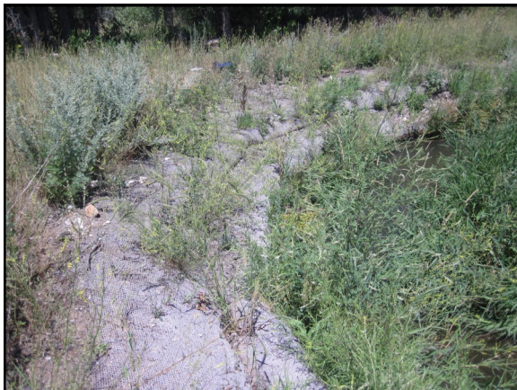
Additional Photo 9 Description: Unvegetated upper soil lift Taken in 2015 looking downstream @ STA 11+25
