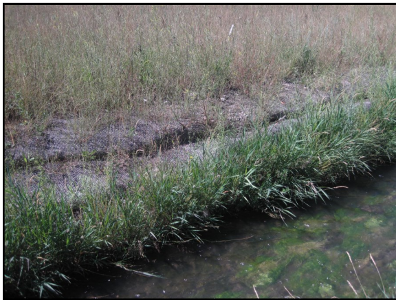
Additional Photo 7 Description: Unvegetated upper soil lift Taken in 2015 looking across channel @ STA 11+00
