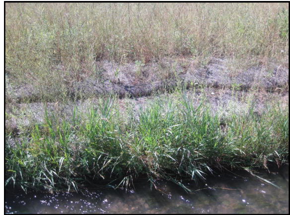
Additional Photo 6 Description: Unvegetated upper soil lift Taken in 2015 looking across channel @ STA 11+00
