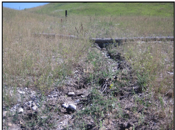
Additional Photo 16 Description: Gully forming east of new channel Taken in 2015
