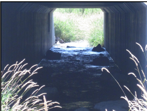
Additional Photo 15 Description: Habitat boulders in box culvert Taken in 2015
