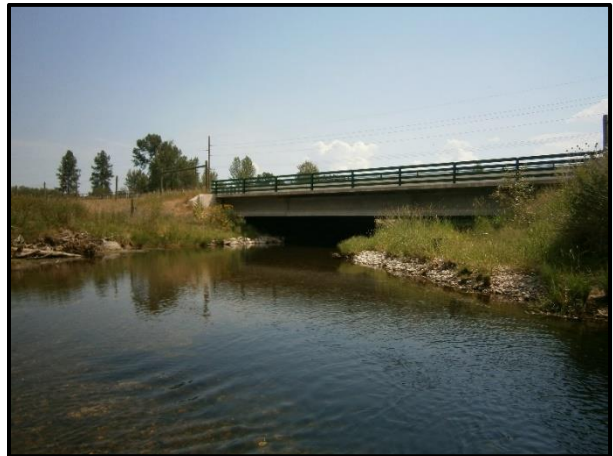
Survey Photo 30. T4 looking East downstream from middle creek.
