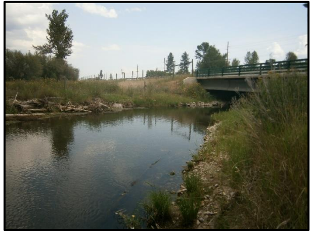
Survey Photo 28. T4 looking East downstream from South bank.
