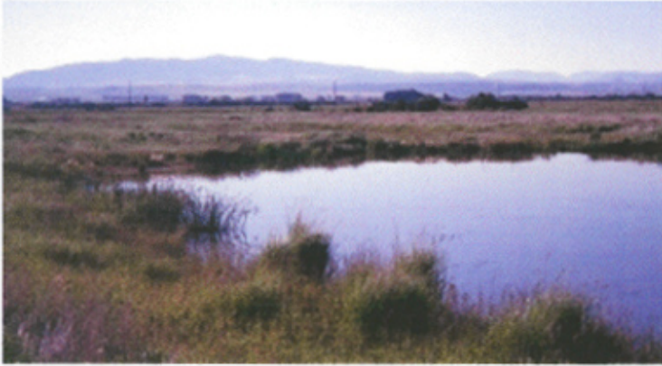
Photo point 1: 90 degrees east Photo taken while standing on top of outlet control structure.
