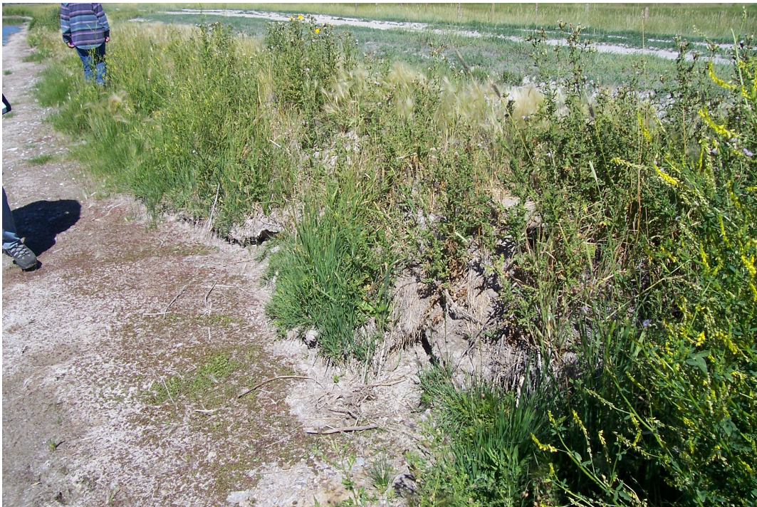
Figure 1. Erosion of upstream face, slowly moving toward crest of dike approximately 375 feet west of overflow structure. Note lack of vegetation on vertical slopes.
