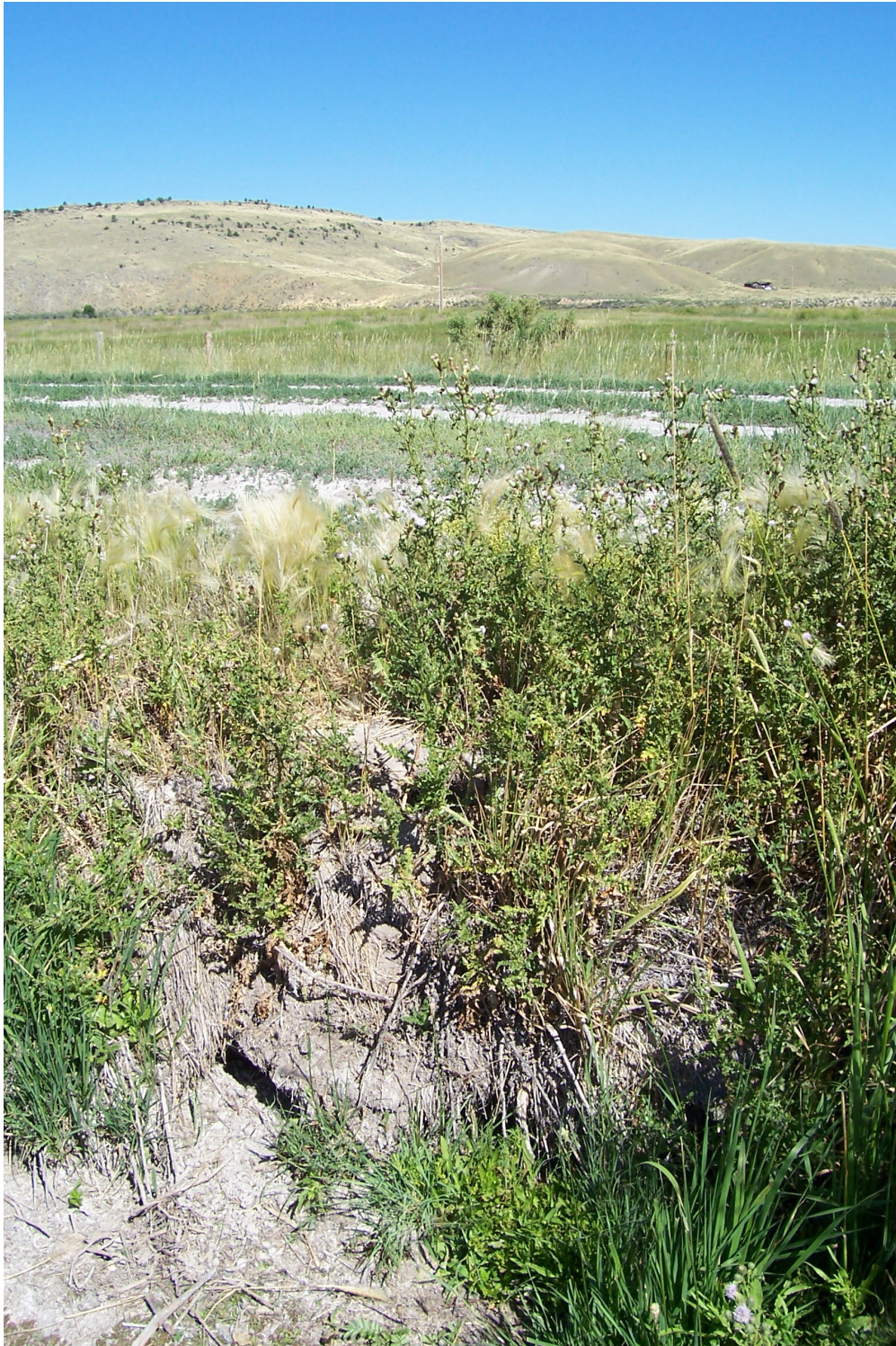
Figure 3. View of upstream face erosion approximately 870 feet west of overflow structure. Vegetation has a difficult time establishing on vertical slopes, so erosion will likely continue. Crest is still 3 feet away, and very wide in this location, so the erosion is not a threat to the safety and stability of the dam at this time.
