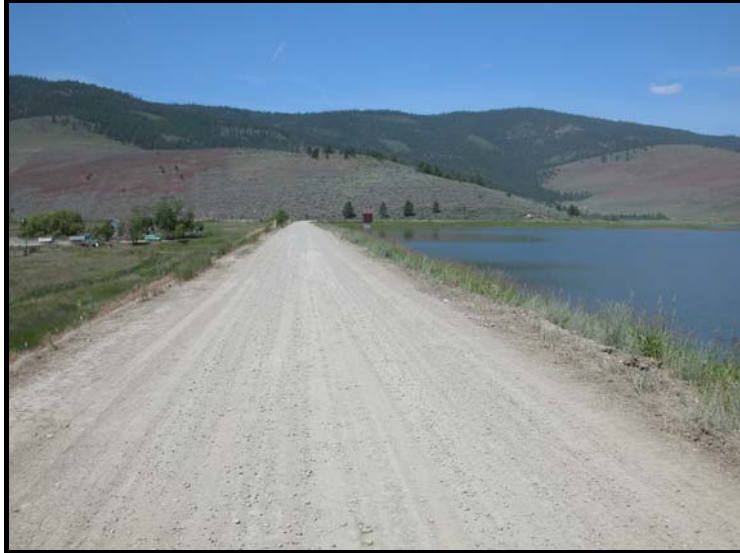
View of dam surface facing west with project site on left.
