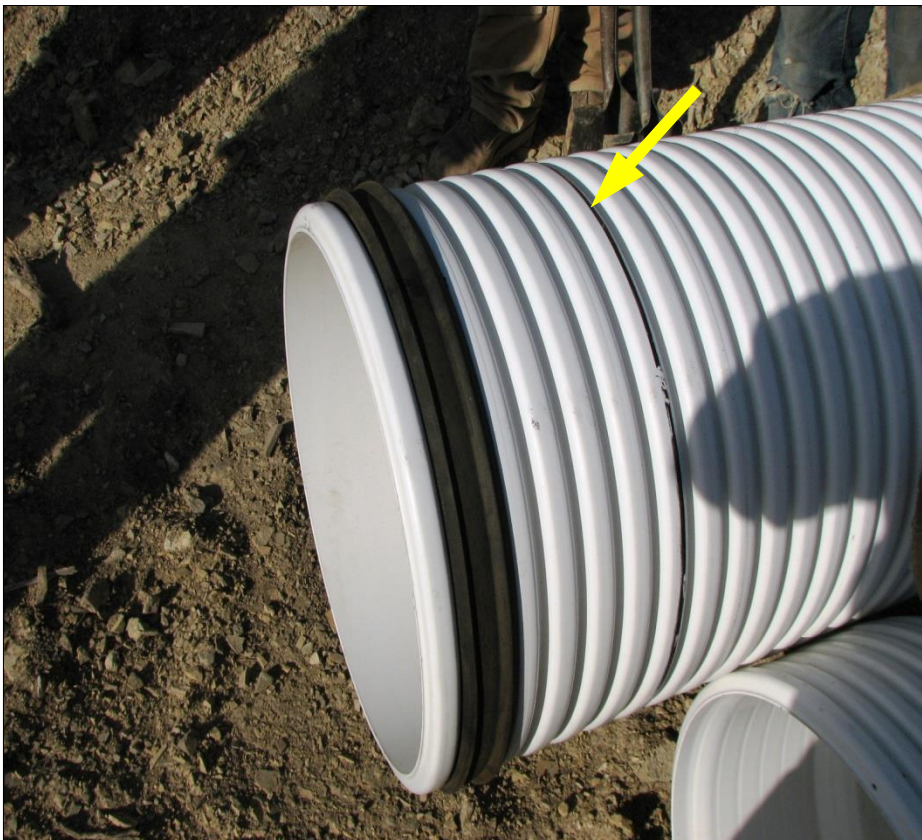
↑ The first section of the A-2000 is placed (view west).
