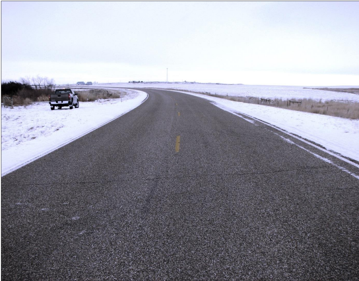
↑ View north. No issues with the roadbed were observed.
