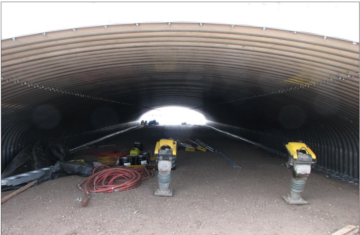
↓ Interior image of completed ABC unit, view looking west.
