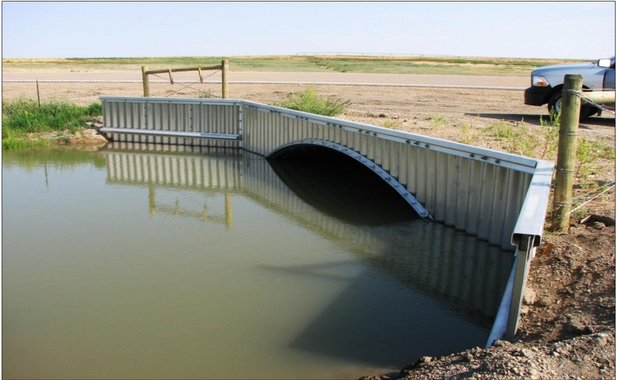
↑ View of culvert inlet.
