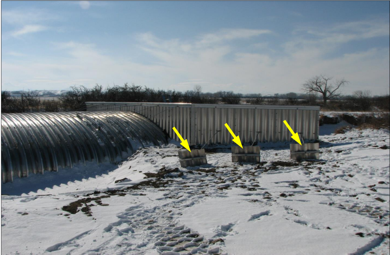
↑ North side of rear inlet wingwall showing three placed deadman anchors.
