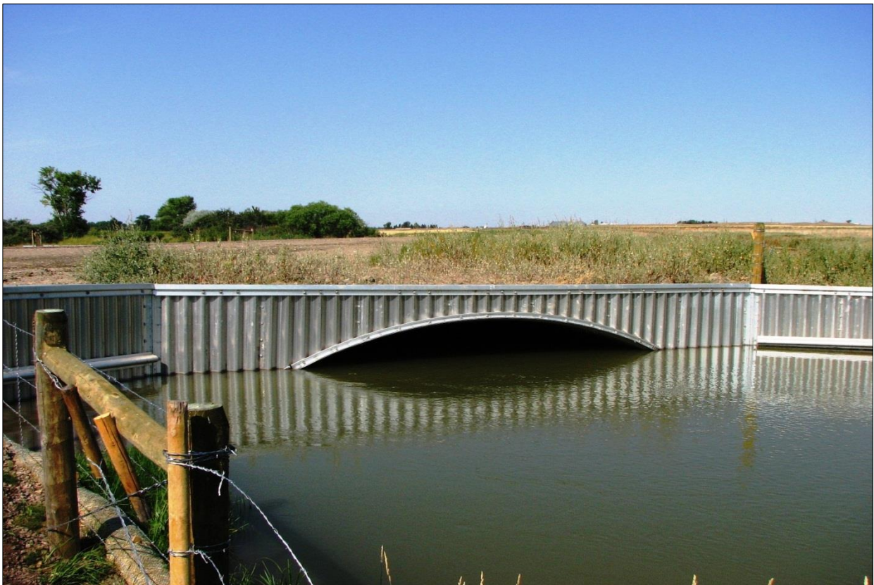
↓ View of culvert outlet.
