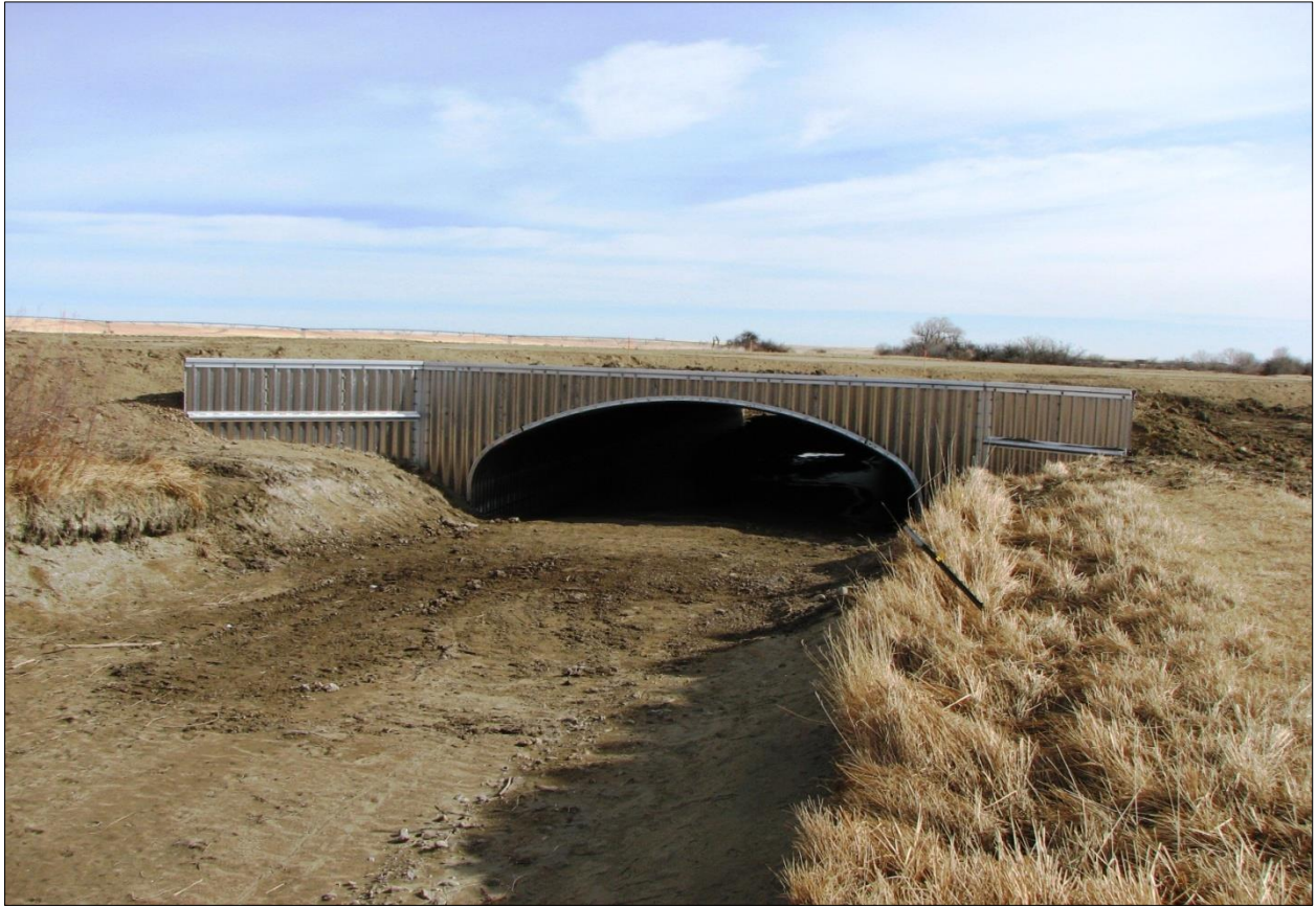
↑↓ Images of completed and covered ABC unit. Above image is the inlet, below image the outlet.
