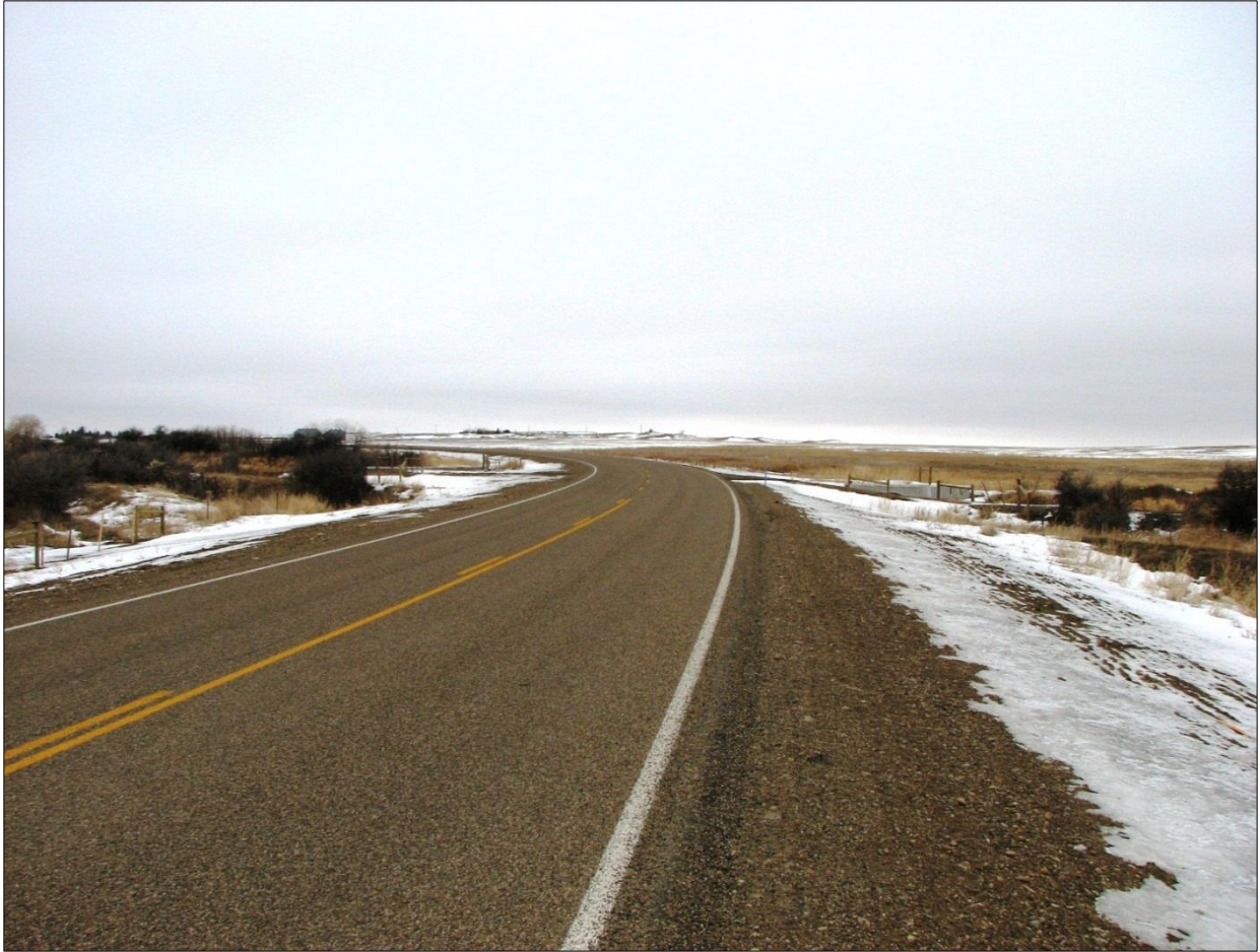
↑ View of completed road bed and culvert as of March 2013; view north.
