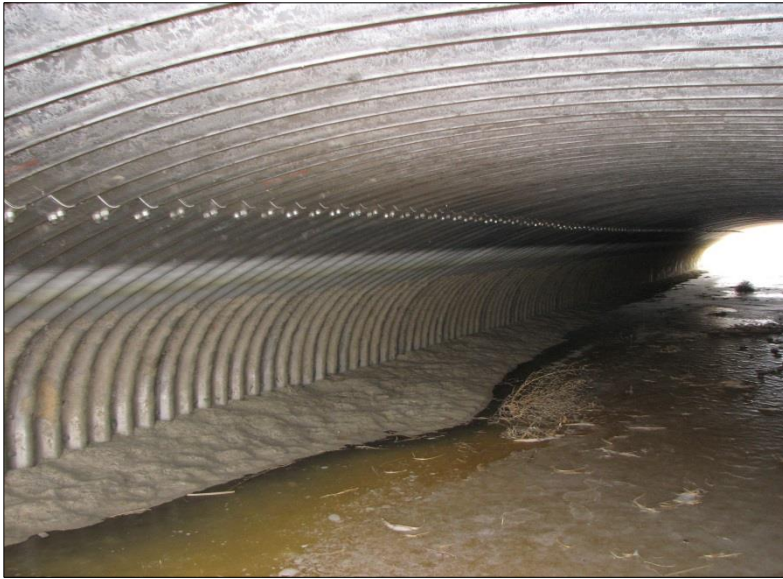
← Interior view of culvert at inlet.
