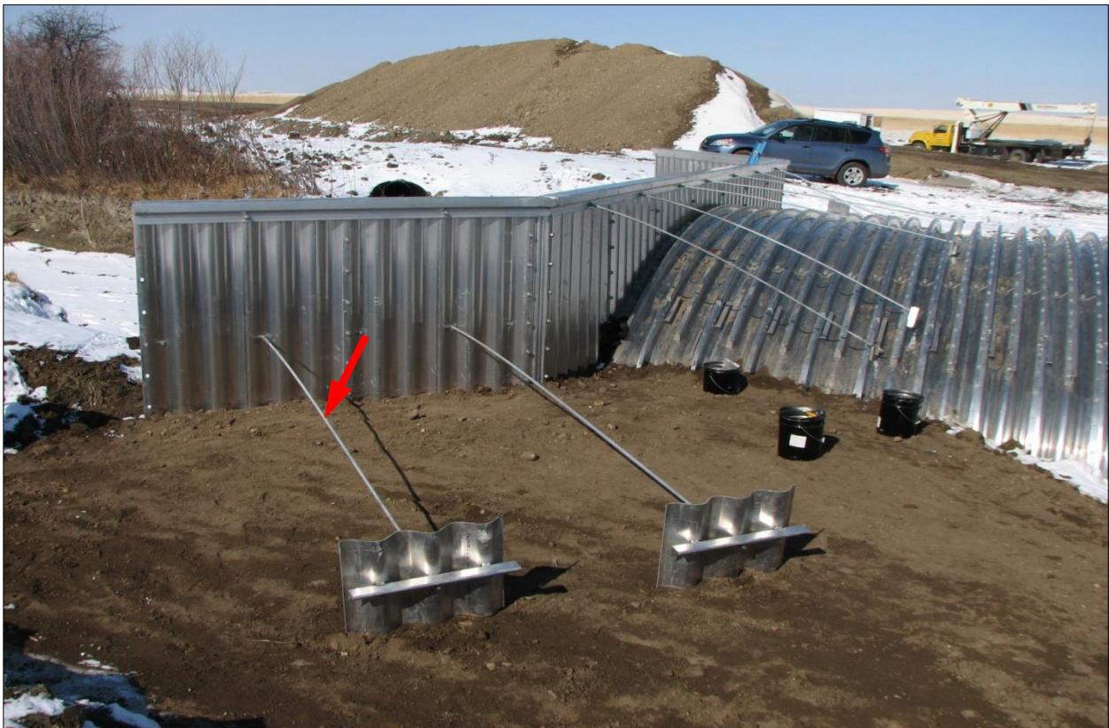
↓ South side of rear inlet wing wall with two attached deadman anchors. The anchor rods (red arrow) have a special attachment to the wingwall wale beam.
