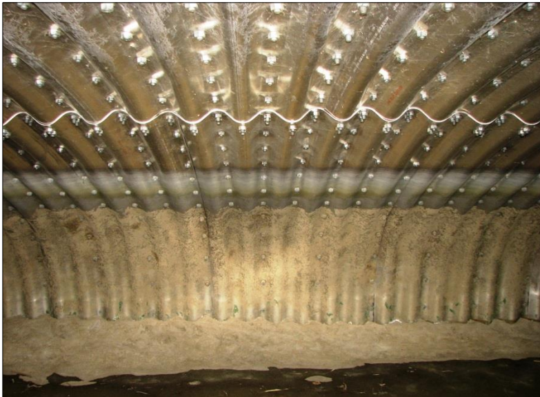
← View of interior sidewall.
