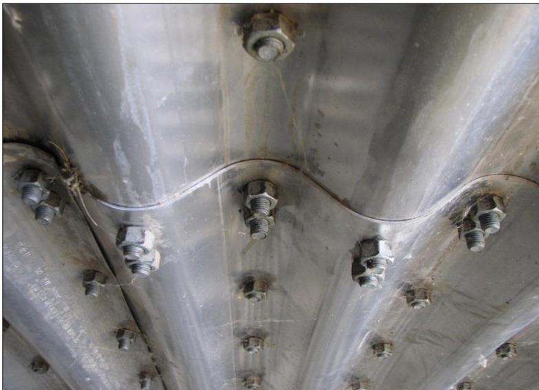
← Close up of plate/rib connections.
