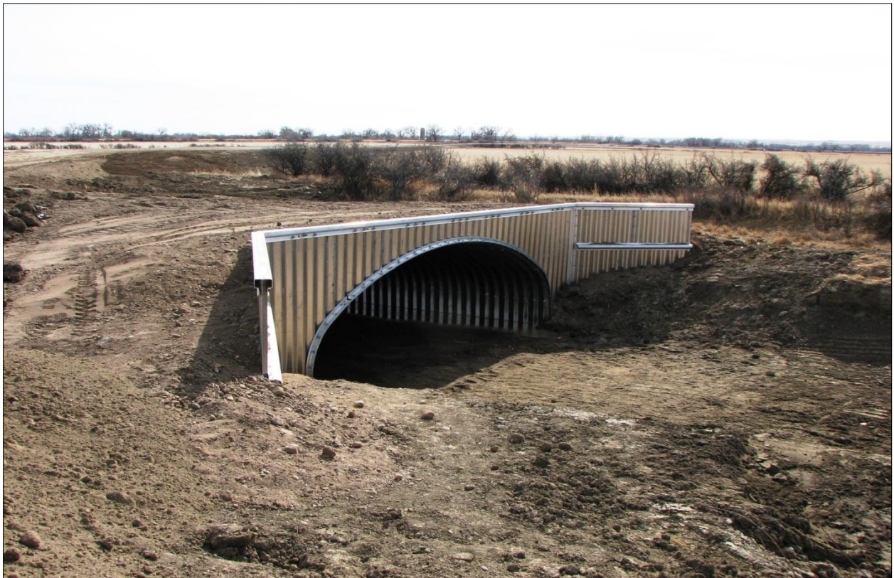
↑↓ Images of completed and covered ABC unit. Above image is the inlet, below image the outlet.
