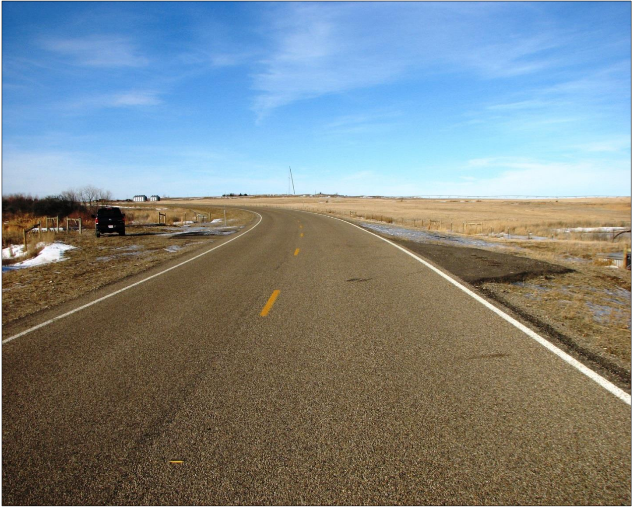
↑ View north. No issues with the roadbed were observed.
