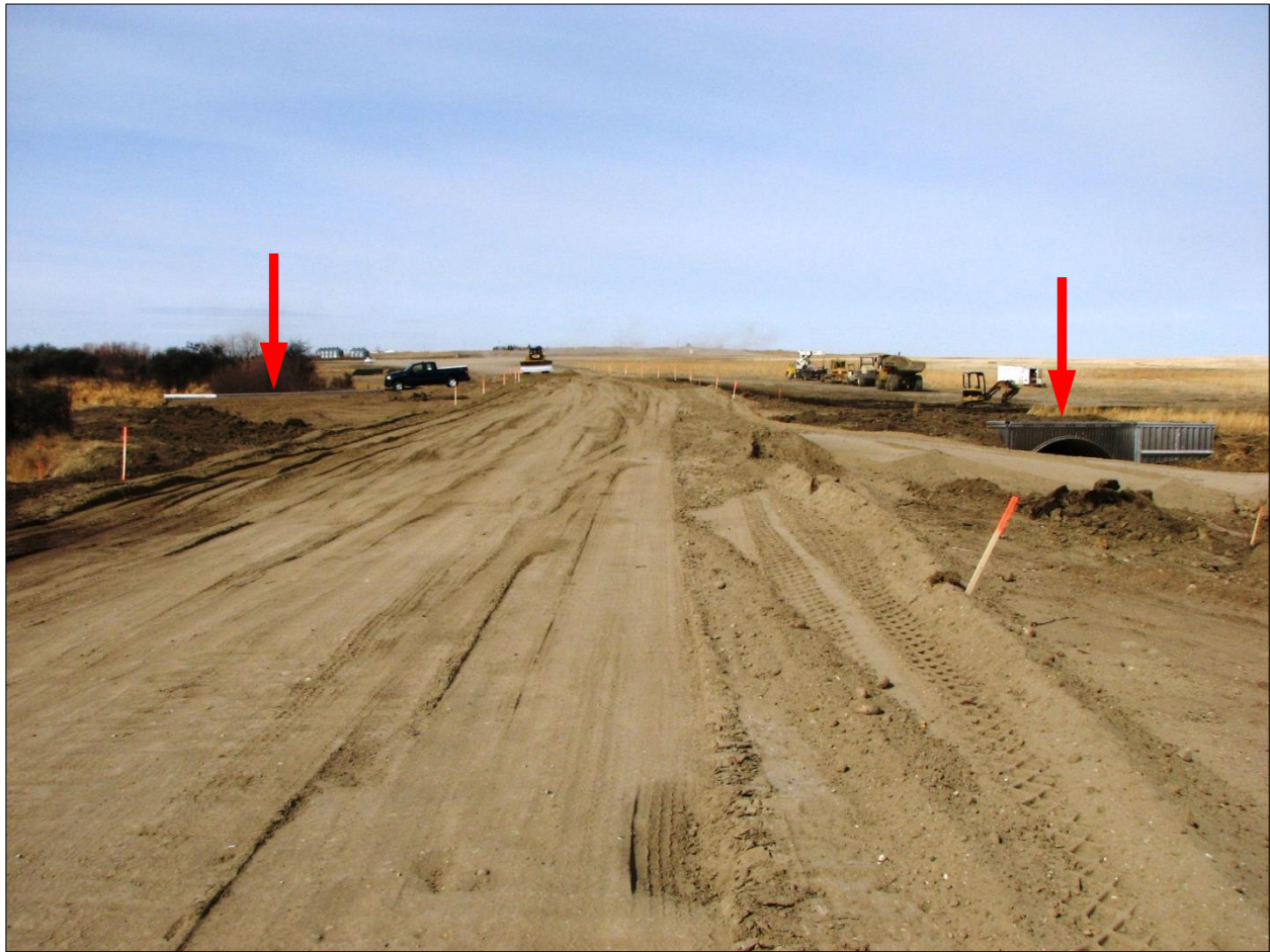
↑ View north. The contractor is beginning to set the base for the roadbed. Red arrows show the location of the culvert inlet/outlet.
