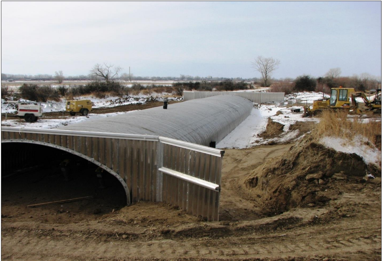
↑ Image of nearly completed outlet head and wingwall, view looking west.
