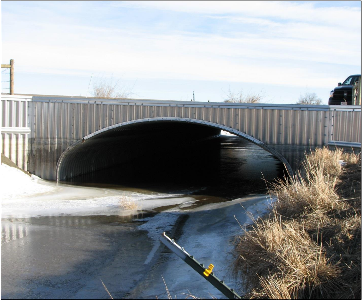
↑ View inlet; west side of culvert.
