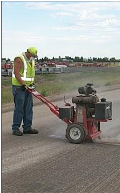
Grinding in process
