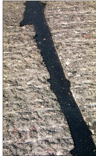
Sealed with Crafc Hot-applied Modified Asphalt Sealant
