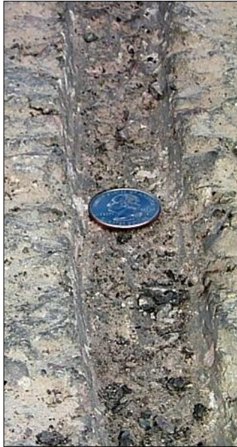
Depth and width of grind
