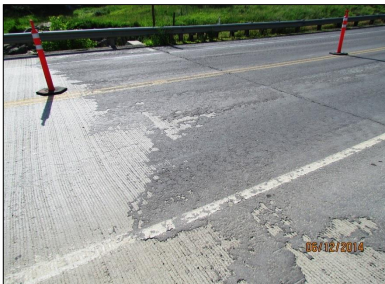
← A previous maintenance patch placed a layer asphalt cement (AC) beyond both approaches of the PCCP deck which will require removal prior to the HFST.
