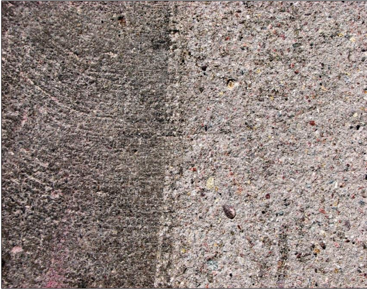
↩️ Several close-up images of the PCCP deck and repair patch after a shot blast past.
