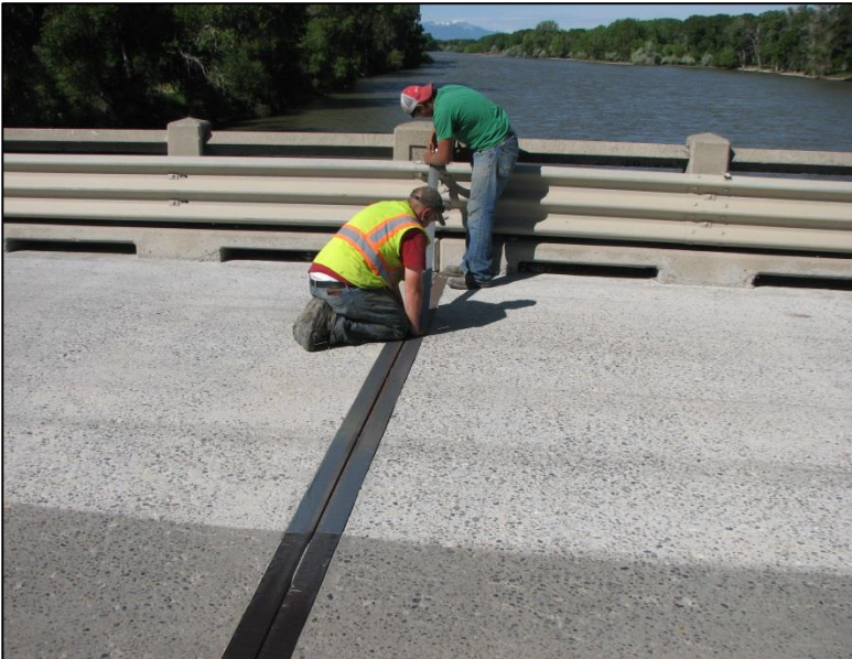
← Bridge expansion joints were covered with duct tape.
