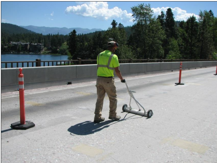
↩️ A magnetic sweeper removed any stray shot from the blasting phase.
