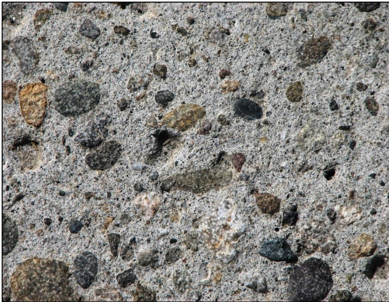
← Representative image of deck surface prepared for HFST treatment.
