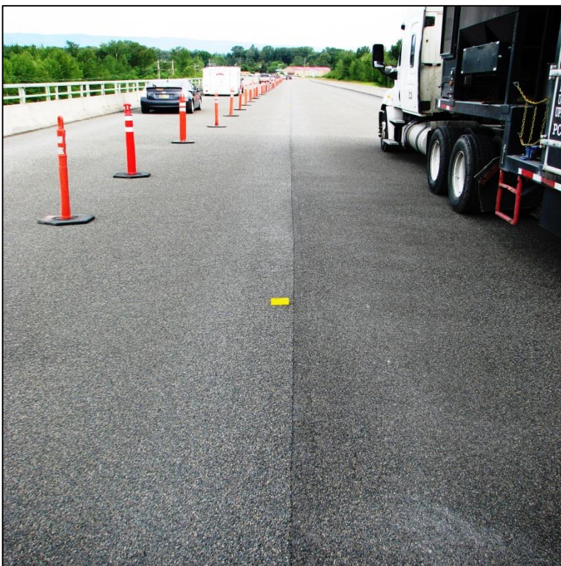
← The eastbound lane (left side of image) has the completed Flexogrid overlay.
