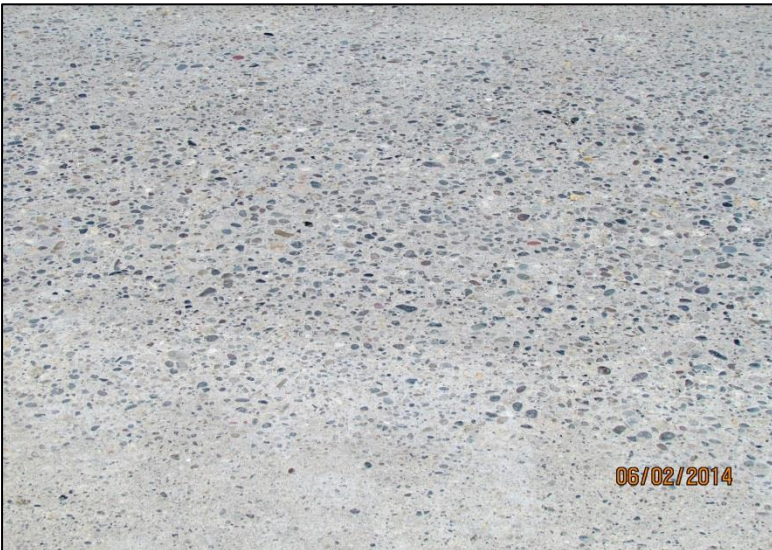
↙ Sample images of average deck surface condition. Most of the deck exhibited polished aggregate, minor popouts and longitudinal cracking.
