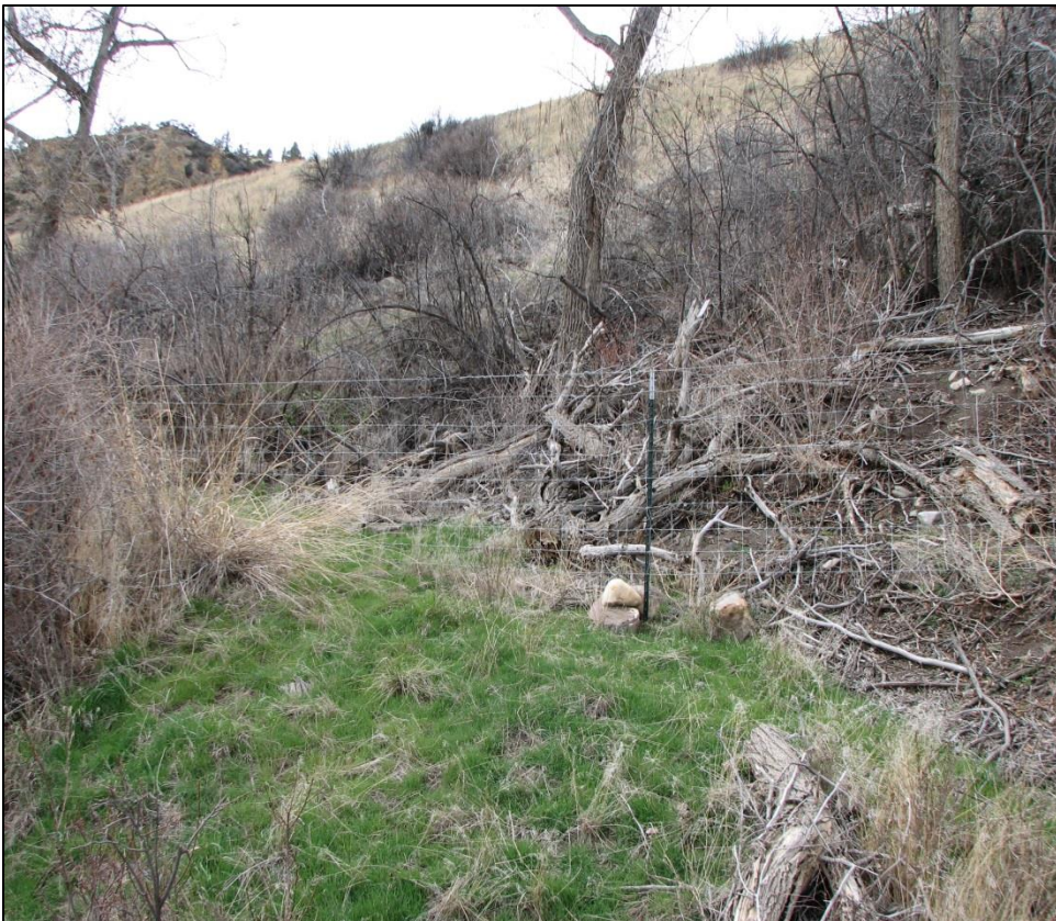
← Image of fence damaged in March 2012 (refer to page 8) in good condition as of April 2014.
