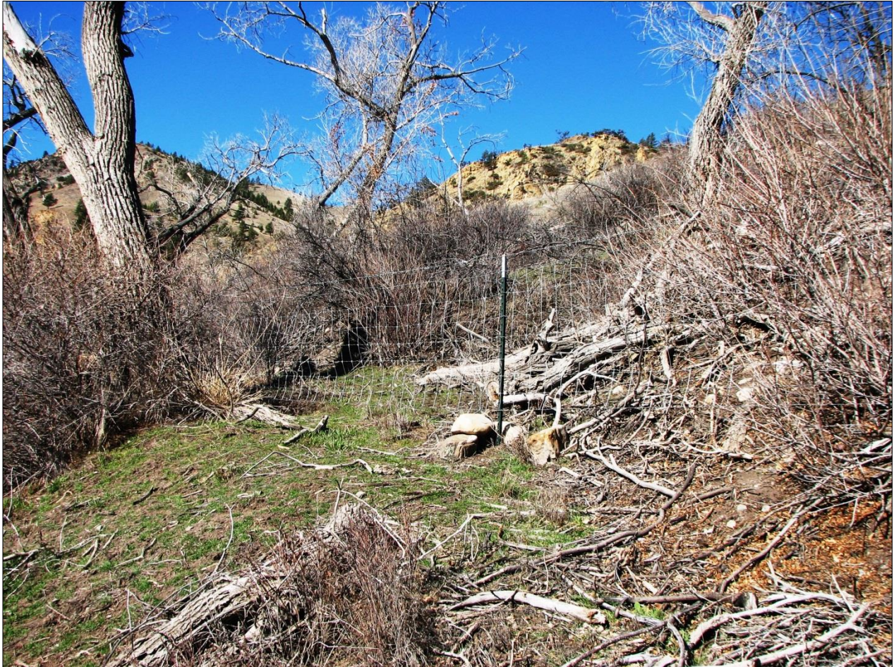
↑ Damaged section as reported in March 2012: No issues to report; repair still intact.
