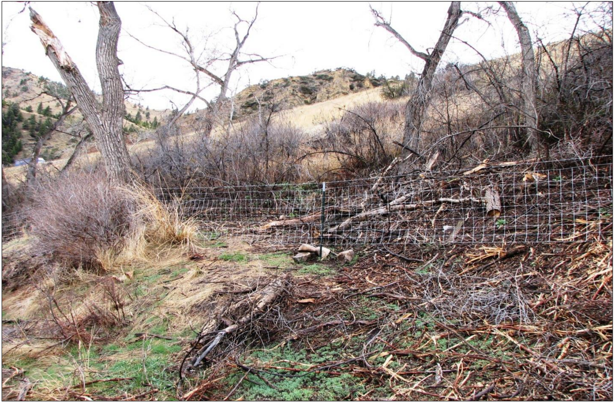
↑ Overview of repaired Stay-Tuff fence section.
