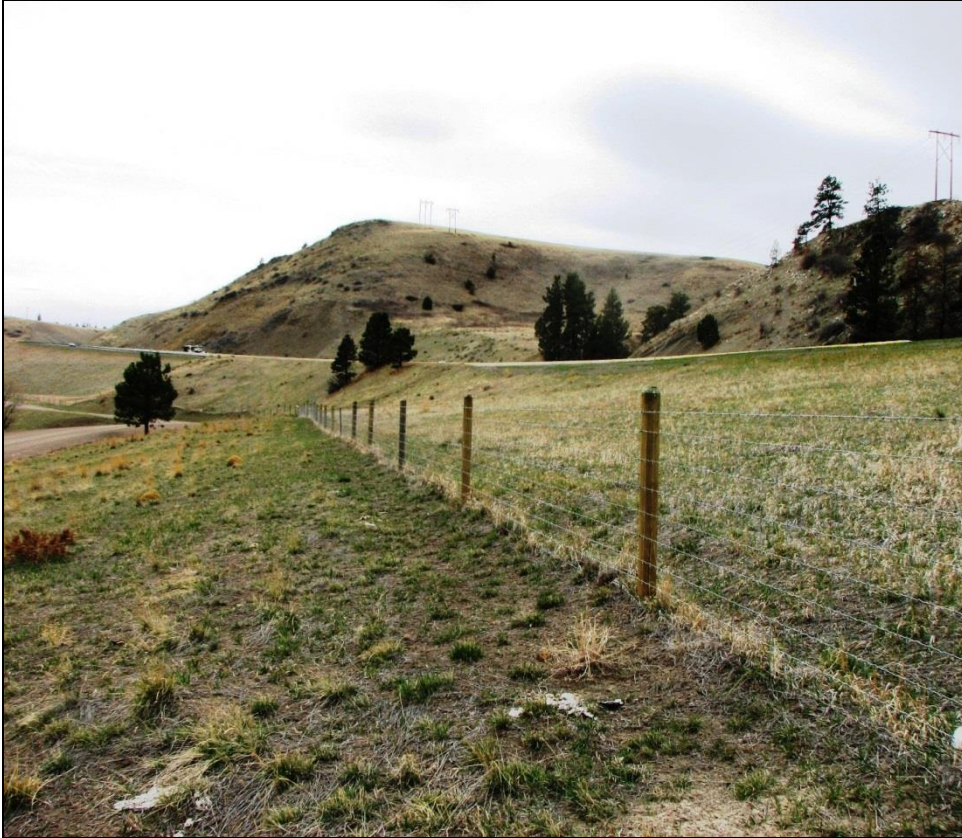
← General condition of the Stay-Tuff fence throughout the project.
