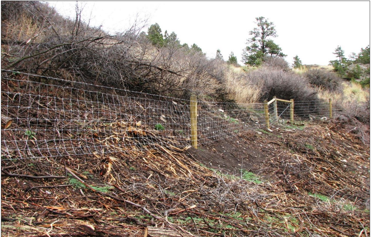
↓ View north of repaired fence.
