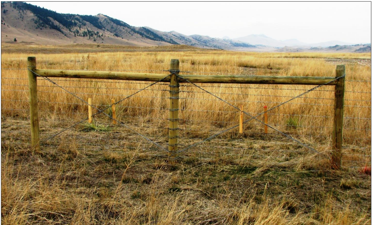
↓ Image of conventional double panel section.
