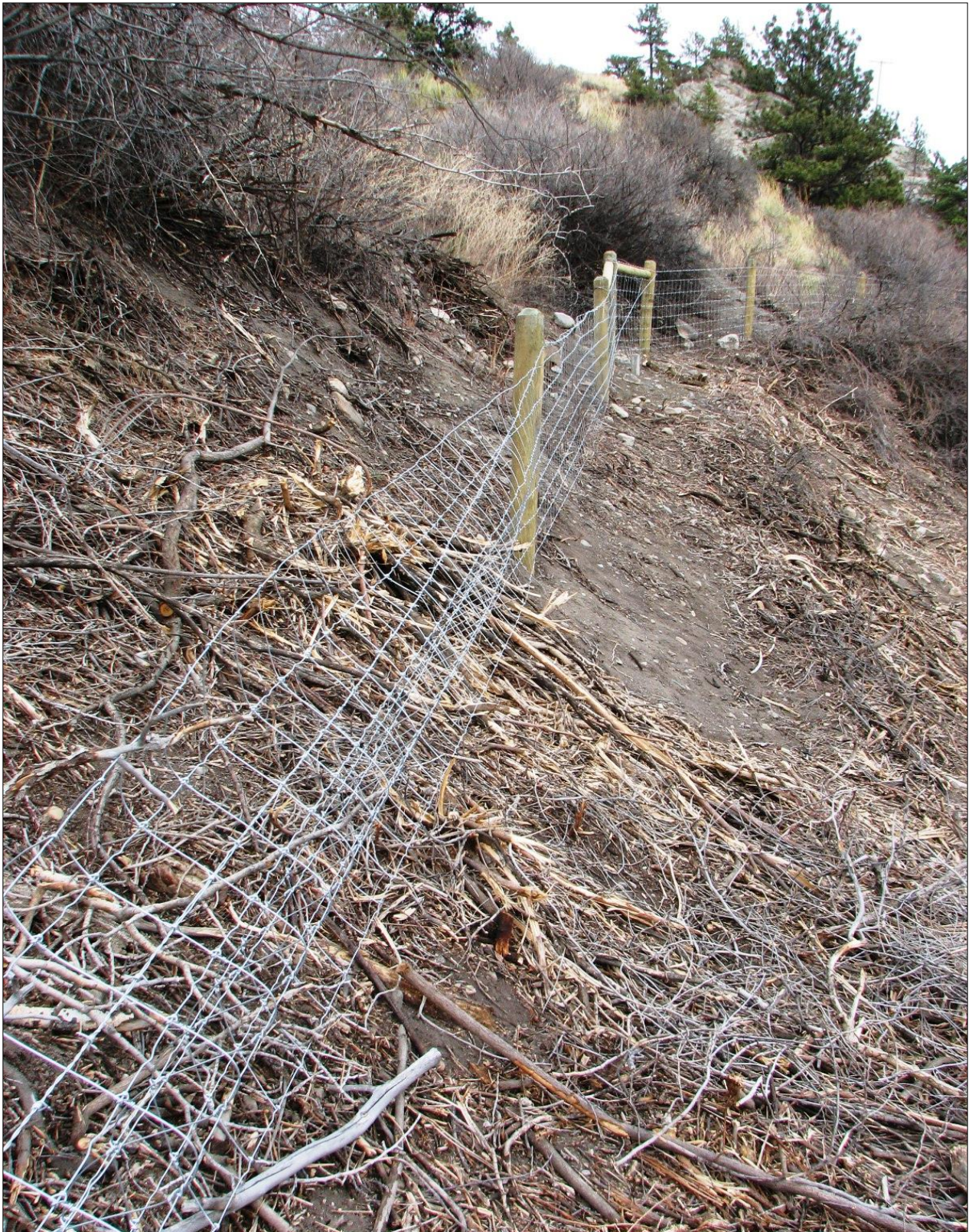
↑ View north of damaged fence section.
