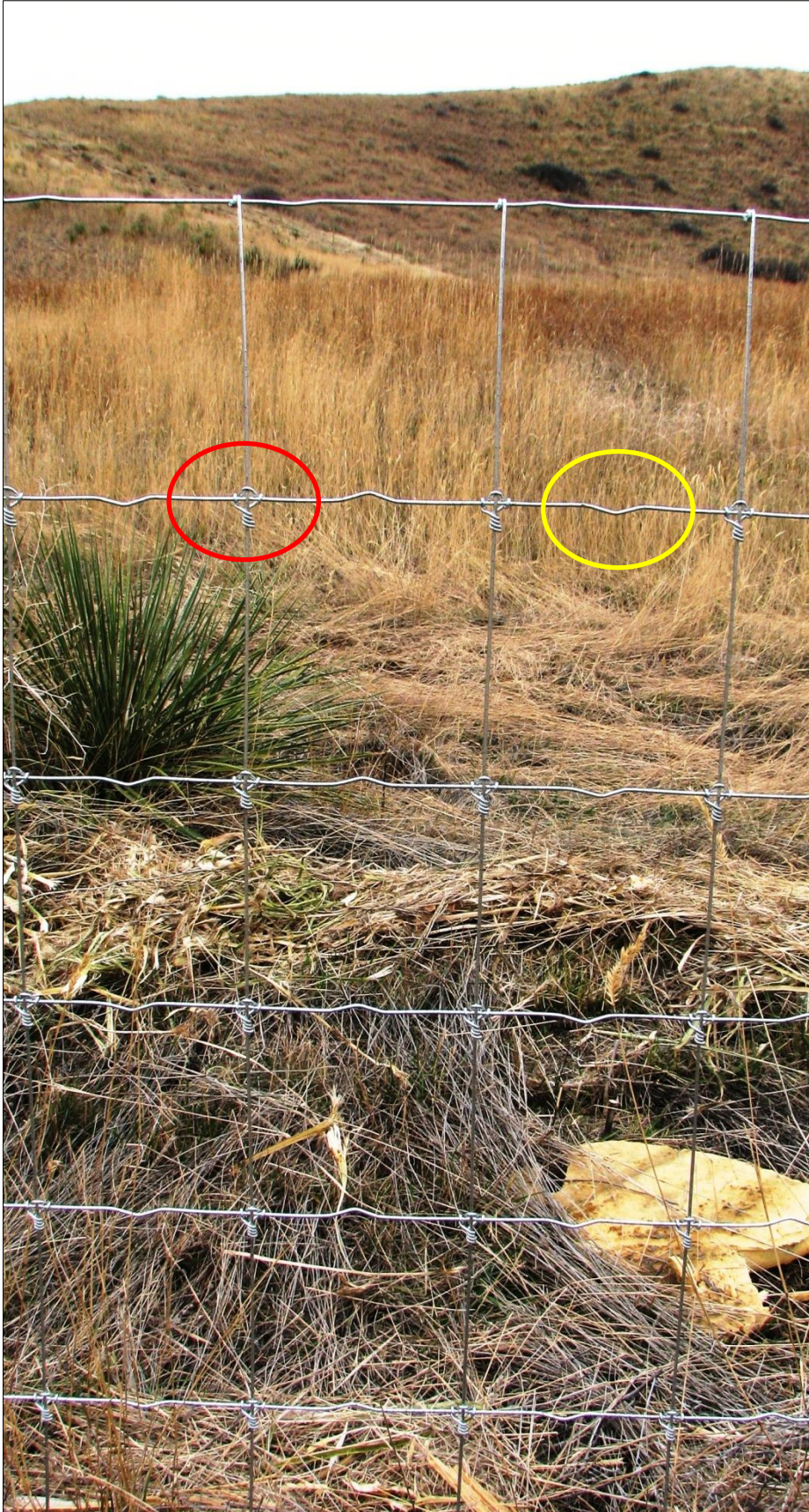
← Image of Stay-Tuff design with the fixed-knot configuration (red circle) and the enhanced vertical crimp (yellow circle).
