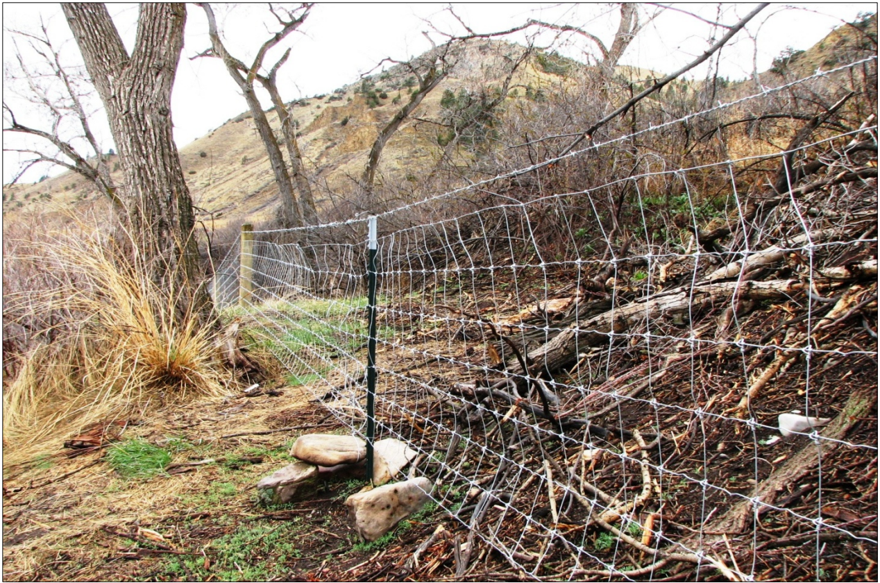
↑ View south of repaired fence.
