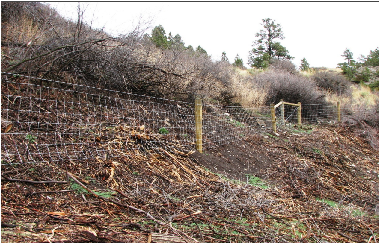
↓ View north of repaired fence.
