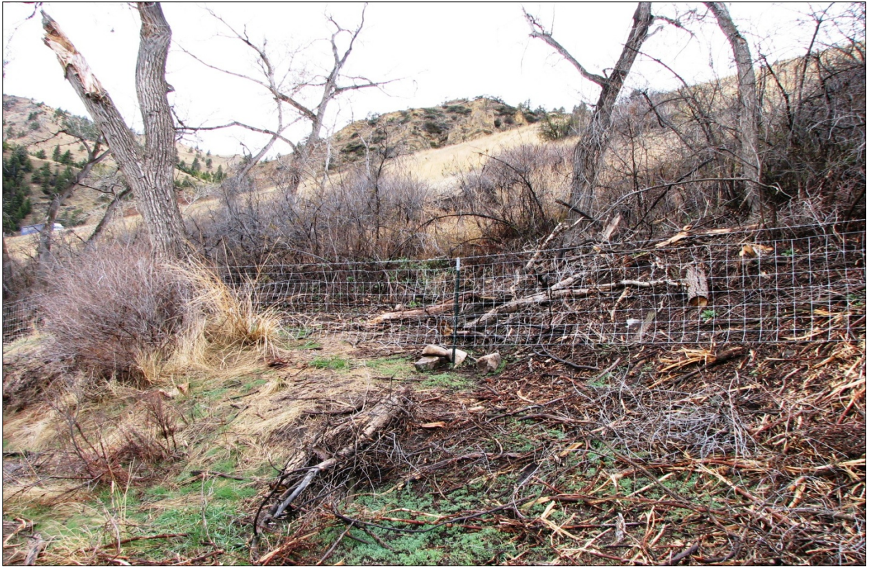
↑ Overview of repaired Stay-Tuff fence section.
