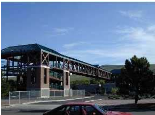
Figure 4-2 Samples of Grade-Separated Structures
