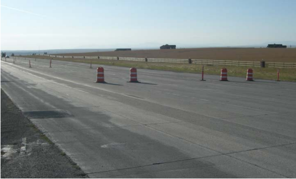
(a) Roadway Construction
