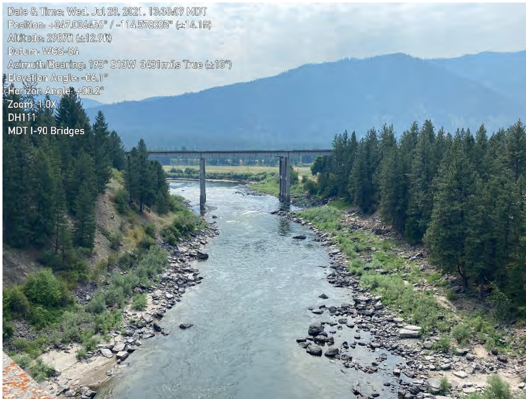
Figure 4: Cyr Bridge facing south.
