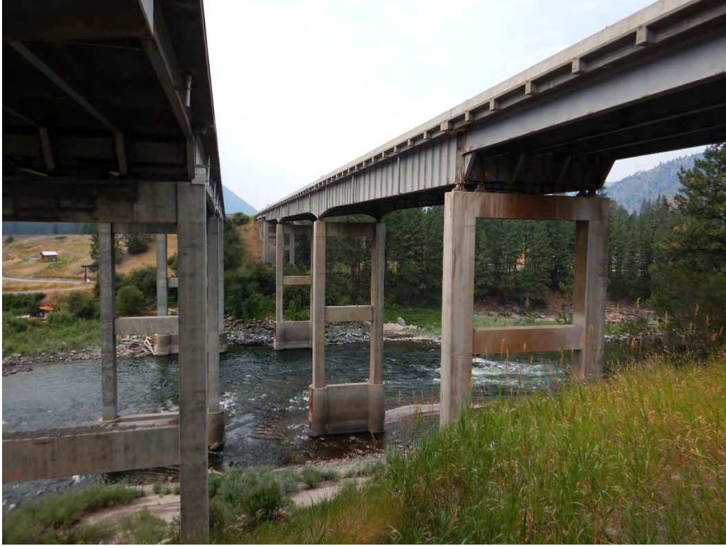
Figure 5: Cyr Bridge facing west.
