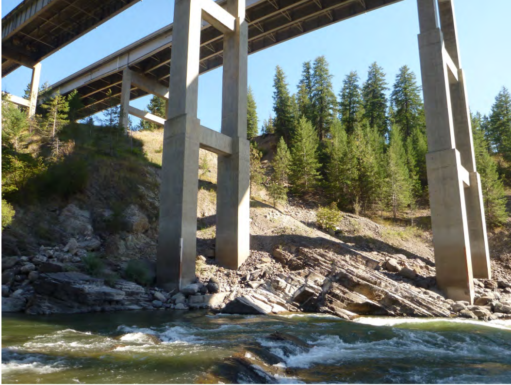
Figure 3: Underside of Clark Fork River Bridge facing southeast.
