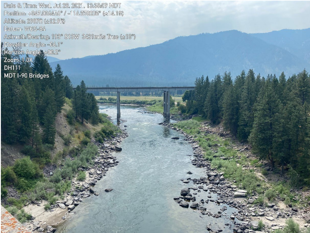
Figure 2: Cyr Bridge facing south.
