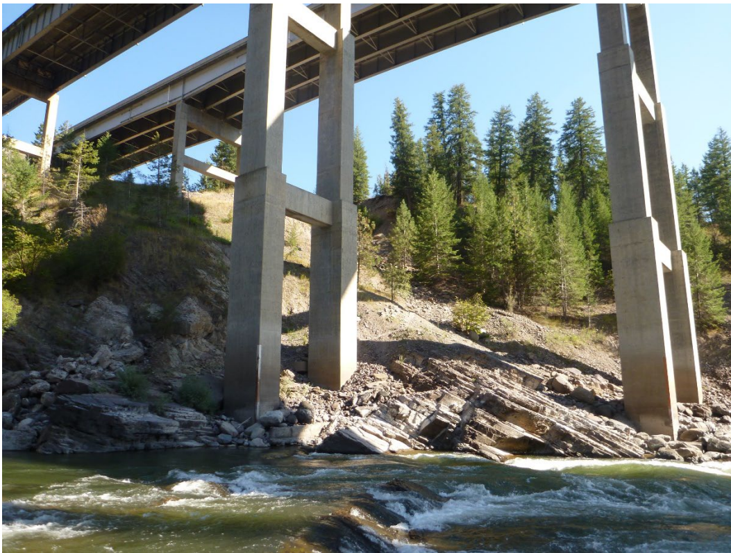
Figure 1: Underside of Clark Fork River Bridge facing southeast.
