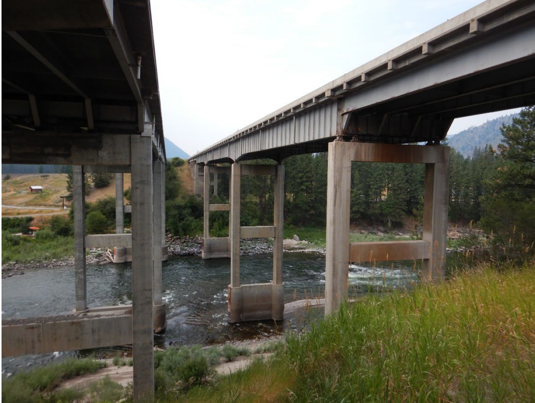
Figure 3: Cyr Bridge facing west.
