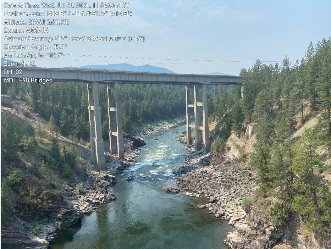
Figure 1: Clark Fork River Bridge facing south.
