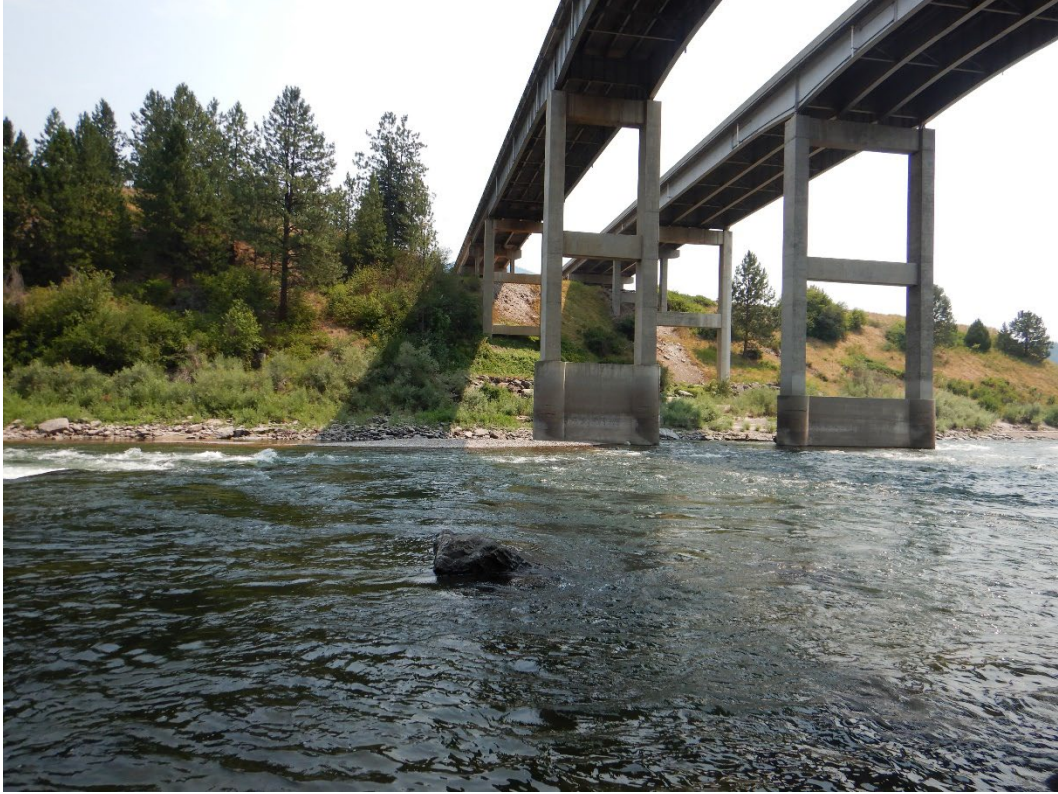
Figure 4: Underside of Cyr Bridge facing east.
