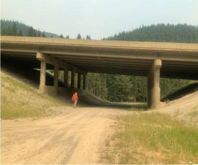
Local Access Bridge @ RP 1.9
