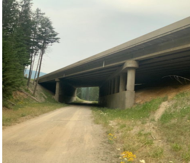
Local Access Bridge @ RP 5.2
