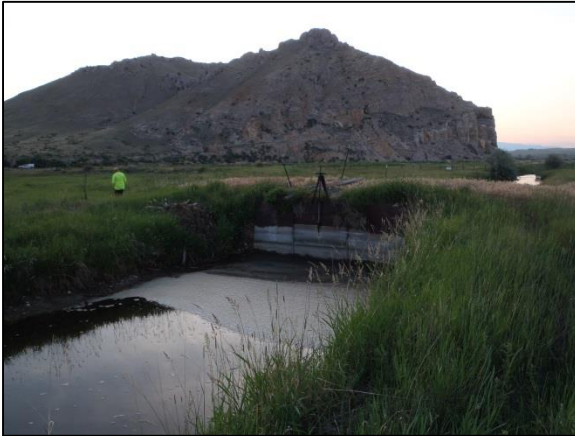
Photo 1. Co-op Ditch headgate (looking northeast)
