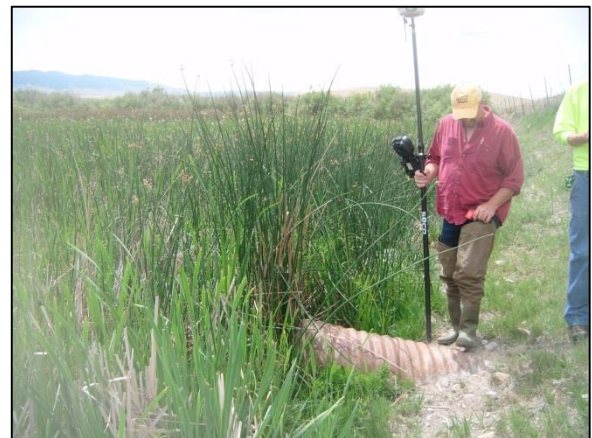
Photo 16. Southern most culvert draining to the east under Highway 41 to wetlands
