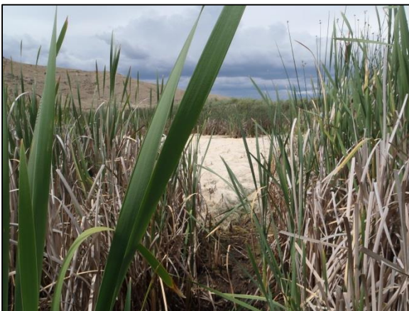
Photo 15. Southernmost culvert channel of recently dried up thermal spring/oxbow draining to the east under Highway 41
