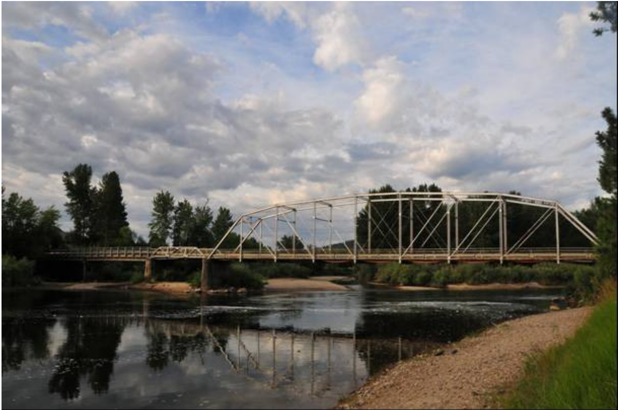
Photo MT_MissoulaCounty_MaclayBridge_0001 (1 of 9) - Maclay Bridge: overview looking south.
