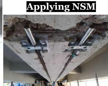
Strengthening of the Buhung Bridge using CFRP NSM bar , Gyeonggi-do, South Korea (Lee et al. 2018)
