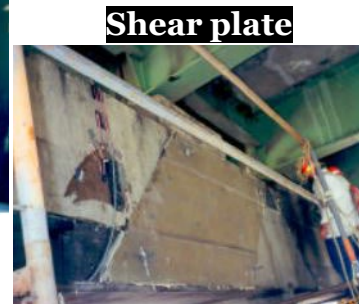
Repair of cracked cap beam using bonded FRP plate , East Church Street bridge, Over State Route 17 City of Elmira, New York (Hag-elsafi et al. 2002)
