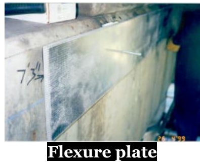
Repair of cracked cap beam using bonded FRP plate , East Church Street bridge, Over State Route 17 City of Elmira, New York (Hag-elsafi et al. 2002)
