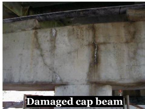
Repair of cracked cap beam using bonded FRP plate , East Church Street bridge, Over State Route 17 City of Elmira, New York (Hag-elsafi et al. 2002)
