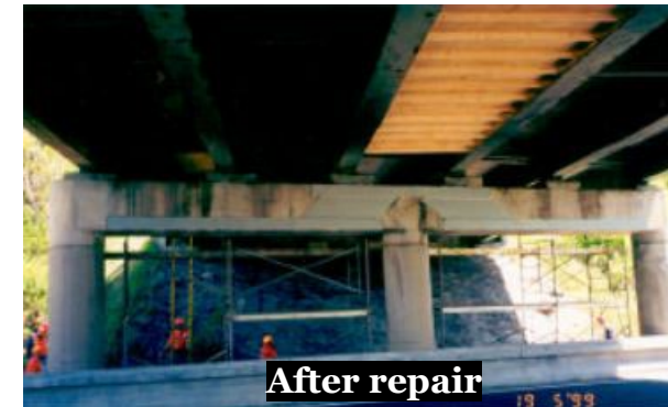
Repair of cracked cap beam using bonded FRP plate , East Church Street bridge, Over State Route 17 City of Elmira, New York (Hag-elsafi et al. 2002)
