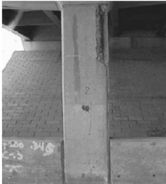
Corrosion damage
