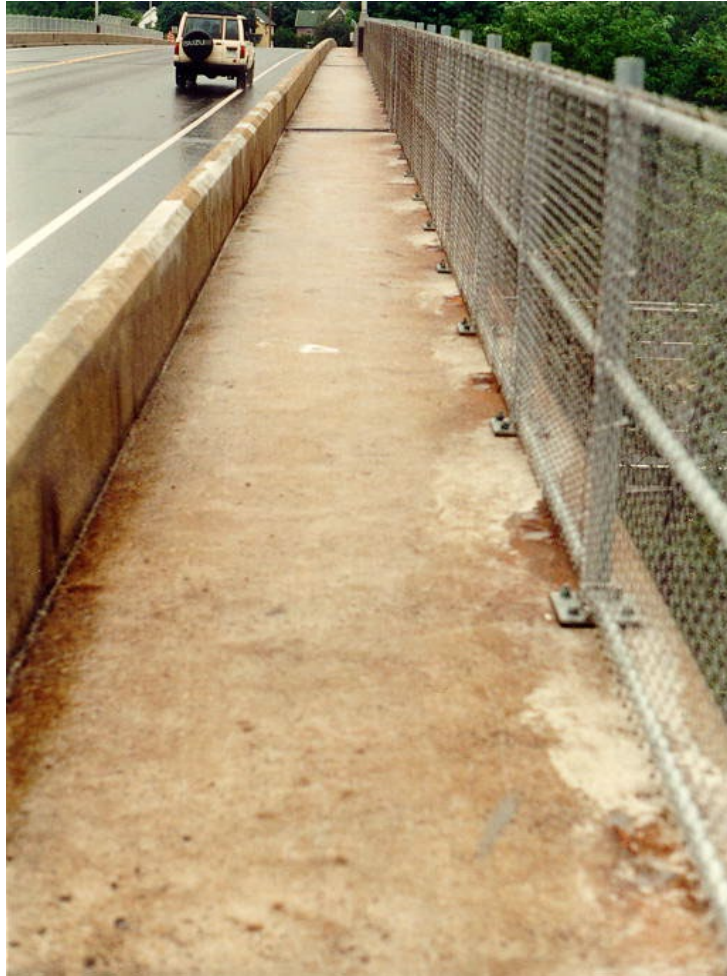
Figure 3.2.7-1 Concrete Sidewalk with Pedestrian Fence and Traffic Divider.
