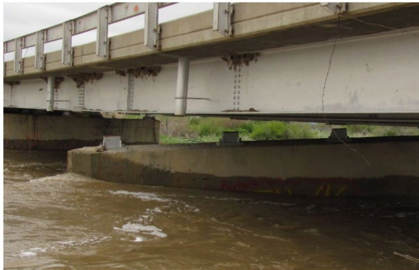
Figure 3.5.2-1 Pier Settlement due to Undermining
