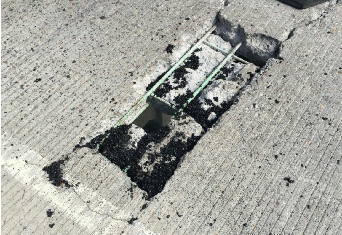
Figure 4 – Holes in Bridge Deck. Note the longitudinal jump cracks that create the rectangular “island” of concrete. The “island” continued to crack until full depth chunk or “island” fell out, creating the hole.
