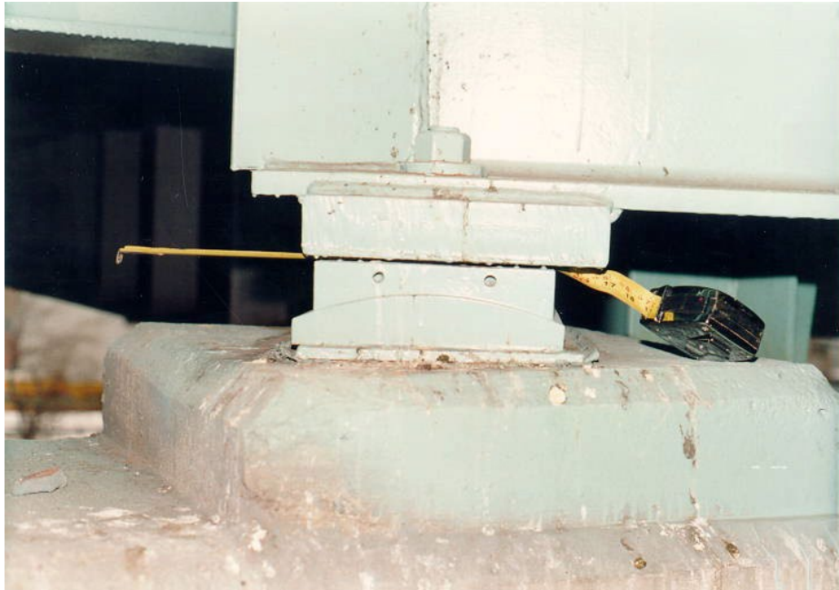
Figure 3.3.1-10 Bronze Sliding Plate Bearing with a Gap Between the Sole Plate and the Sliding Plate.
