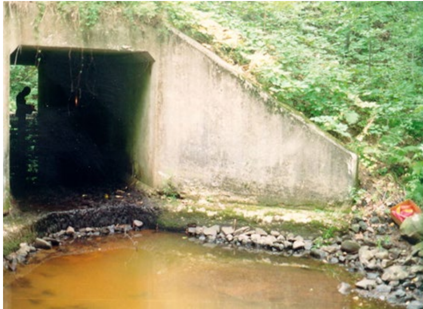
Figure 3.6.3-1 Cast-In-Place Concrete Culvert with Erosion at the Outlet.
