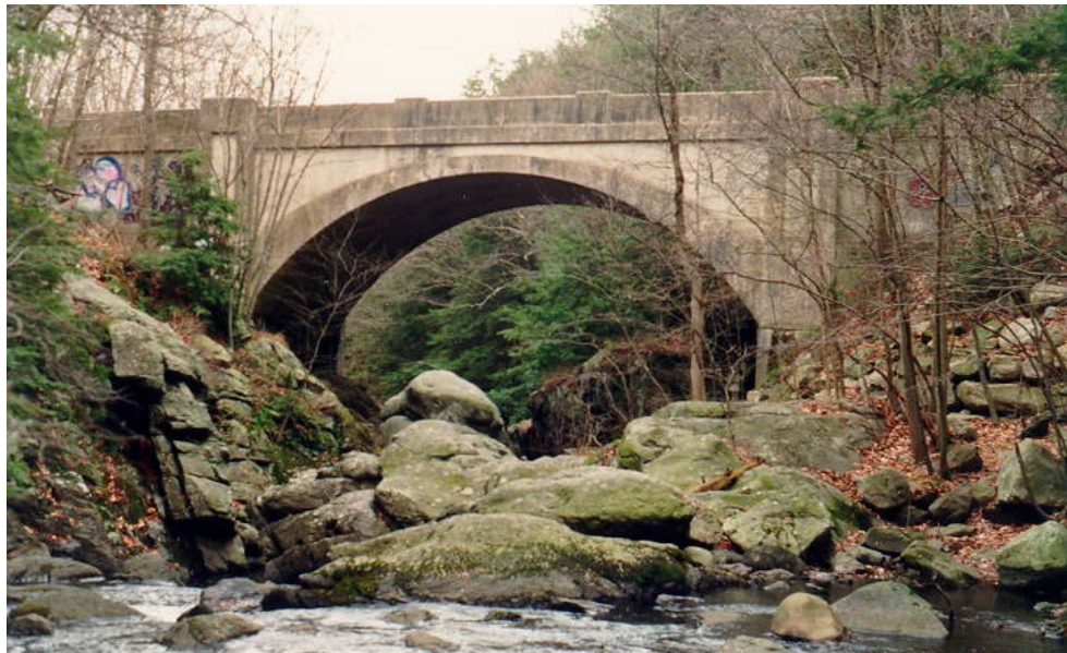
Figure 3.3.5-1 A Closed Spandrel Reinforced Concrete Arch Bridge
