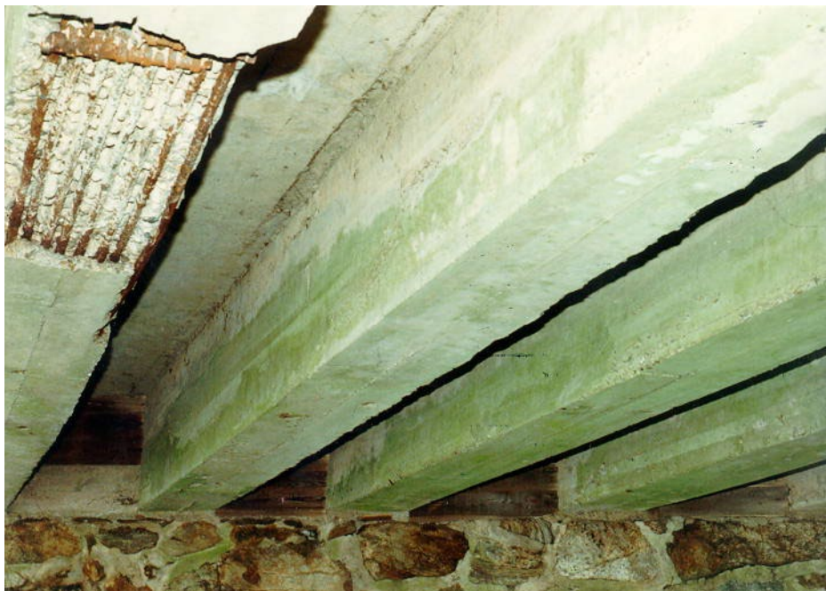
Figure 3.3.4-1 Concrete T-Beams with Large Spalls Exposing the Bottom Layer of Reinforcing Steel
