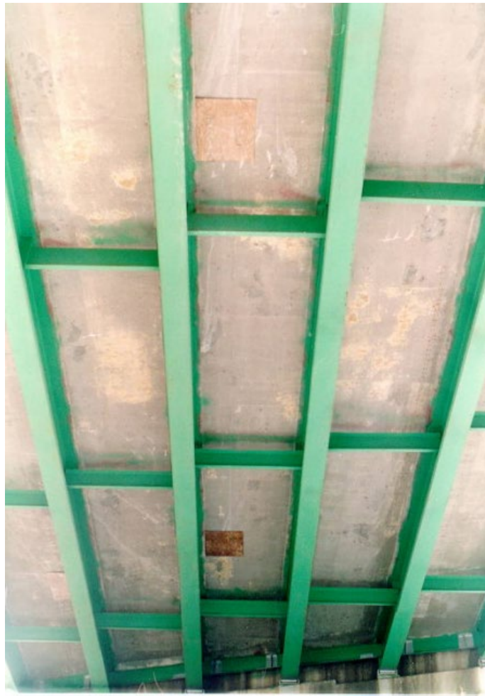
Figure 3.2.2-1 Typical Underside of Concrete Deck. Note Cracking with Efflorescence and Formwork Remaining from Full Depth Patching.
