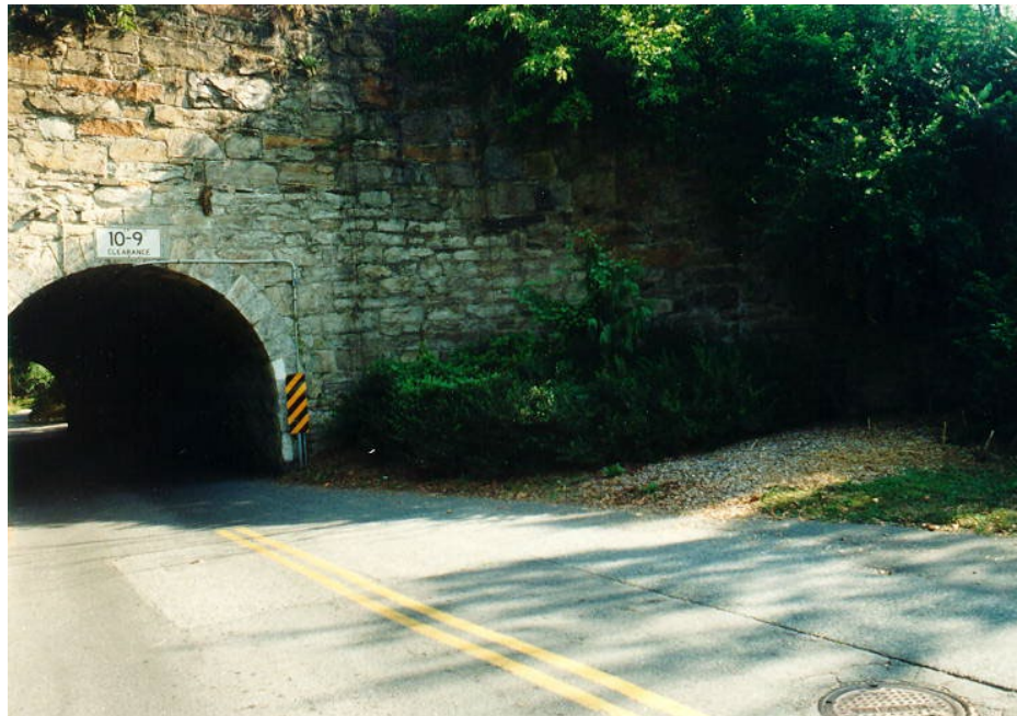
Figure 3.3.13-1 Stone Masonry Arch and Spandrel Wall
