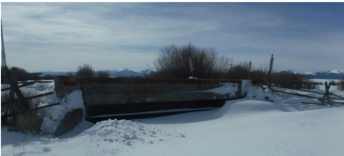
Figure 2.6.7-2 A follow-up inspection is required to check the condition of the wingwalls, abutments, and part of the exterior girder.
