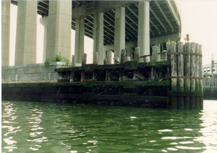
Figure 3.5.1-1 Timber Fender System with Navigation Lights.
