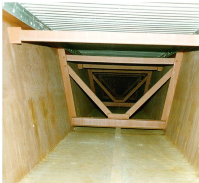
Figure 3.3.10-2 Inside Steel Box Girder.
