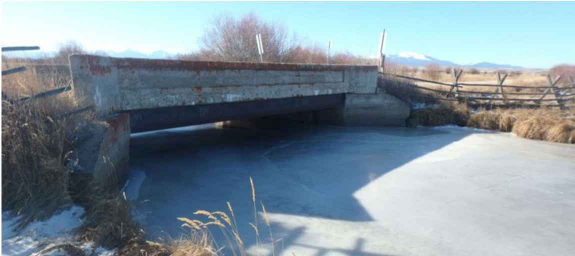
Figure 2.6.7-3 A follow-up inspection is required to check the condition of the bottom of the abutments and to check for scour.
