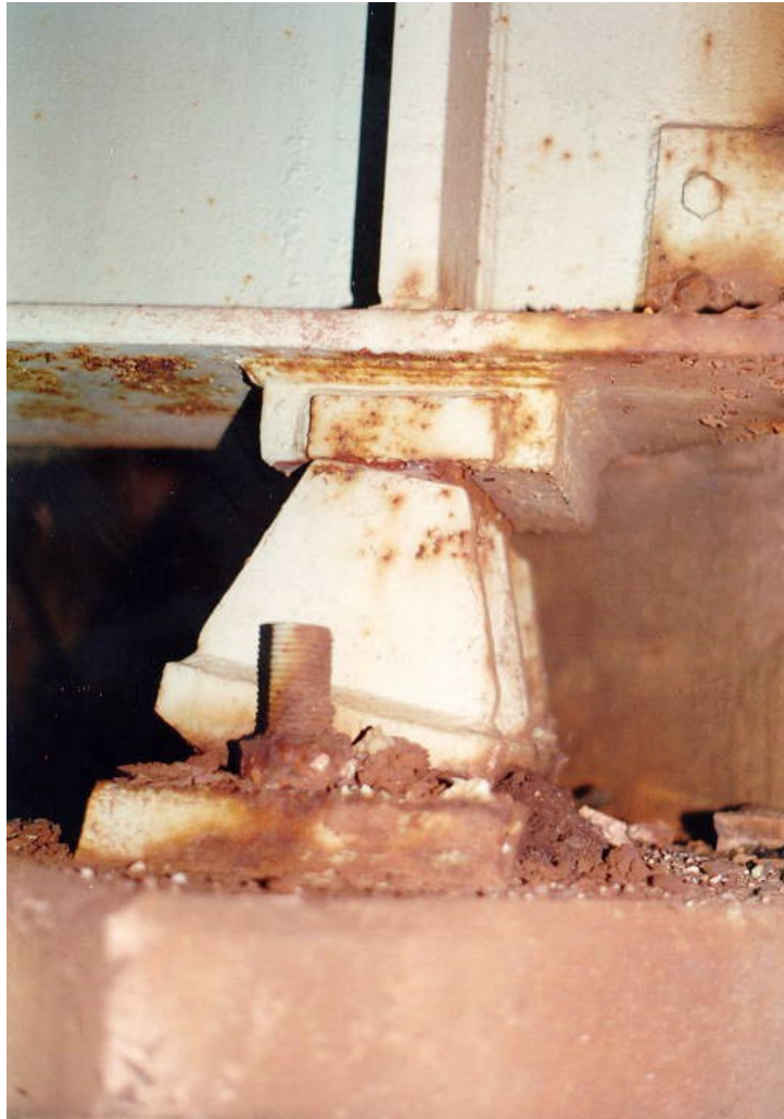
Figure 3.3.1-9 Over Extended Rocker Bearing.
