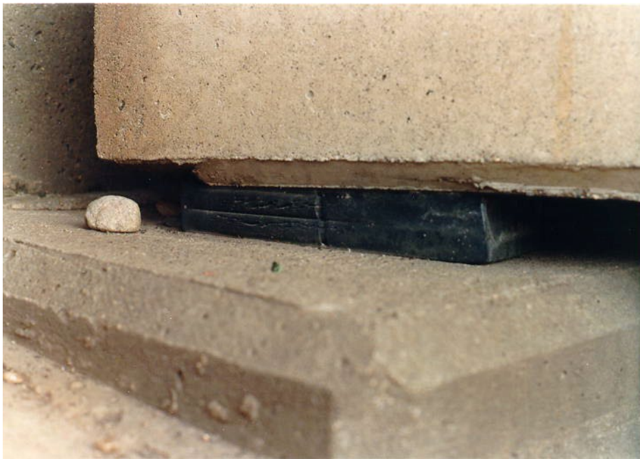
Figure 3.3.1-13 Elastomeric Bearing. Note the Non-parallel Bearing Surfaces Causing Bulging and Cracking at the Rear of the Elastomeric Bearing Pad.
