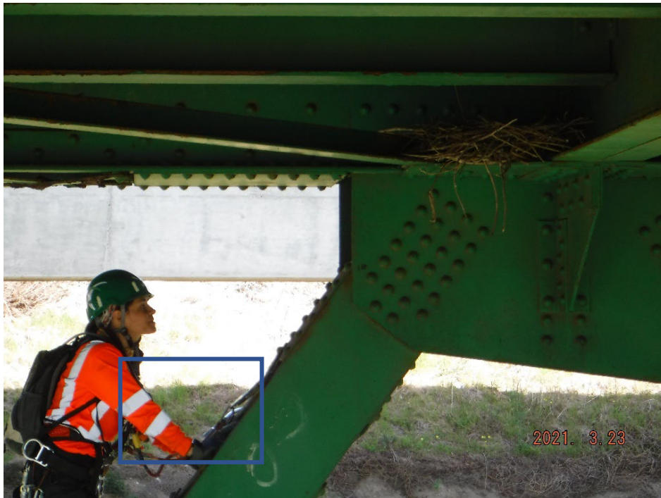
Figure 3.7.2-2 Bridge Inspector Using Climbing Techniques (Level B Climbing)
