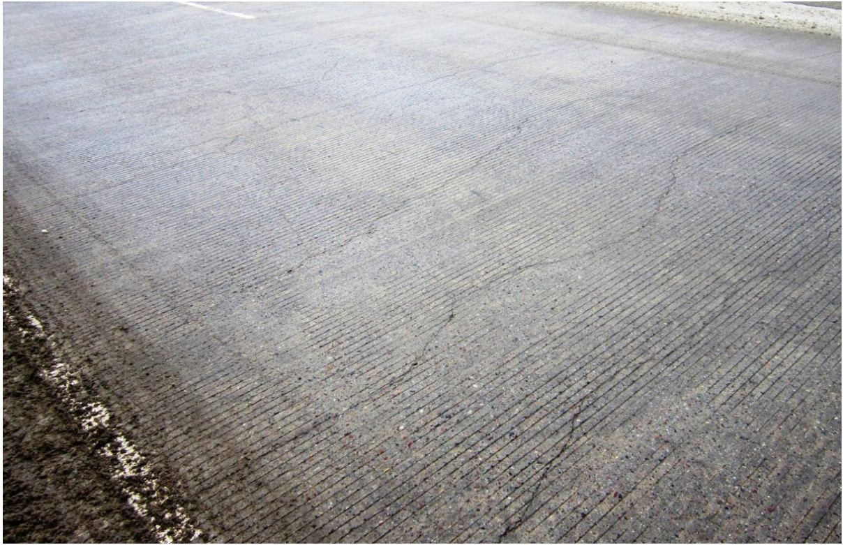
Figure 2. Transverse Cracks in Bridge Deck
