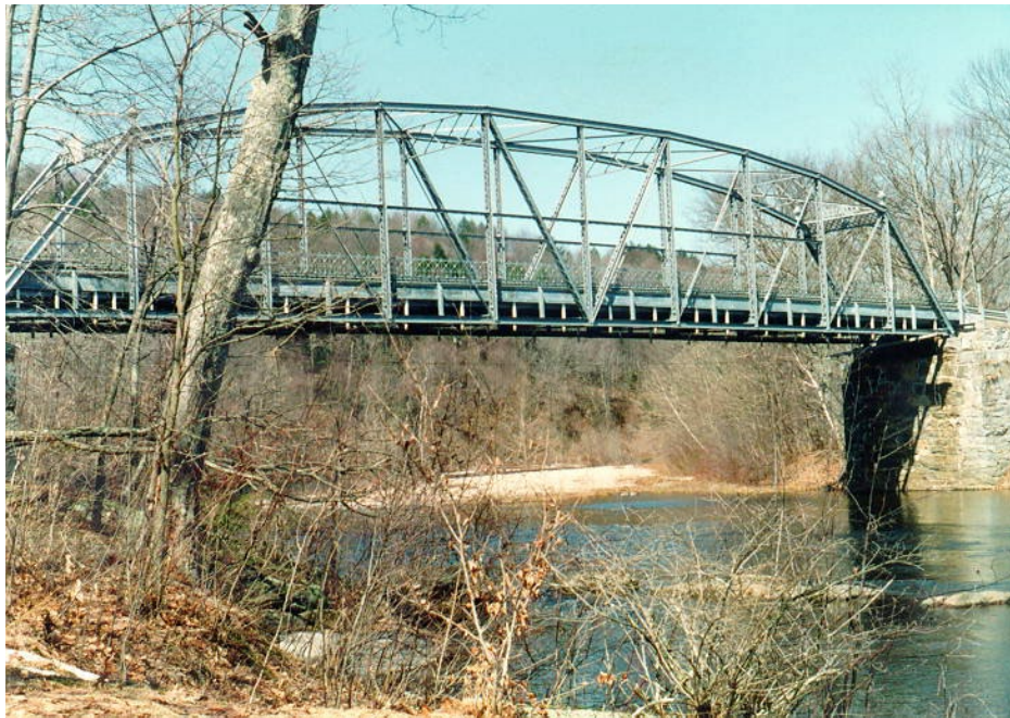
Figure 3.3.11-1 Historic Steel Through Truss Bridge.
