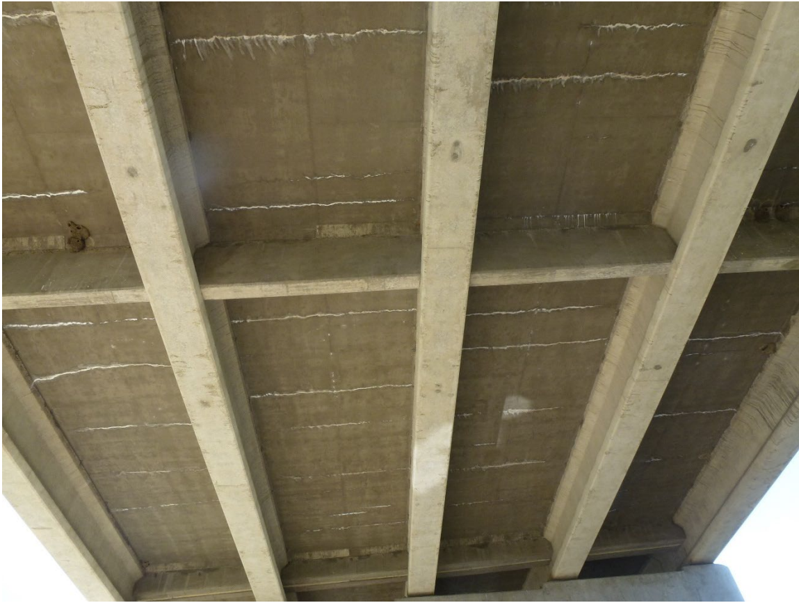
Figure 7. When to not use the transverse pattern cracking defect. Use the deck cracking defect only. Transverse cracking is present but sporadic. Note the wide crack spacing, the lack of staining, and no longitudinal jump cracks. All efflorescence is white.
