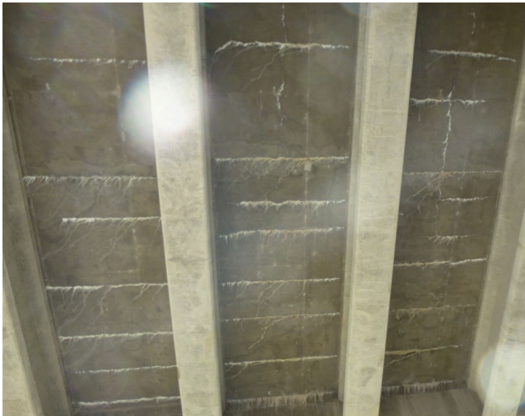
Figure 10. Example of Condition State 3. Tight spacing, jump cracks, some light staining from leakage, and some gray efflorescence.
