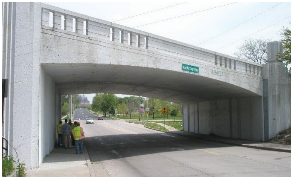
Figure 3.3.5-1 A Closed Spandrel Reinforced Concrete Arch Bridge
