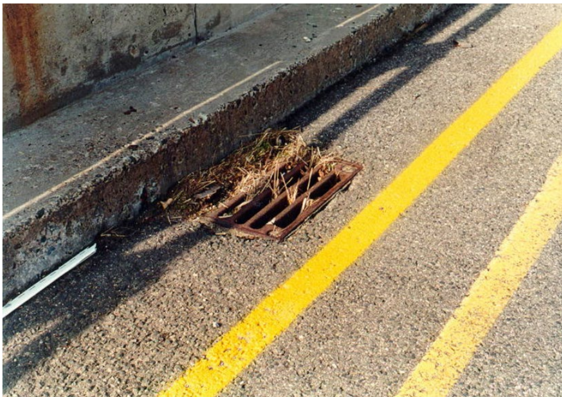
Figure 3.2.5-2 Typical Concrete Curb with Safety Walk
