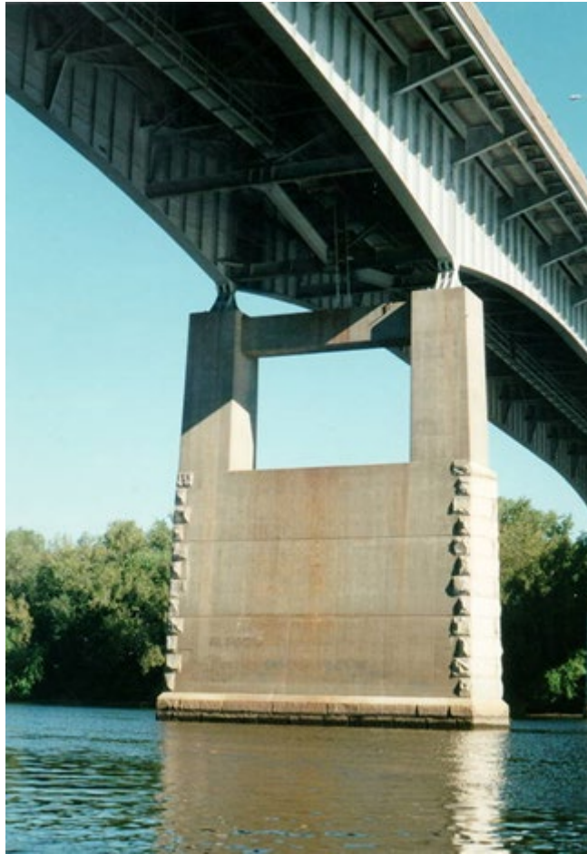
Figure 3.4.1-2 Tall Concrete Pier with Decorative Stone Masonry Facing
