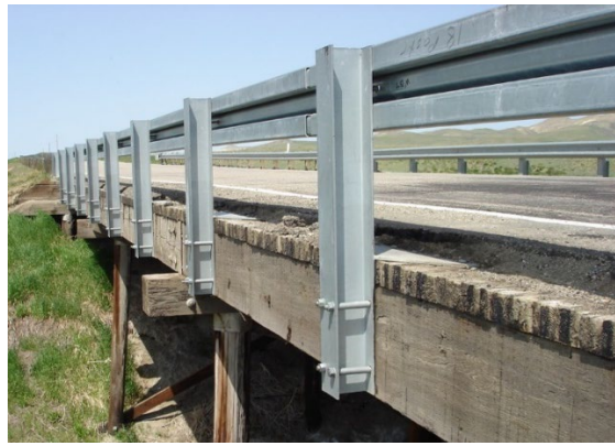
Figure 3.1.4-3 Any Rail Attached to Timber: Code 0 (NOT Crash Tested)
