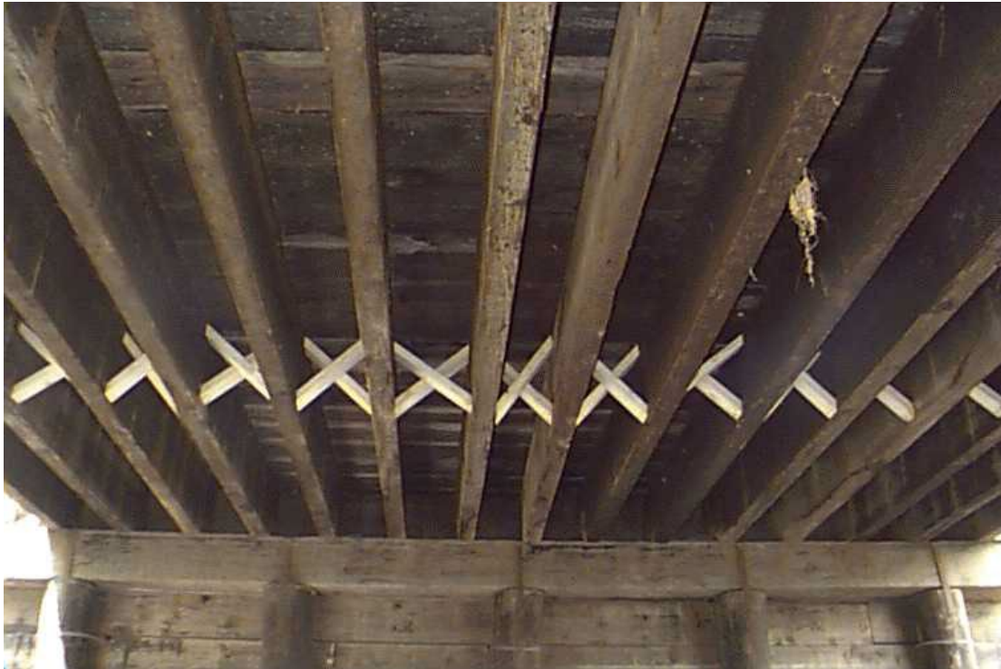
Figure 3.3.12-2 Underside View of a Solid Sawn Multi-Beam Timber Bridge.
