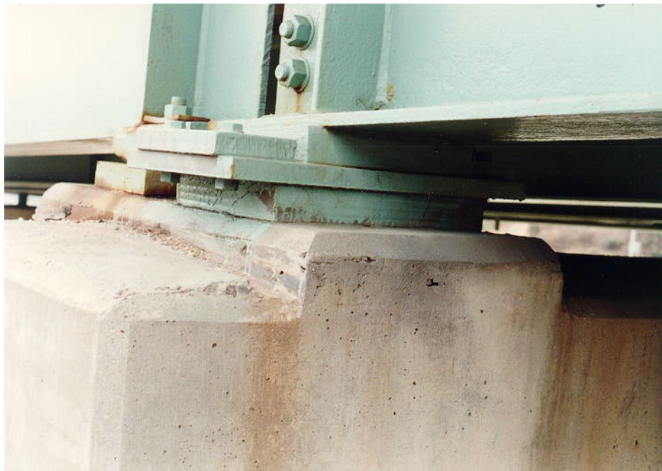
Figure 3.3.1-11 Retrofit Detail. Elastomeric Bearing Installed to Replace Bronze Sliding Plate Bearing.
