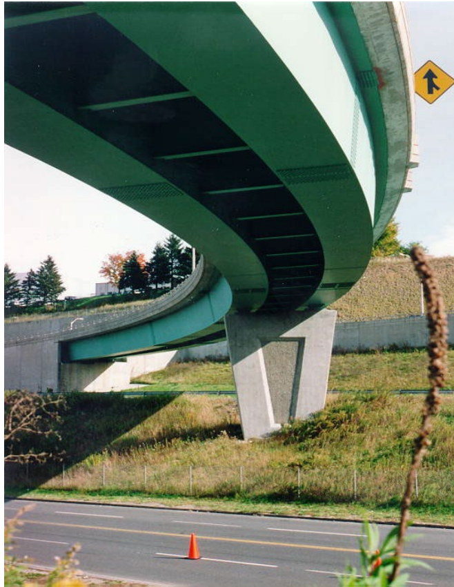
Figure 3.3.10-1 Curved Steel Box Girder Bridge.
