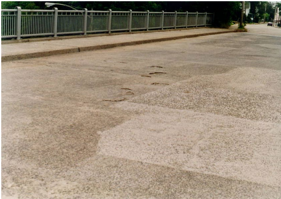
Figure 3.2.2-1 Top of Bare Concrete Deck with Patched, Spalled and Hollow Areas.
