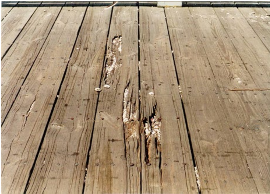
Figure 3.2.1-1 Deterioration of timber plank deck surface.
