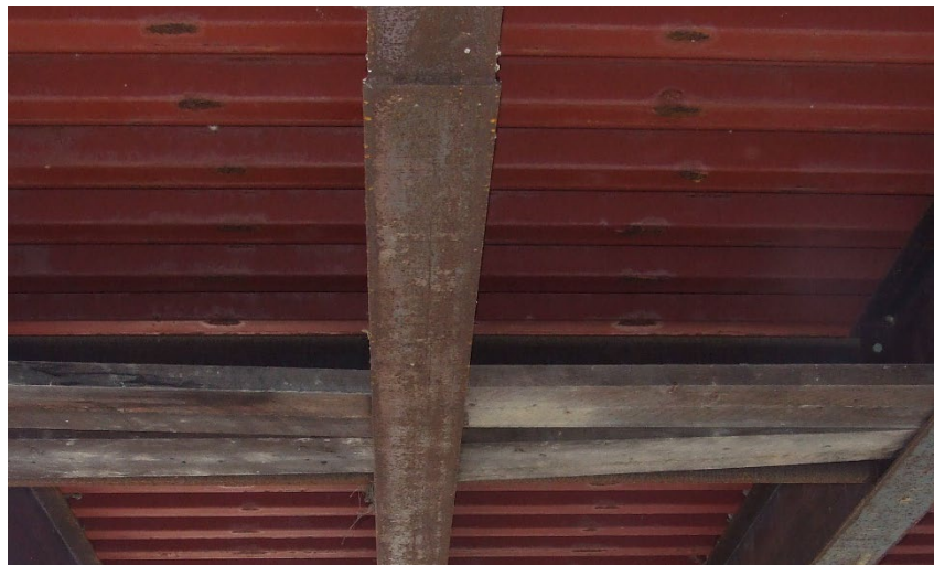
Figure 3.2.3-1 Underside of Corrugated Metal Deck
