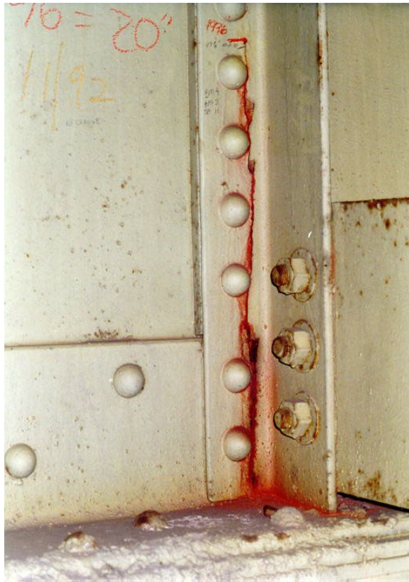
Figure 3.3.8-2 Fatigue Crack in a Diaphragm Connection Angle on a Girder.
