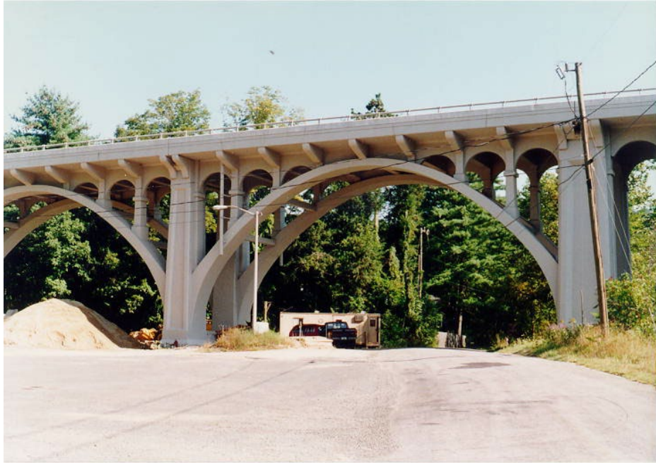
Figure 3.3.6-1 Open Spandrel Concrete Arch Bridge.
