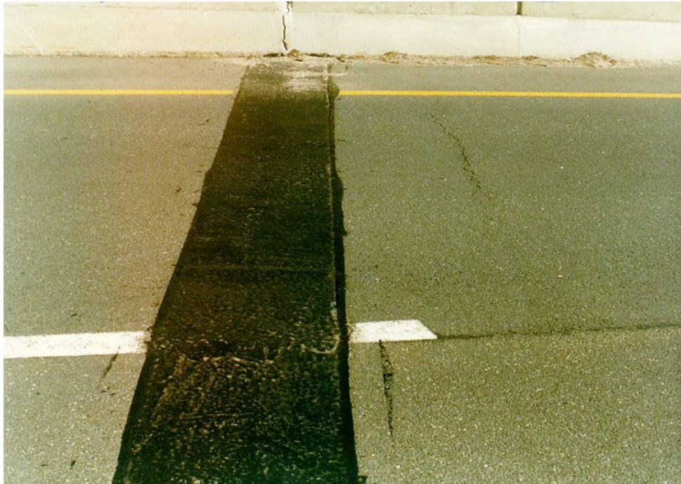
Figure 3.2.10-2 Asphaltic Plug Expansion Joint.
