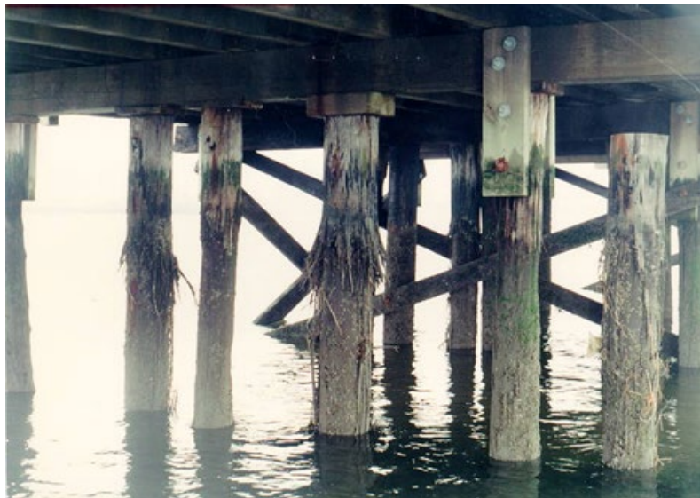
Figure 3.4.3-1 Timber Pile Bent exhibiting Freeze-Thaw Damage above the waterline. Also examples of shims, blocking and splices between the piles and pile cap
