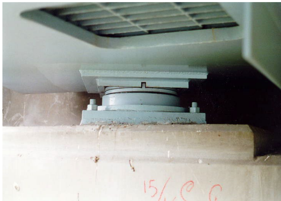
Figure 3.3.1-15 Center Guided Pot Bearing
