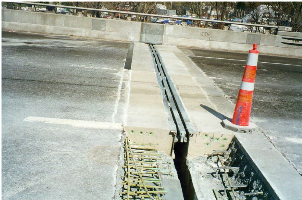
Figure 3.2.10-3 Modular Type Expansion Joint Replacement.
