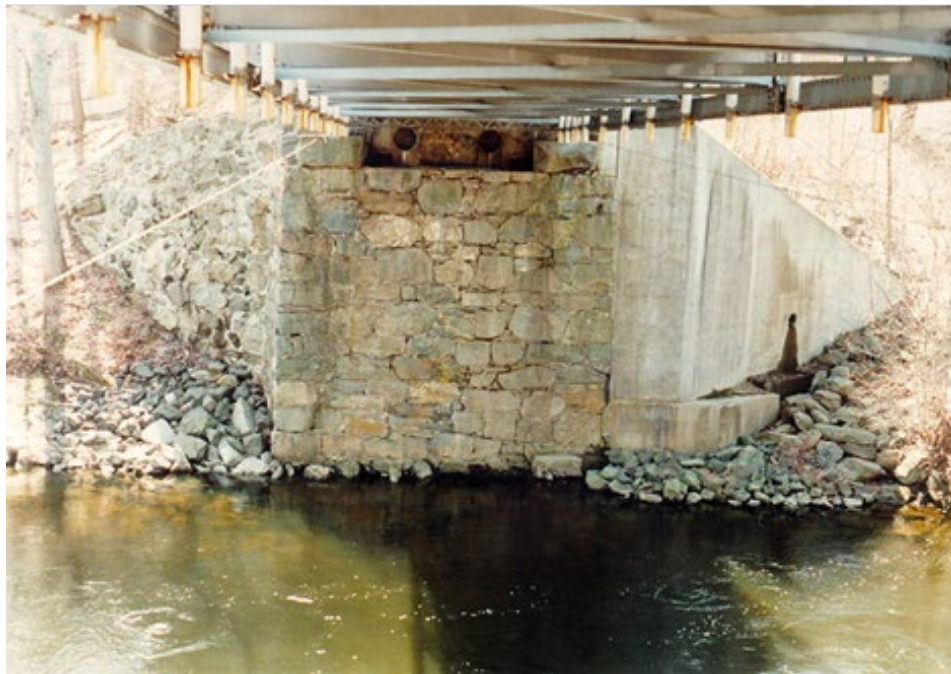
Figure 3.4.2-1 Tall Stone Masonry Bridge Abutment with Newer Concrete Wingwall Added.
