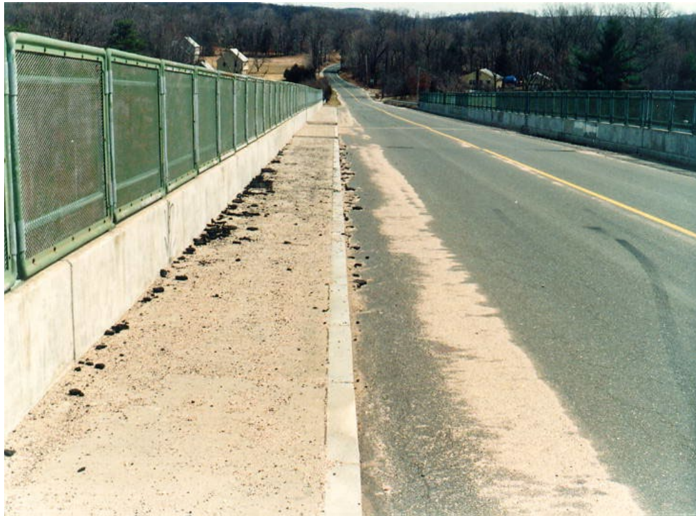
Figure 3.2.9-2 Pedestrian Fence atop Concrete Parapet.
