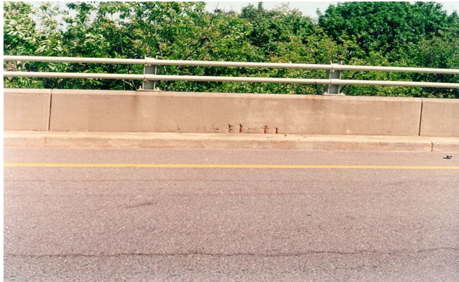
Figure 3.2.8-1 Concrete Parapet with Metal Pipe Railing. Note Spalling with Exposed Reinforcing Steel.
