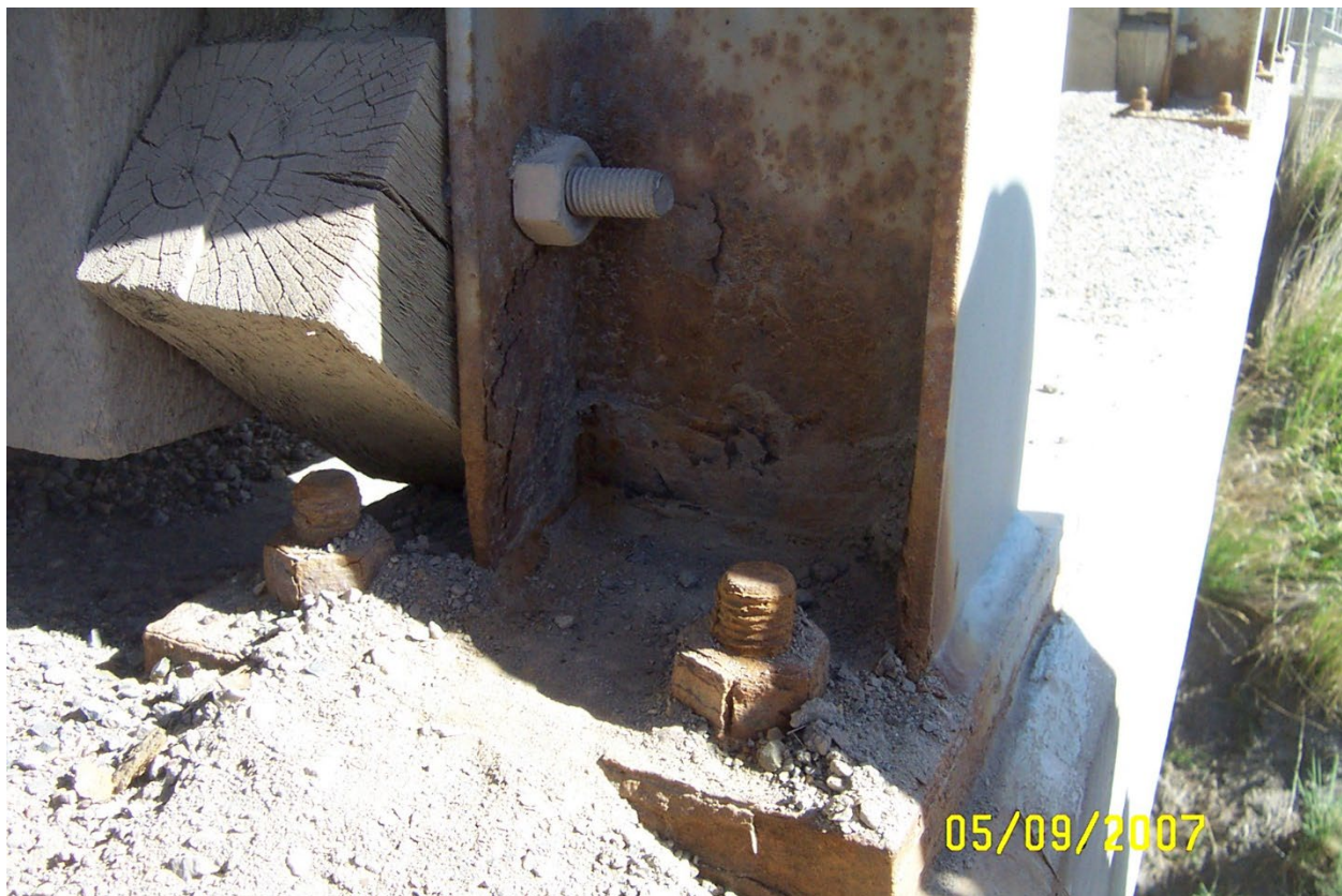
Figure 3.2.9-1 Steel Bridge Railing Post with Corrosion
