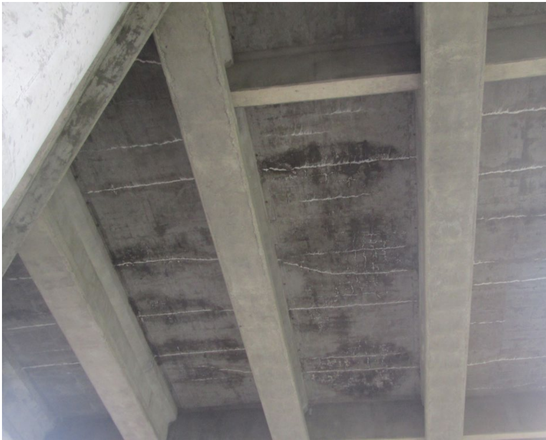
Figure 3. Typical Transverse Cracks Seen from Underneath
